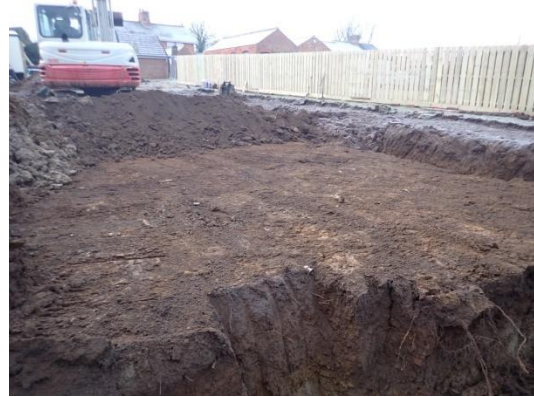
Plate 25: Internal ground reduction, from the north
