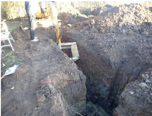
Plate 17: Excavation of the foundations, from the north-west
