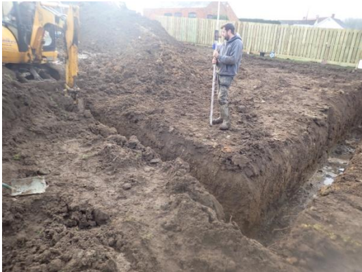
Plate 70: Excavation of the foundations, from the east
