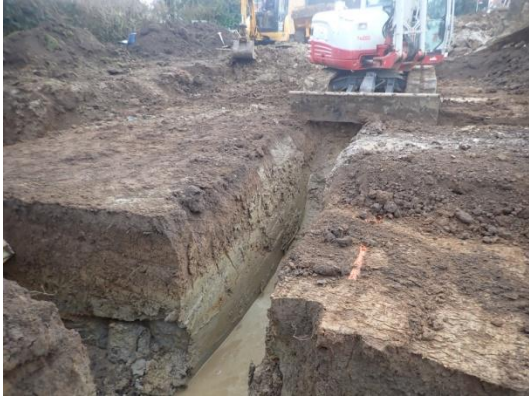
Plate 45: Excavation of the foundations, from the north
