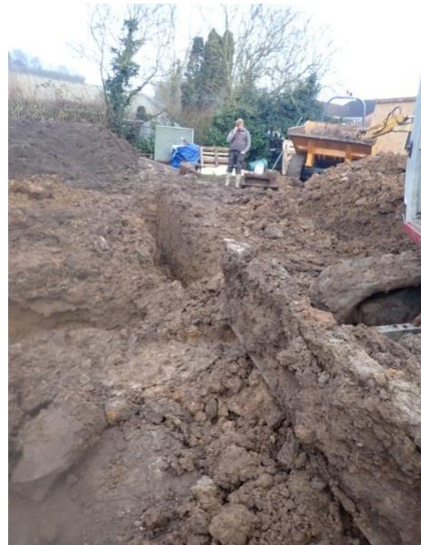
Plate 80: Excavation of the foundations, from the west
