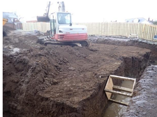
Plate 27: Internal ground reduction, from the east
