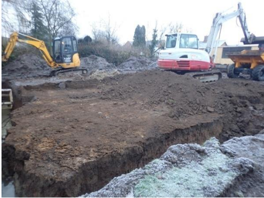
Plate 22: Internal ground reduction, from the west
