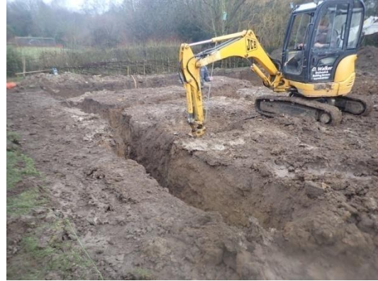
Plate 60: Excavation of the foundations, from the south
