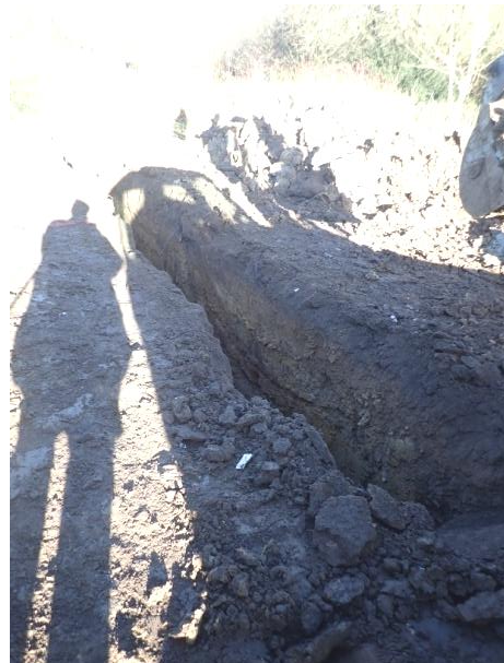
Plate 12: Excavation of the foundations, from the south
