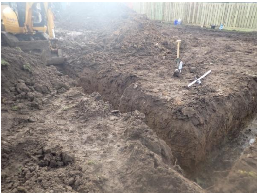
Plate 71: Excavation of the foundations, from the east
