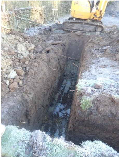
Plate 7: Excavation of the foundations, from the west
