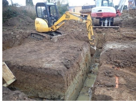
Plate 48: Excavation of the foundations, from the north
