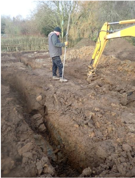
Plate 76: Excavation of the foundations, from the south
