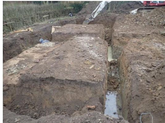
Plate 55: Excavation of the foundations, from the west
