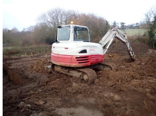
Plate 79: Excavation of the foundations, from the south-west
