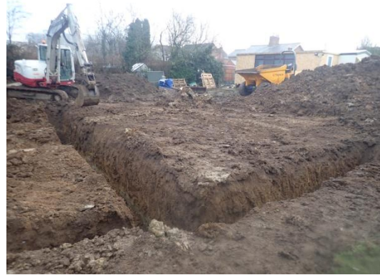
Plate 66: Excavation of the foundations, from the west
