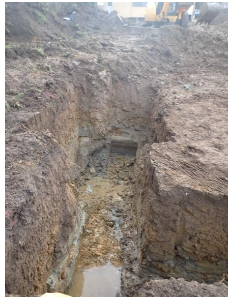
Plate 44: Excavation of the foundations, from the north
