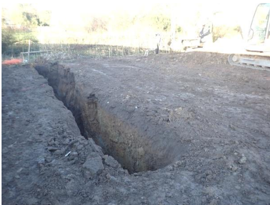
Plate 18: Excavation of the foundations, from the south
