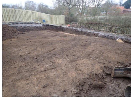
Plate 37: Internal ground reduction, from the east
