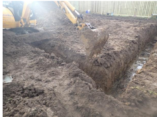
Plate 68: Excavation of the foundations, from the east
