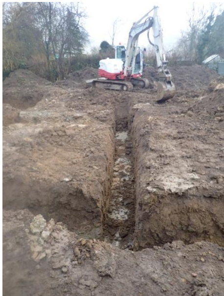
Plate 65: Excavation of the foundations, from the west
