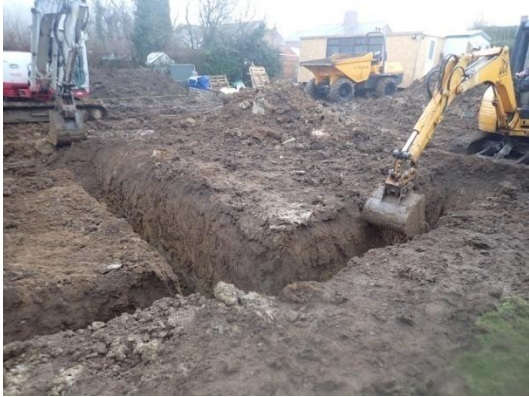
Plate 63: Excavation of the foundations, from the west
