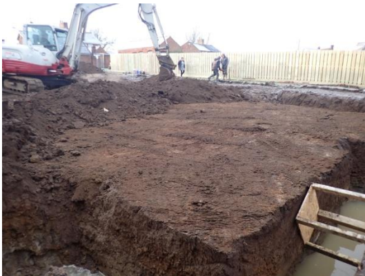
Plate 30: Internal ground reduction, from the east
