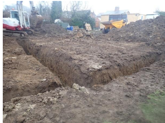
Plate 67: Excavation of the foundations, from the west
