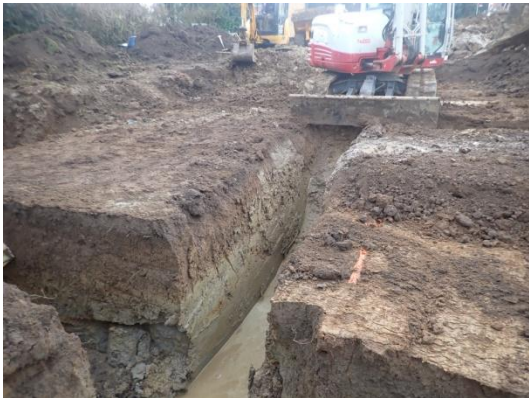
Plate 46: Excavation of the foundations, from the north
