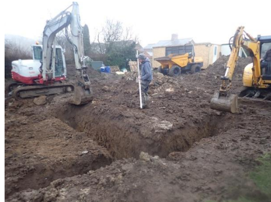
Plate 61: Excavation of the foundations, from the west
