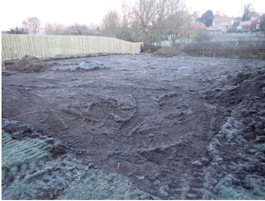
Plate 1: Pre-groundworks, from the south-east
