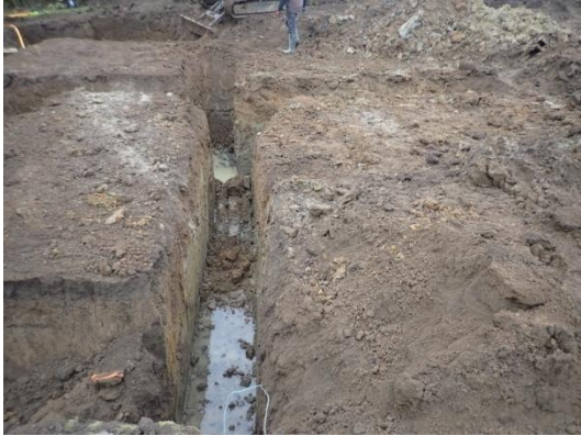
Plate 51: Excavation of the foundations, from the west
