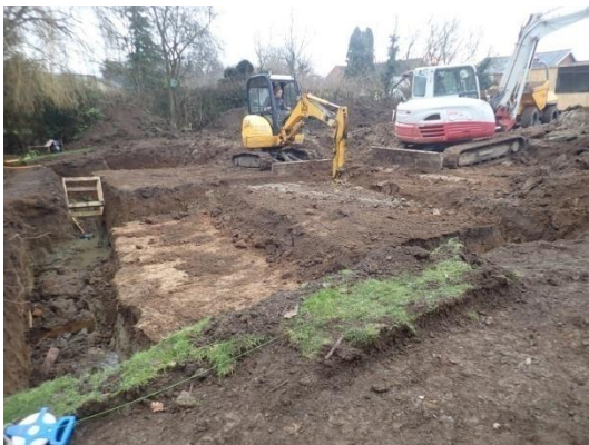
Plate 47: Excavation of the foundations, from the west
