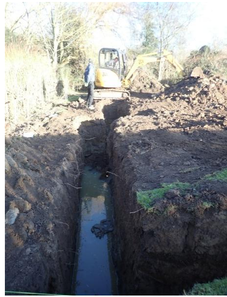
Plate 15: Excavation of the foundations, from the west
