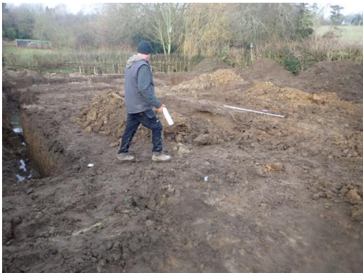
Plate 77: Excavation of the foundations, from the south
