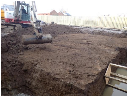
Plate 29: Internal ground reduction, from the east
