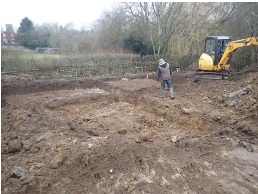
Plate 53: Excavation of the foundations, from the south
