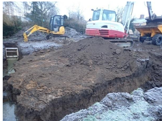
Plate 21: Internal ground reduction, from the west
