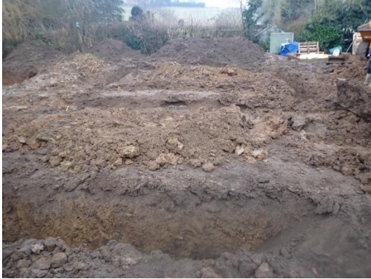
Plate 81: Excavation of the foundations, from the west
