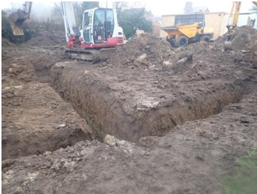
Plate 64: Excavation of the foundations, from the west
