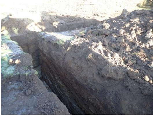
Plate 11: Excavation of the foundations, from the south
