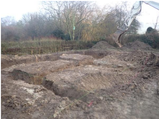
Plate 58: Excavation of the foundations, from the south-west
