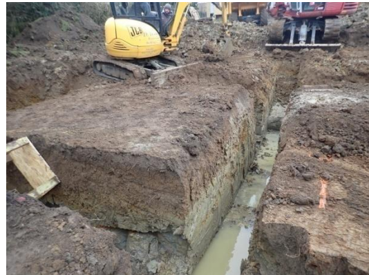
Plate 49: Excavation of the foundations, from the north
