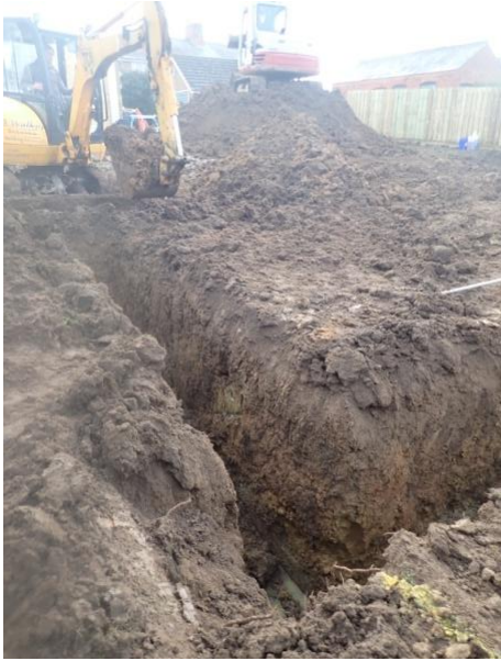
Plate 69: Excavation of the foundations, from the north
