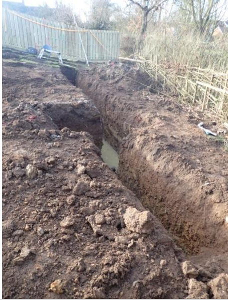
Plate 16: Excavation of the foundations, from the east
