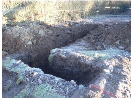
Plate 9: Excavation of the foundations, from the west
