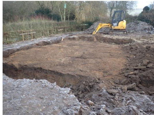
Plate 26: Internal ground reduction, from the west
