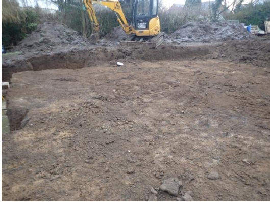
Plate 34: Internal ground reduction, from the west
