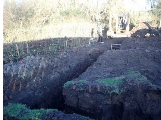
Plate 19: Excavation of the foundations, from the west
