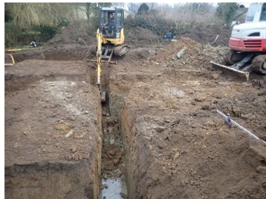
Plate 50: Excavation of the foundations, from the west
