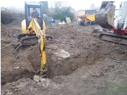
Plate 59: Excavation of the foundations, from the west
