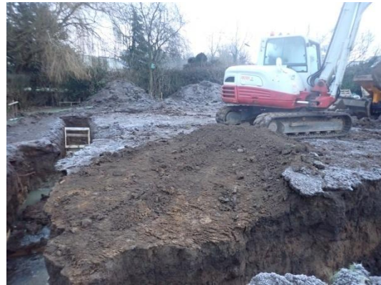
Plate 20: Internal ground reduction, from the west
