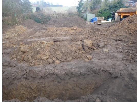
Plate 78: Excavation of the foundations, from the west
