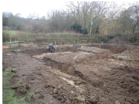
Plate 56: Excavation of the foundations, from the south-west
