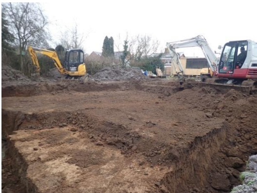
Plate 36: Internal ground reduction, from the west
