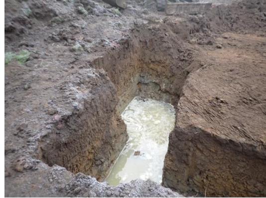
Plate 31: Excavation of the foundations, from the north
