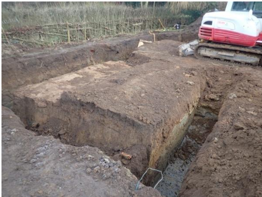
Plate 41: Excavation of the foundations, from the west
