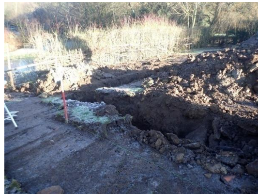
Plate 10: Excavation of the foundations, from the south-west
