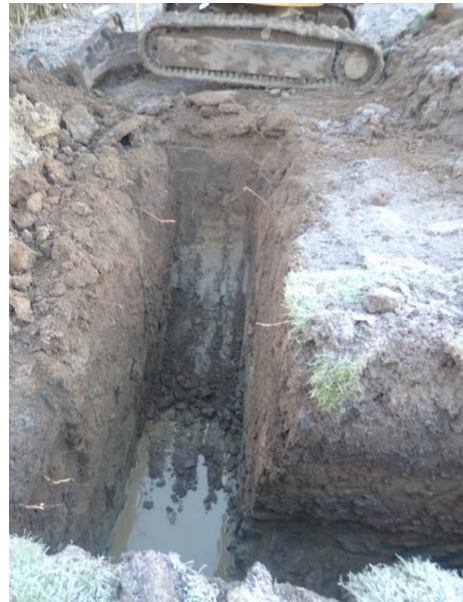
Plate 5: Excavation of the foundations, from the west
