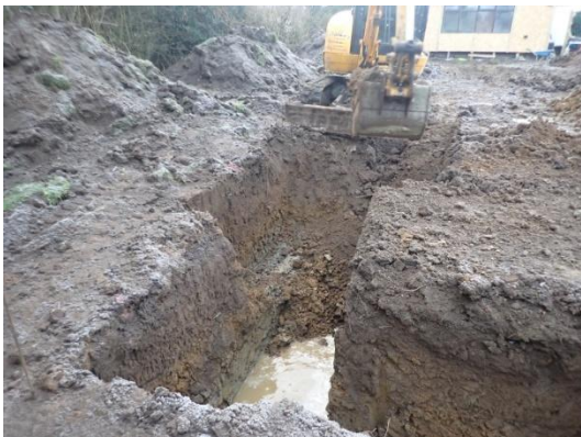
Plate 24: Excavation of the foundations, from the north
