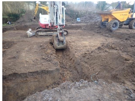
Plate 39: Excavation of the foundations, from the west
