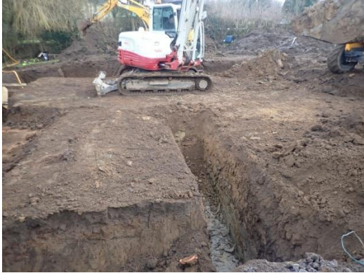
Plate 40: Excavation of the foundations, from the west
