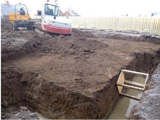
Plate 28: Internal ground reduction, from the east
