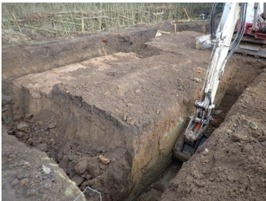
Plate 42: Excavation of the foundations, from the west
