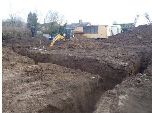
Plate 72: Excavation of the foundations, from the north-west
