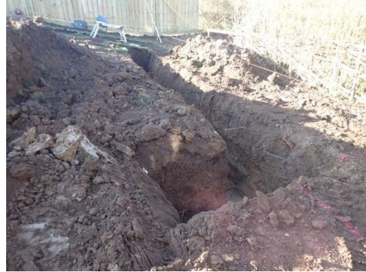
Plate 14: Excavation of the foundations, from the east
