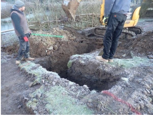
Plate 6: Excavation of the foundations, from the south-west
