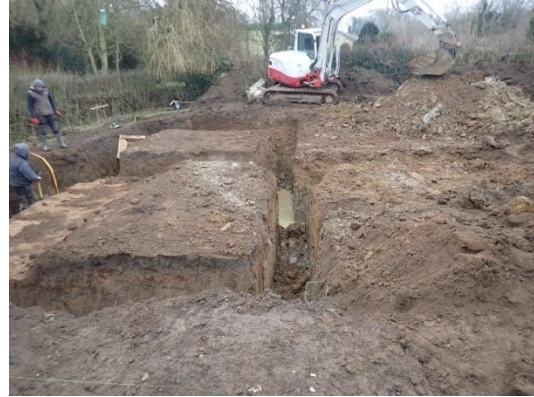
Plate 54: Excavation of the foundations, from the west
