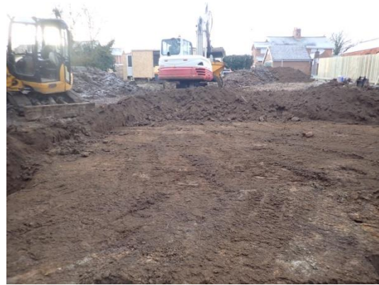
Plate 33: Internal ground reduction, from the north
