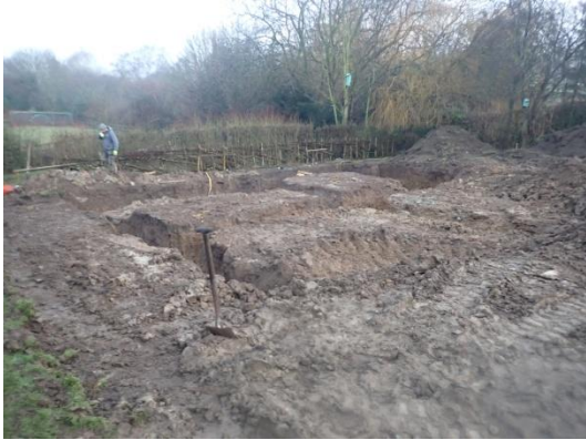
Plate 57: Excavation of the foundations, from the south-west
