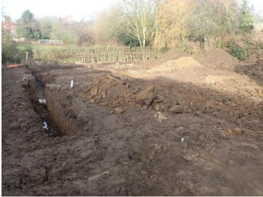
Plate 75: Excavation of the foundations, from the south
