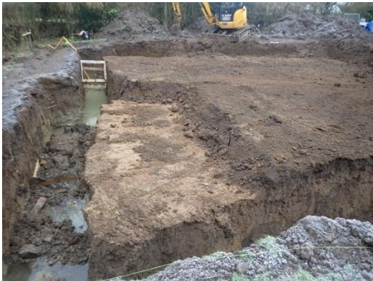
Plate 35: Internal ground reduction, from the west
