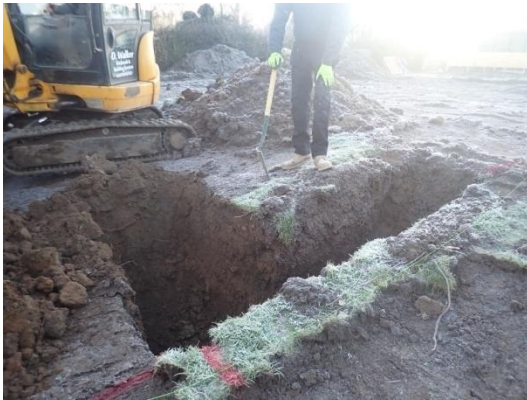
Plate 3: Excavation of the foundations, from the west
