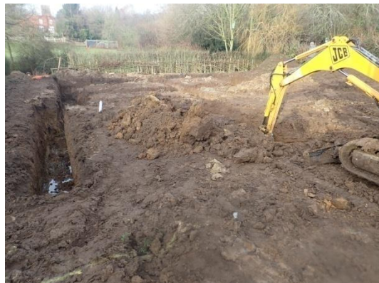
Plate 74: Excavation of the foundations, from the south
