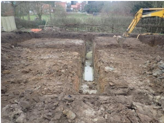
Plate 52: Excavation of the foundations, from the south
