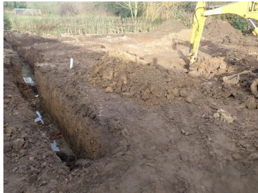
Plate 73: Excavation of the foundations, from the south
