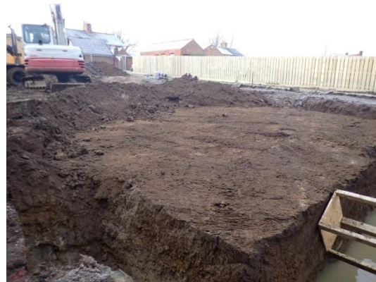
Plate 32: Internal ground reduction, from the east
