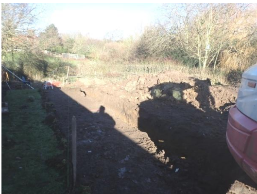
Plate 13: Excavation of the foundations, from the south
