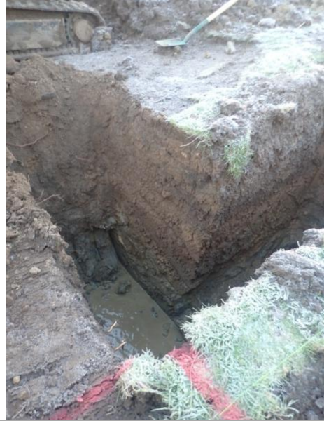
Plate 4: Excavation of the foundations, from the west
