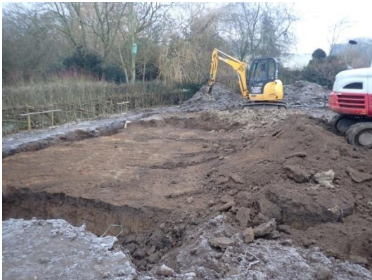
Plate 23: Internal ground reduction, from the west
