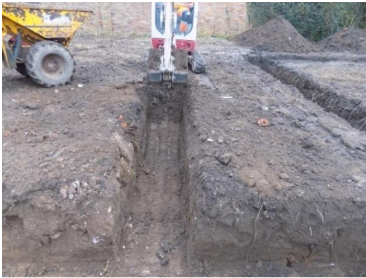
Plate 25: Excavation of the foundations, from the north
