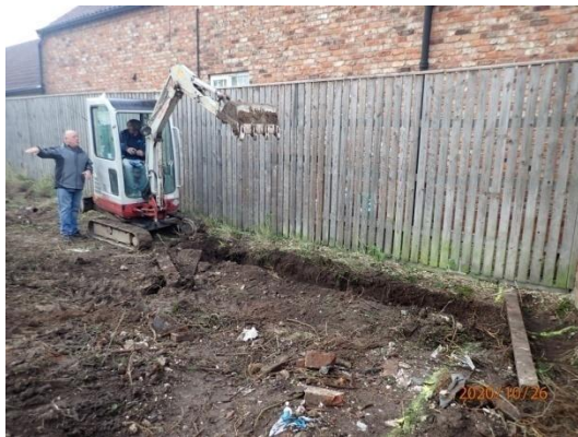
Plate 2: Excavation of the foundations, from the south-west
