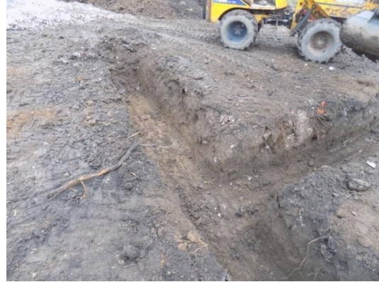
Plate 26: Excavation of the foundations, from the north
