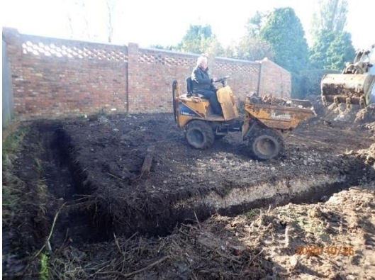
Plate 7: Excavation of the foundations, from the north
