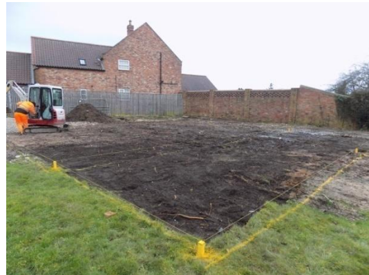
Plate 17: Pre-groundworks, from the north-west
