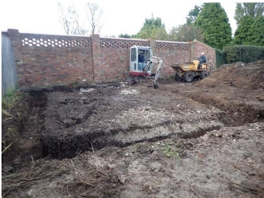
Plate 15: Excavation of the foundations, from the north
