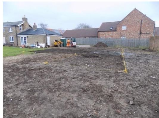
Plate 18: Pre-groundworks, from the west
