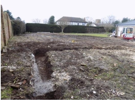
Plate 19: Excavation of the foundations, from the east
