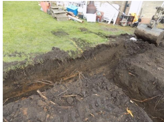
Plate 23: Excavation of the foundations, from the south-east
