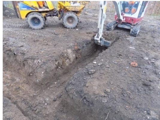
Plate 27: Excavation of the foundations, from the north
