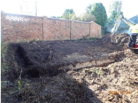
Plate 8: Excavation of the foundations, from the north
