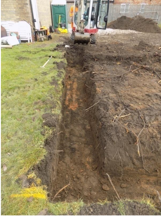
Plate 24: Excavation of the foundations, from the west
