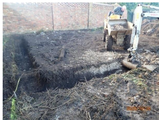
Plate 6: Excavation of the foundations, from the north
