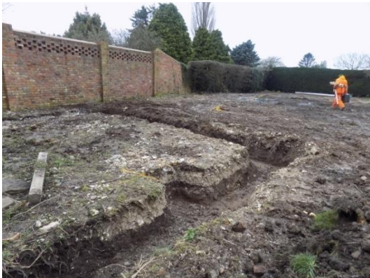
Plate 20: Excavation of the foundations, from the east
