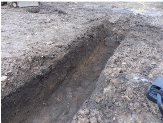
Plate 21: Excavation of the foundations, from the east
