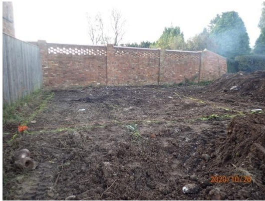
Plate 1: Pre-groundworks, from the north
