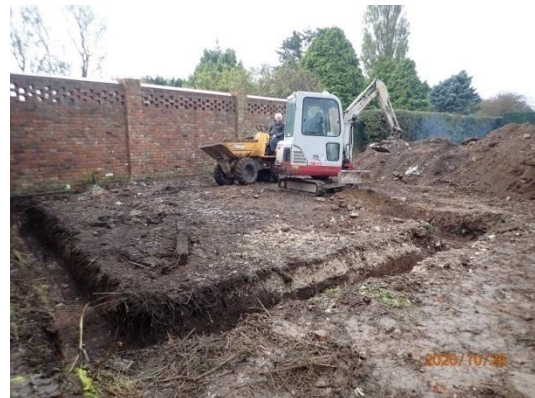
Plate 12: Excavation of the foundations, from the north
