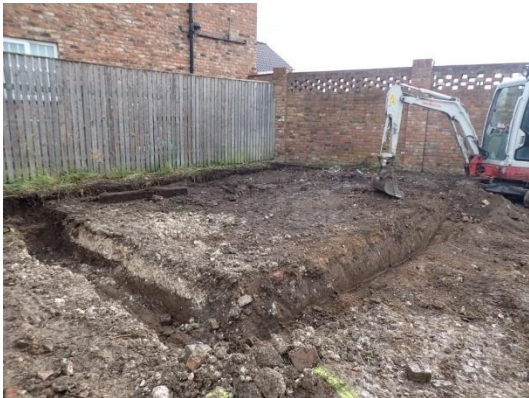
Plate 14: Excavation of the foundations, from the north-west
