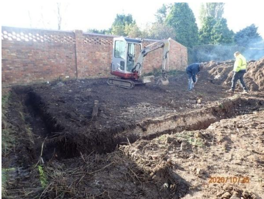
Plate 9: Excavation of the foundations, from the north
