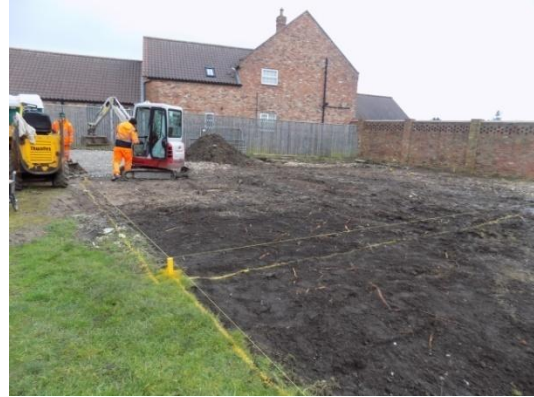
Plate 16: Pre-groundworks, from the west
