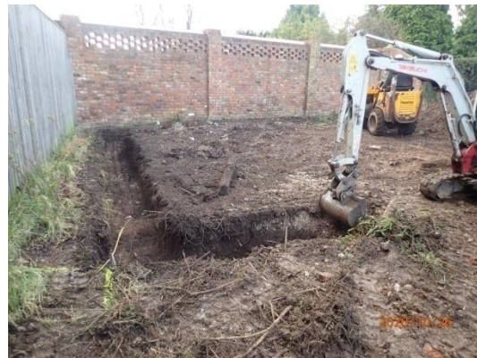
Plate 5: Excavation of the foundations, from the north
