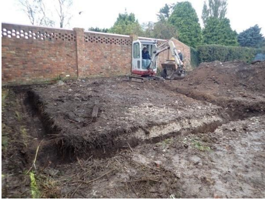
Plate 13: Excavation of the foundations, from the north
