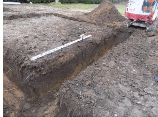
Plate 22: Excavation of the foundations, from the south-east
