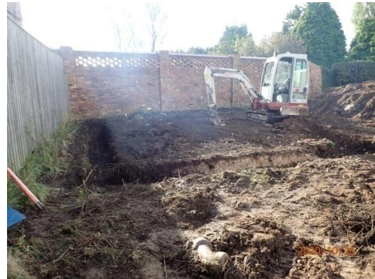
Plate 11: Excavation of the foundations, from the north
