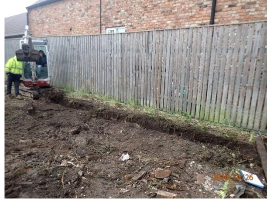
Plate 4: Excavation of the foundations, from the south-west
