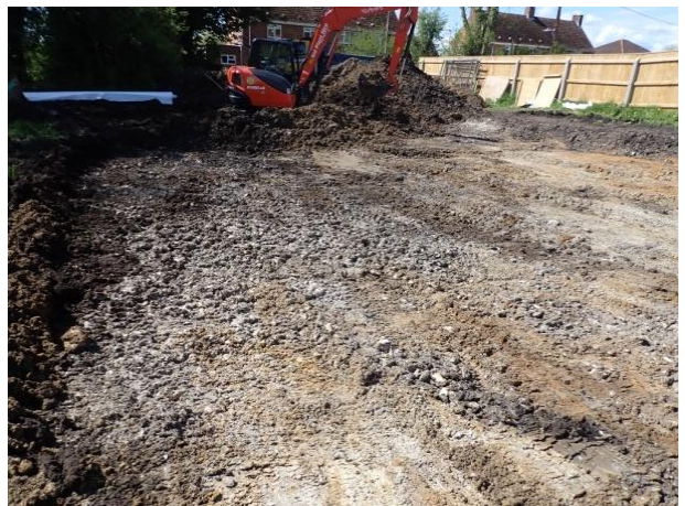
Plate 42: Site ground reduction, from the north
