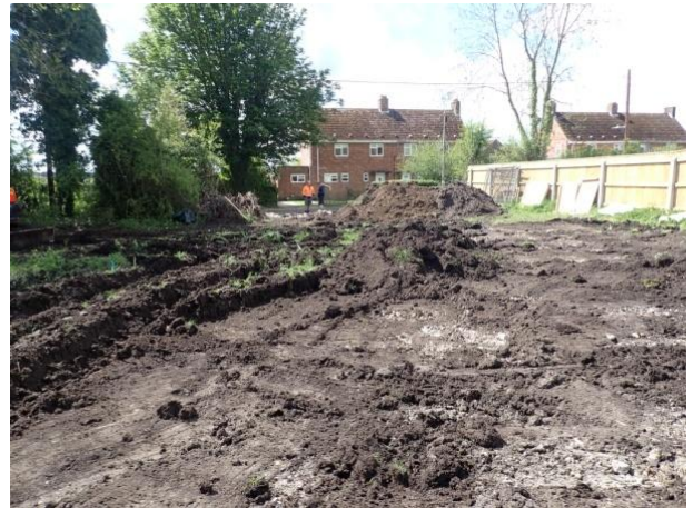
Plate 17: Site ground reduction, from the north
