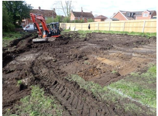
Plate 11: Site ground reduction, from the north
