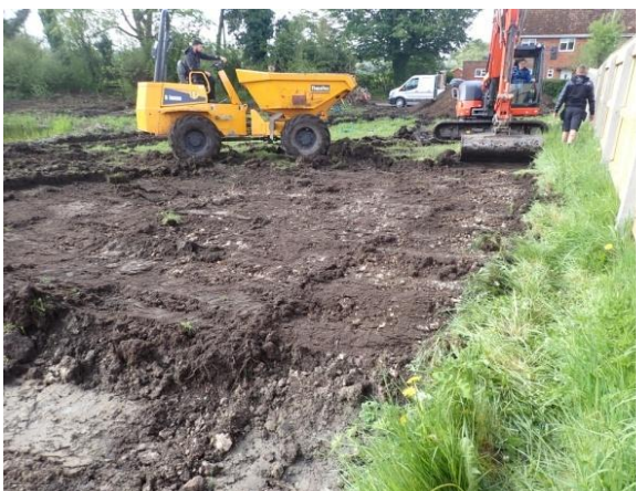
Plate 9: Site ground reduction, from the north
