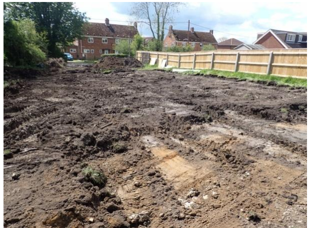
Plate 24: Site ground reduction, from the north
