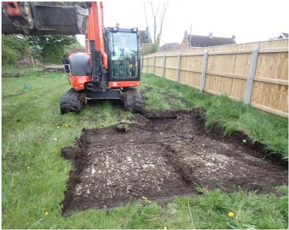
Plate 1: Site ground reduction, from the north
