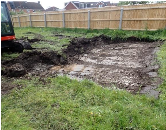
Plate 3: Site ground reduction, from the east
