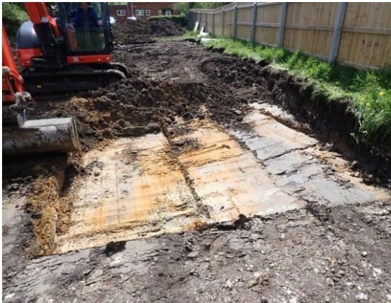
Plate 26: Site ground reduction, from the north
