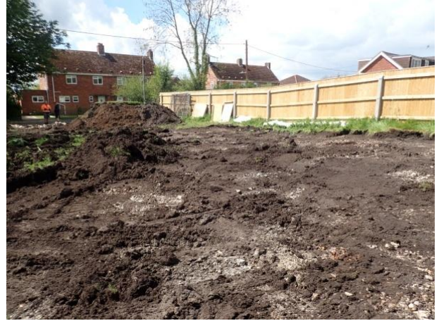
Plate 16: Site ground reduction, from the north
