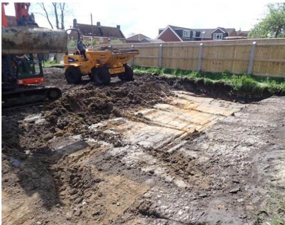
Plate 27: Site ground reduction, from the east
