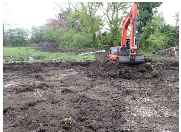
Plate 18: Site ground reduction, from the north-west
