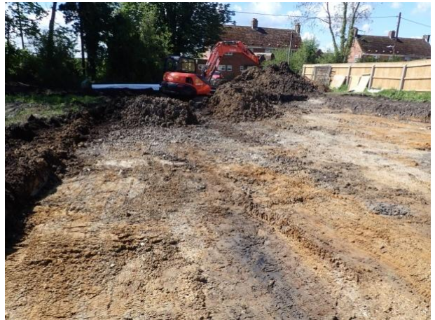
Plate 41: Site ground reduction, from the north
