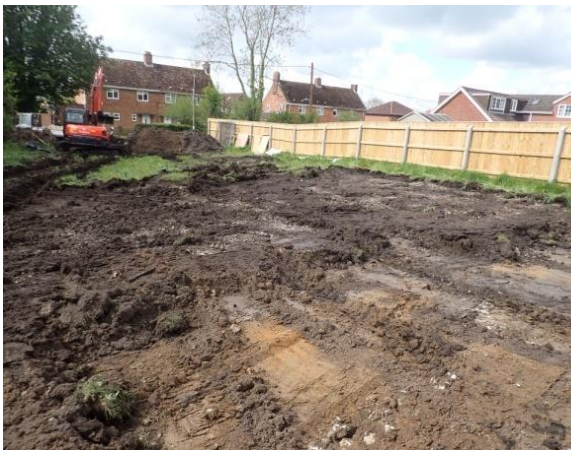
Plate 15: Site ground reduction, from the north-east
