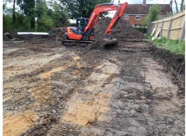
Plate 52: Site ground reduction, from the north
