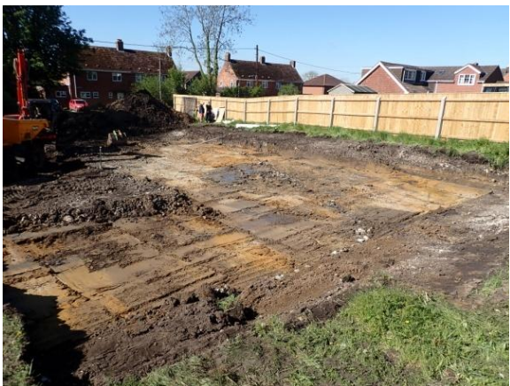
Plate 39: Site ground reduction, from the north-east
