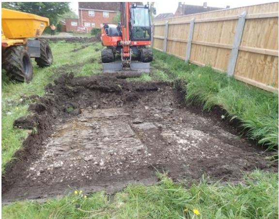
Plate 2: Site ground reduction, from the north
