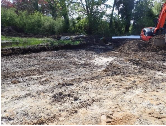
Plate 43: Site ground reduction, from the north
