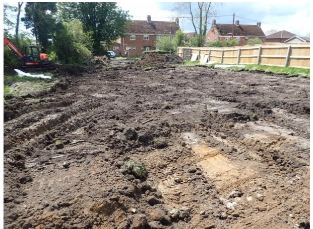
Plate 23: Site ground reduction, from the north
