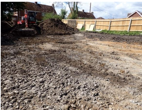
Plate 45: Site ground reduction, from the north-east
