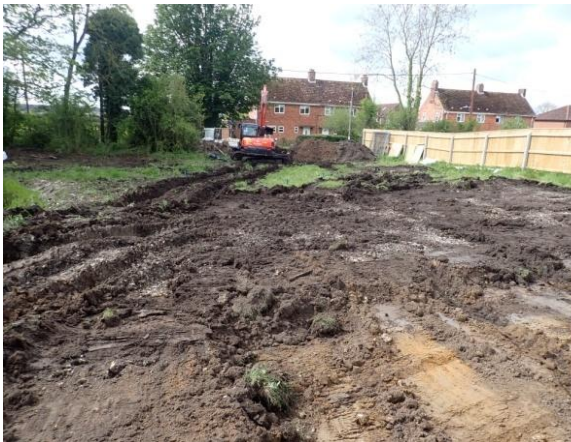
Plate 14: Site ground reduction, from the north
