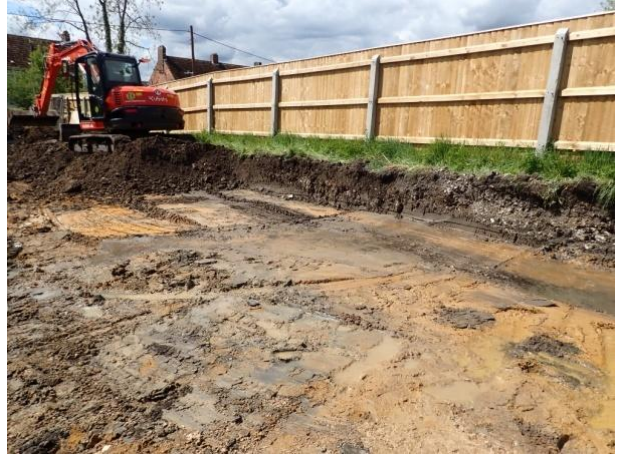
Plate 46: Site ground reduction, from the north-east
