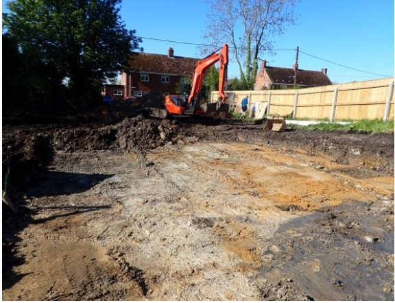
Plate 37: Site ground reduction, from the north
