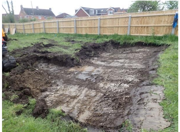
Plate 4: Site ground reduction, from the east
