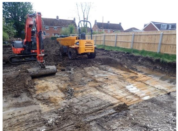
Plate 30: Site ground reduction, from the north
