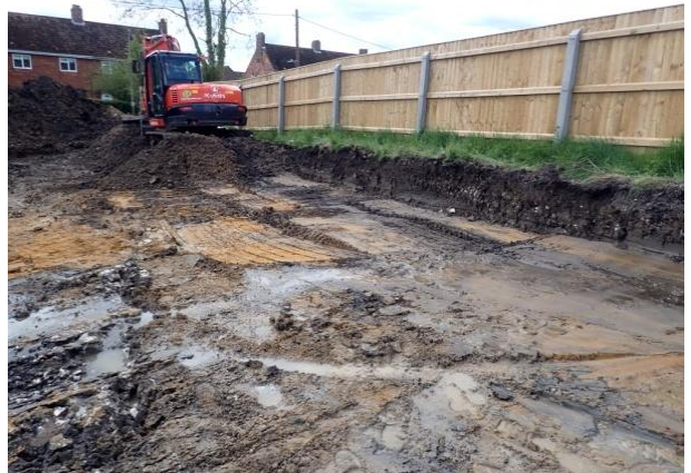
Plate 47: Site ground reduction, from the north
