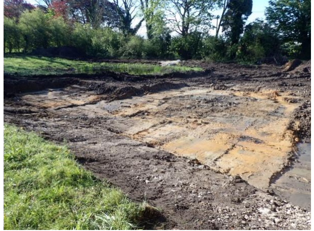
Plate 34: Site ground reduction, from the north-west
