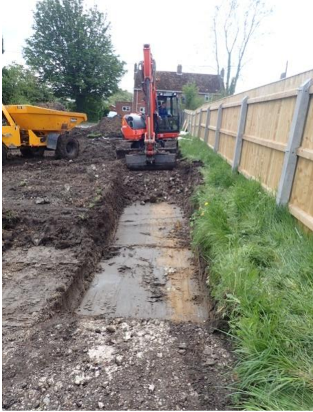
Plate 25: Site ground reduction, from the north
