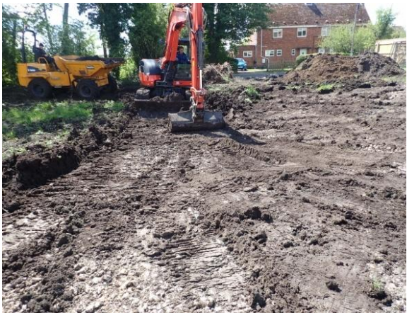
Plate 20: Site ground reduction, from the north
