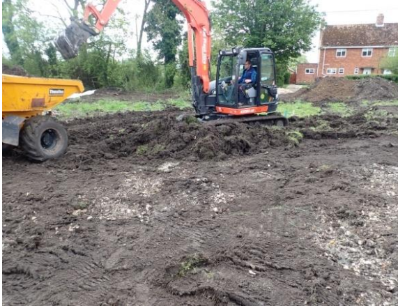
Plate 13: Site ground reduction, from the north
