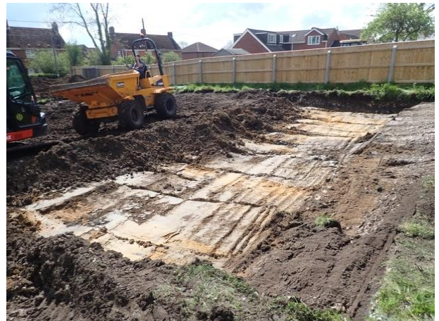
Plate 29: Site ground reduction, from the east
