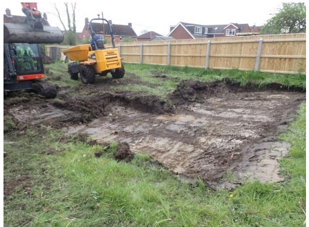
Plate 5: Site ground reduction, from the east
