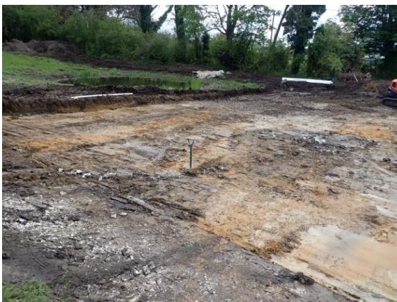
Plate 51: Site ground reduction, from the north-west
