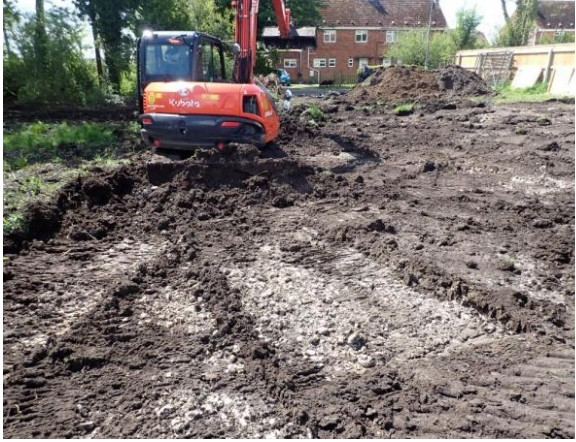
Plate 19: Site ground reduction, from the north
