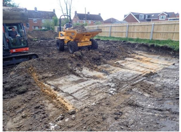
Plate 28: Site ground reduction, from the north-east
