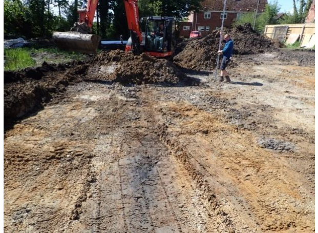
Plate 40: Site ground reduction, from the north
