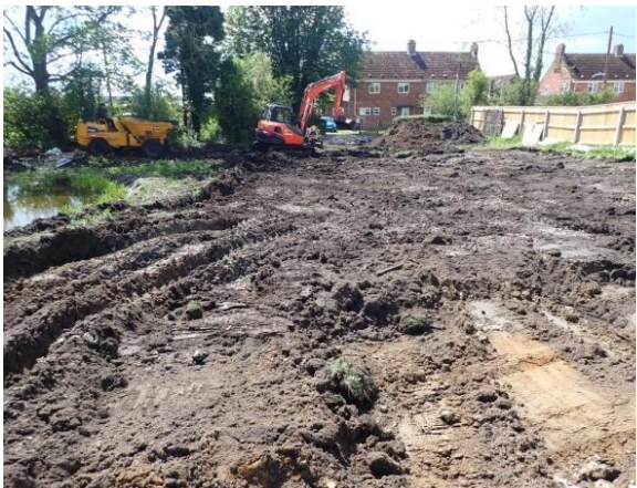
Plate 21: Site ground reduction, from the north
