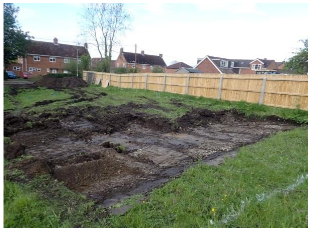
Plate 6: Site ground reduction, from the north-east
