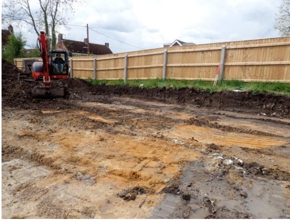
Plate 49: Site ground reduction, from the north-east
