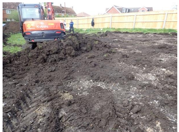
Plate 12: Site ground reduction, from the north
