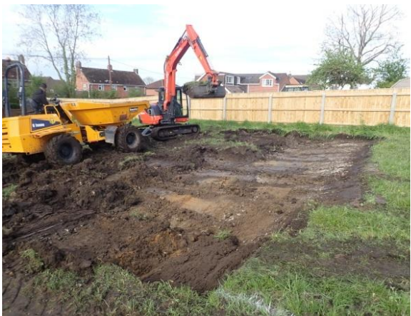
Plate 8: Site ground reduction, from the east
