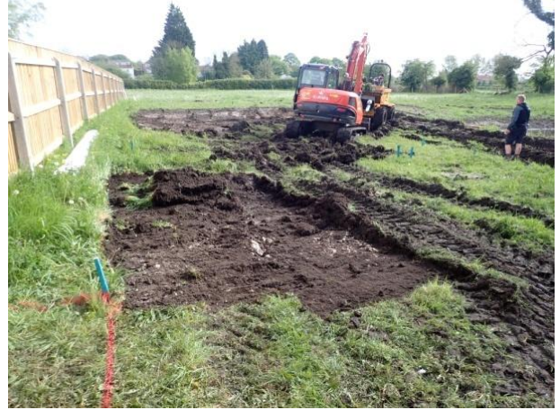
Plate 10: Site ground reduction, from the south
