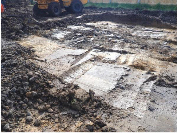
Plate 31: Site ground reduction, from the east
