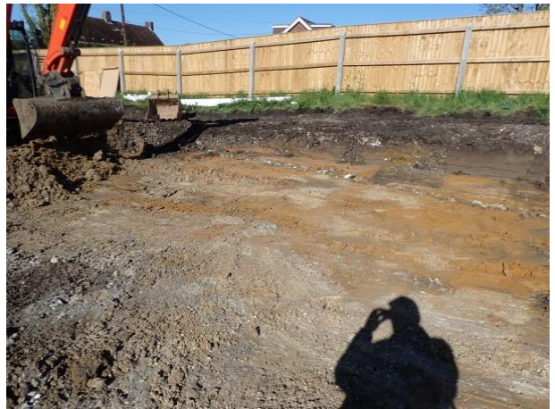
Plate 36: Site ground reduction, from the east
