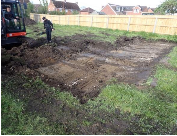
Plate 7: Site ground reduction, from the north-east
