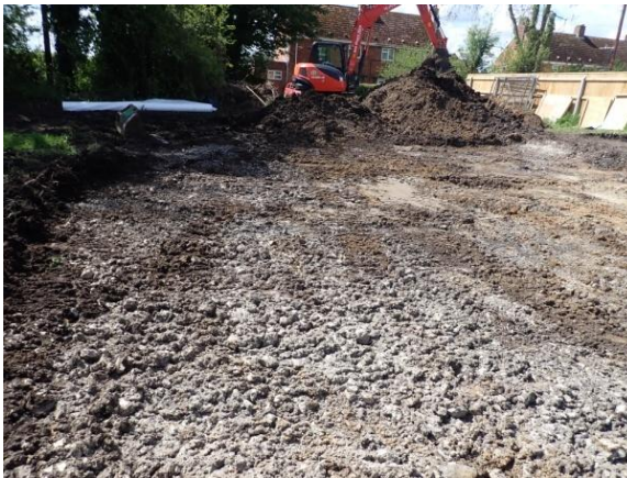
Plate 44: Site ground reduction, from the north
