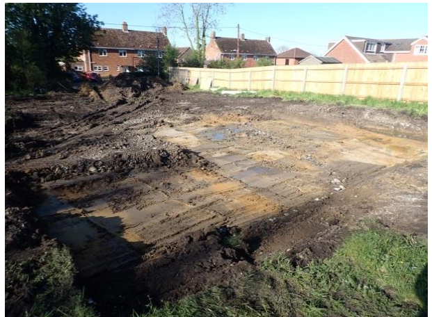
Plate 35: Site ground reduction, from the north-east
