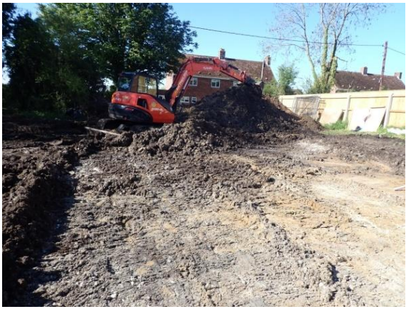
Plate 38: Site ground reduction, from the north
