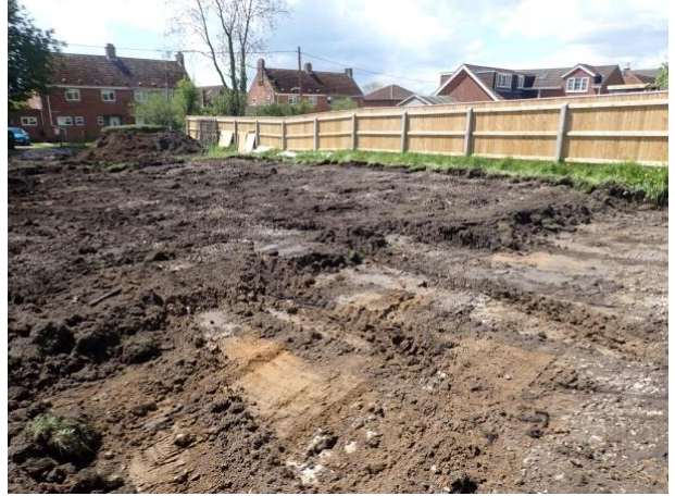
Plate 22: Site ground reduction, from the north-east
