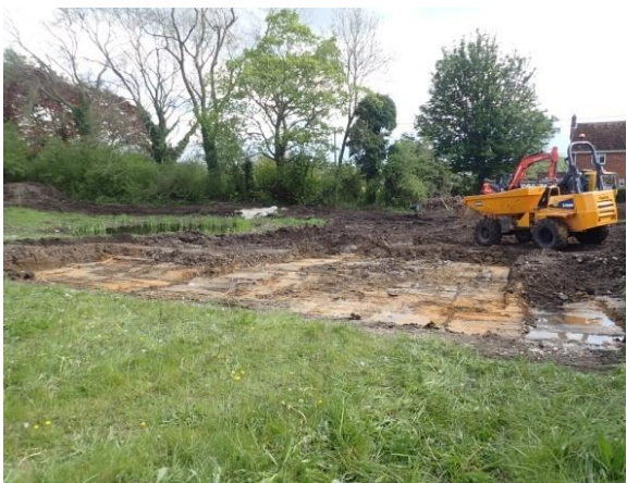
Plate 33: Site ground reduction, from the north
