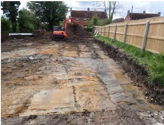
Plate 50: Site ground reduction, from the north
