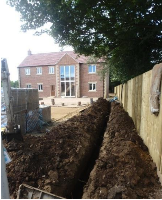
Plate 10: Excavation of the first service trench, from the north
