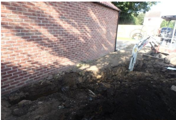
Plate 19: Excavation of the second service trench, from the east
