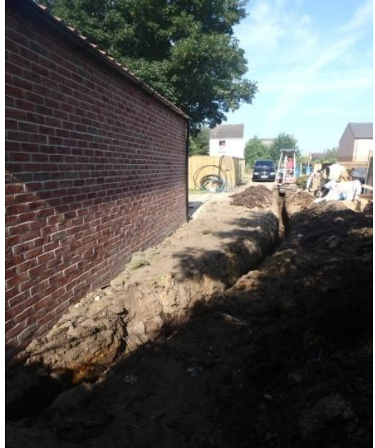
Plate 30: Excavation of the second service trench, from the east
