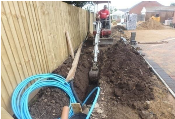
Plate 2: Excavation of the first service trench, from the south
