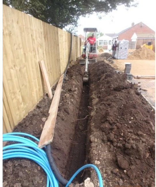
Plate 4: Excavation of the first service trench, from the south
