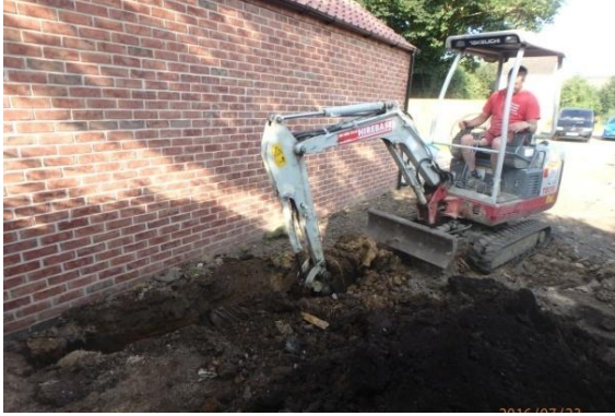
Plate 18: Excavation of the second service trench, from the east
