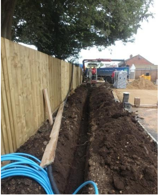
Plate 6: Excavation of the first service trench, from the south
