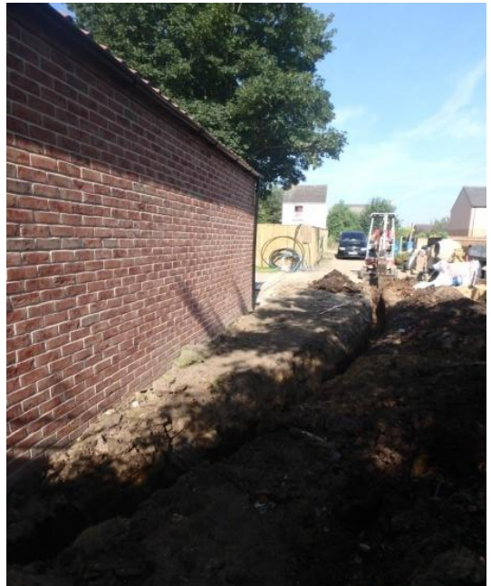
Plate 27: Excavation of the second service trench, from the east
