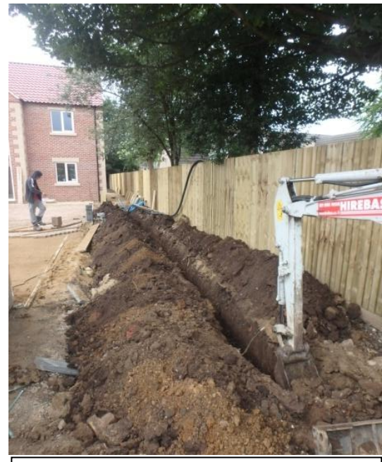
Plate 9: Excavation of the first service trench, from the north
