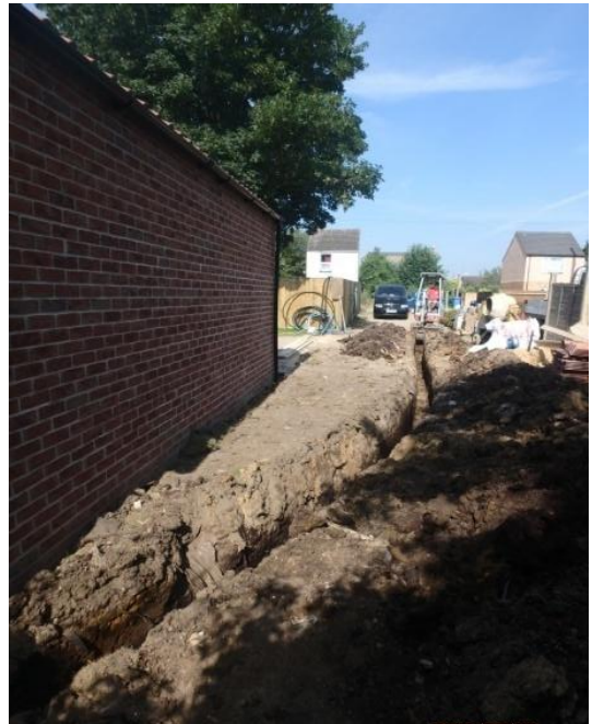
Plate 31: Excavation of the second service trench, from the east
