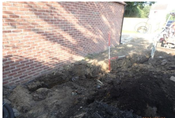
Plate 22: Excavation of the second service trench, from the east
