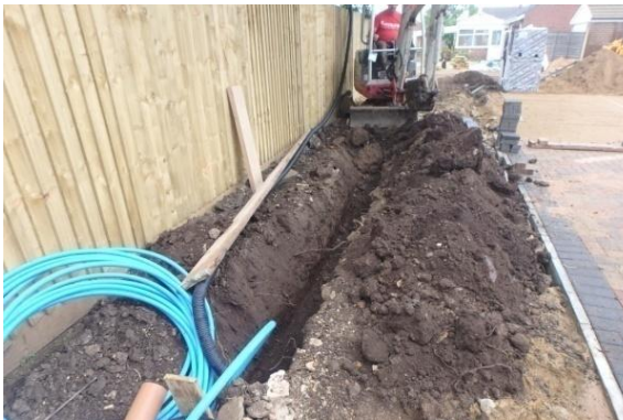
Plate 3: Excavation of the first service trench, from the south
