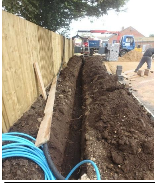
Plate 8: Excavation of the first service trench, from the south
