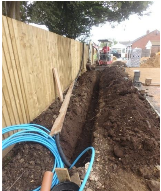
Plate 5: Excavation of the first service trench, from the south
