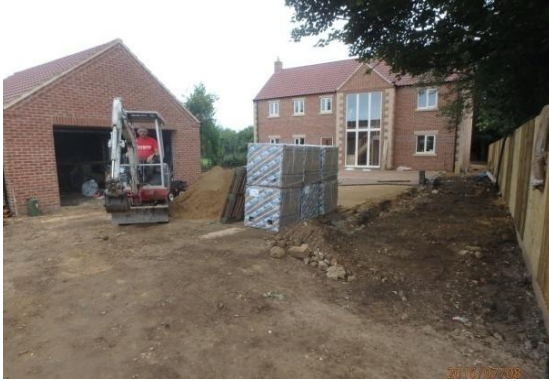
Plate 1: Pre-excitation, first service trench, from the south
