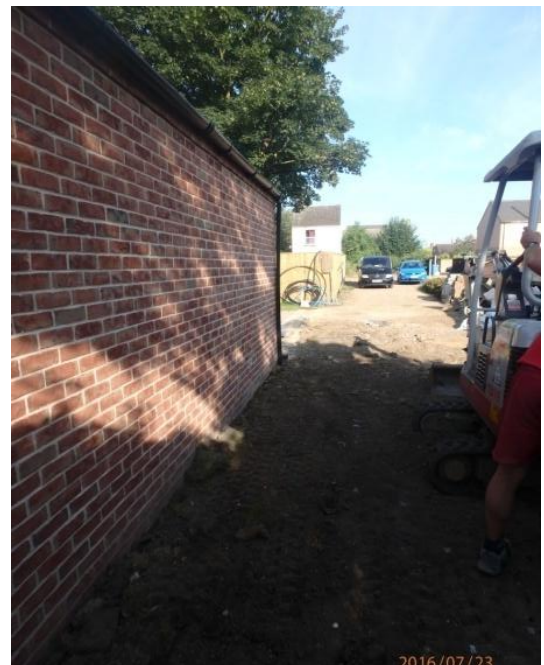
Plate 17: Pre-excavation, second service trench, from the east
