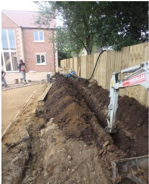
Plate 7: Excavation of the first service trench, from the north
