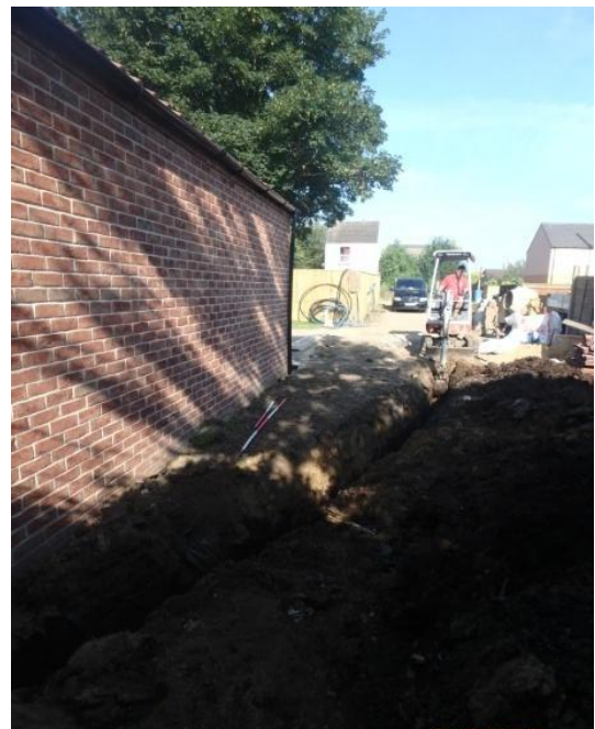
Plate 23: Excavation of the second service trench, from the east
