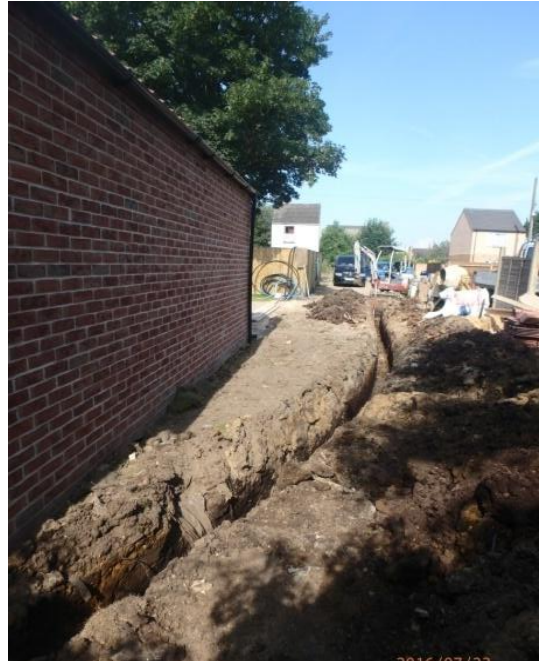
Plate 34: Excavation of the second service trench, from the east
