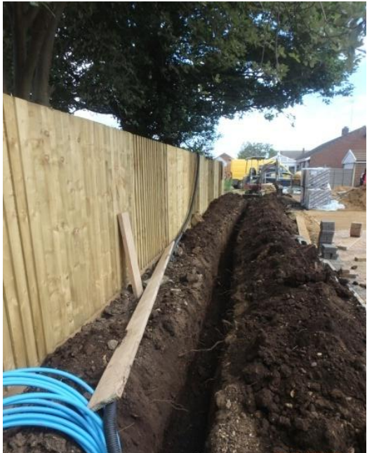
Plate 11: Excavation of the first service trench, from the south
