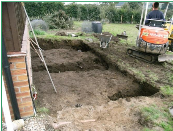
Plate 6: Completed excavation of new build footprint showing foundation trenches and posthole to north-east, from the east
