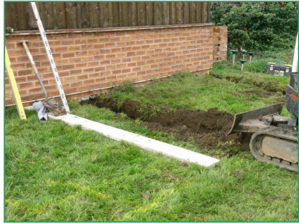
Plate 2: Work in progress, excavated foundation trenches, from the east
