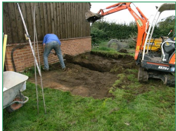
Plate 4: Work in progress, removal of turf within build footprint, from the east
