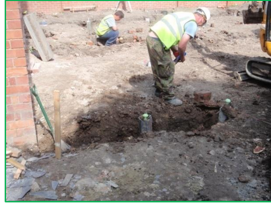
Plate 30: Work in progress, excavation of ring beams, from the south
