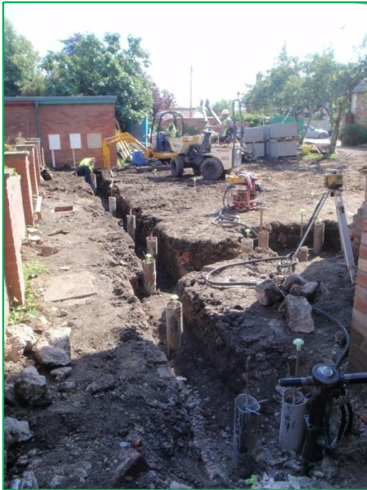
Plate 15: Ring beam excavations, from the west
