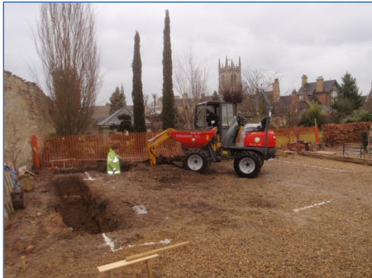
Plate 6: Work in progress, from the south
