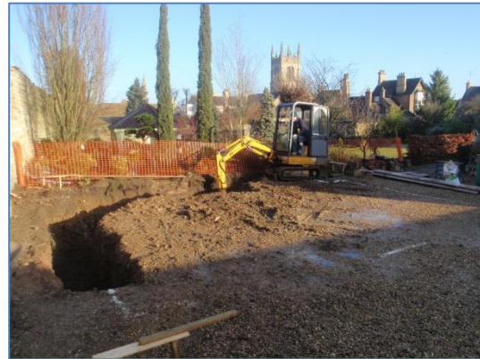
Plate 12: Work in progress, from the south
