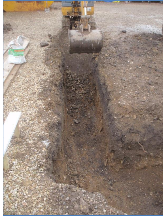
Plate 16: Work in progress, from the north
