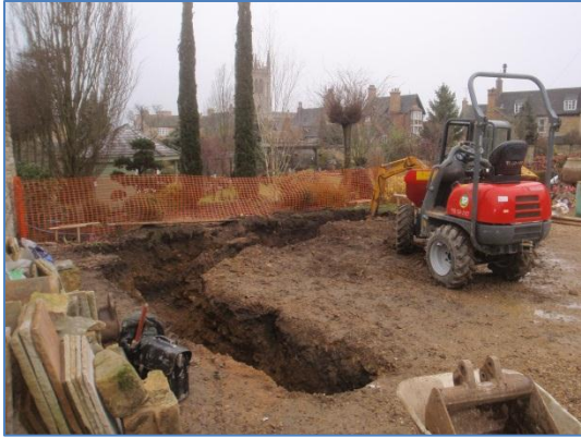
Plate 14: Work in progress, from the south
