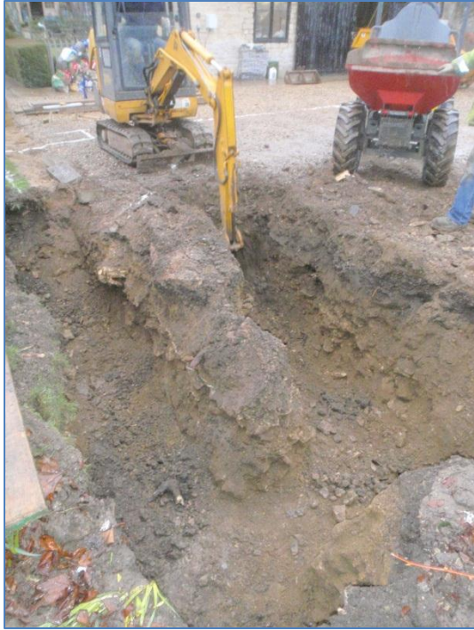
Plate 9: Work in progress, from the west
