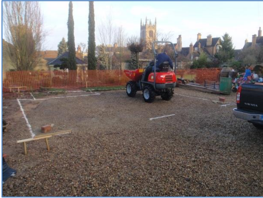
Plate 1: Pre-groundworks, from the south
