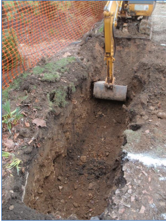
Plate 5: Work in progress, from the west
