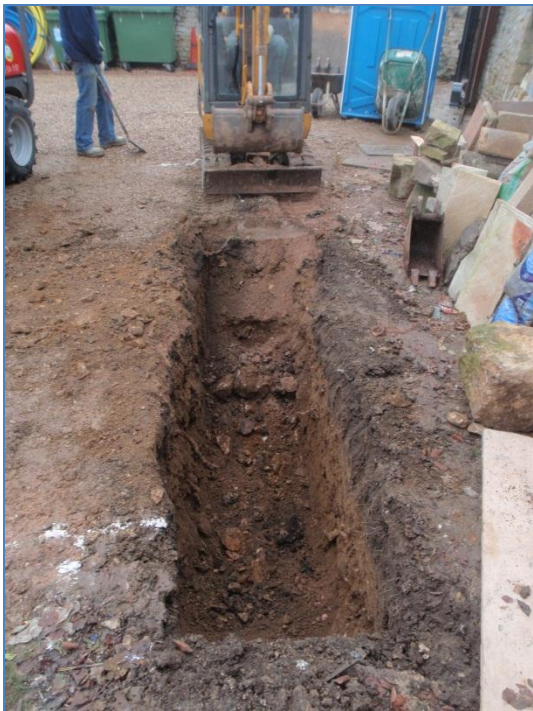
Plate 2: Work in progress, from the north
