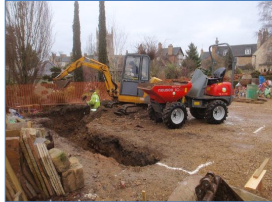
Plate 7: Work in progress, from the south
