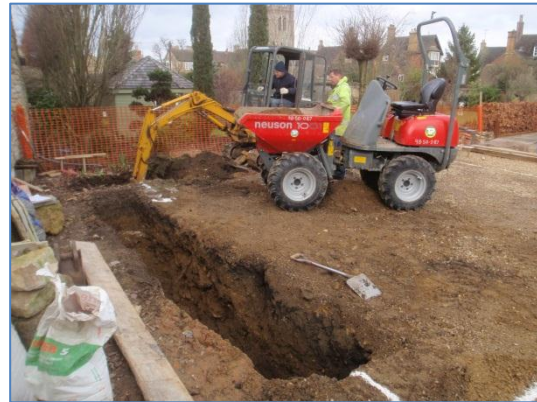
Plate 4: Work in progress, from the south
