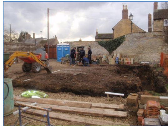
Plate 17: Work in progress, from the east
