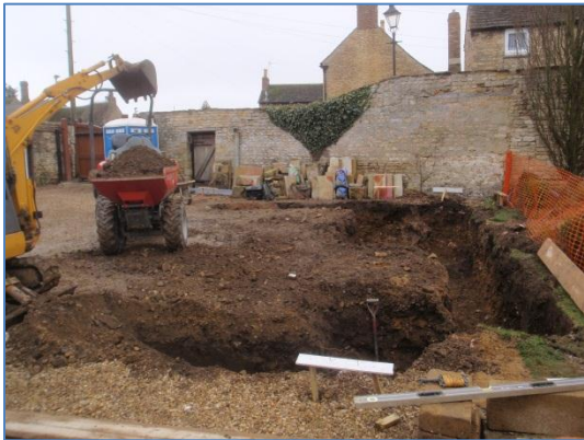
Plate 15: Work in progress, from the east
