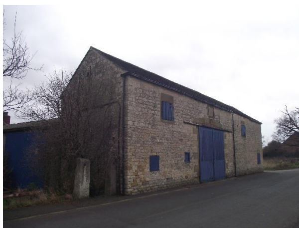
View of the barn along Chapel Lane
