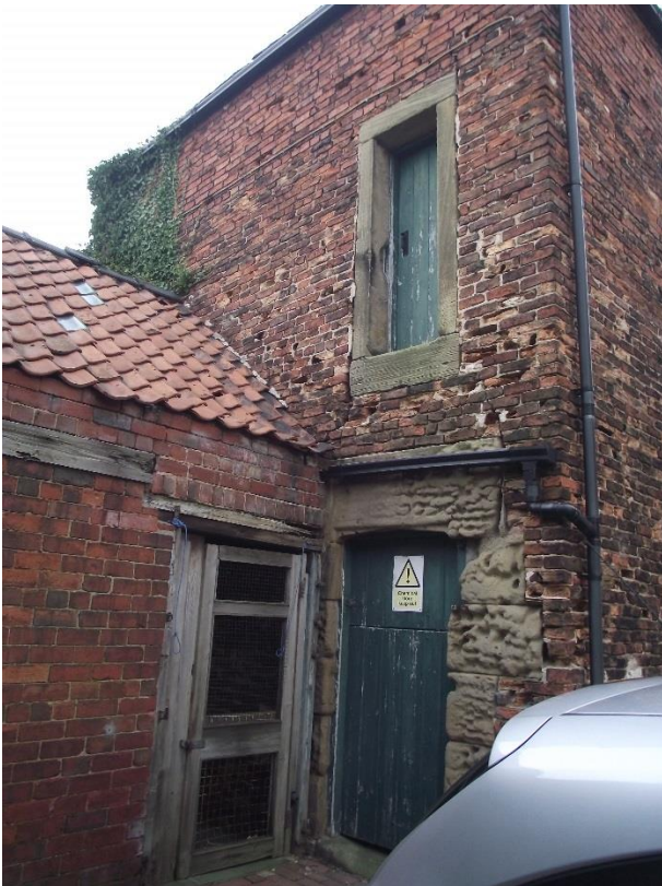
Dovecote ground and first floor entrances (left). Note the ground floor Gibbs style sandstone surround. The east elevation (right) displays a decorative Gothick window
