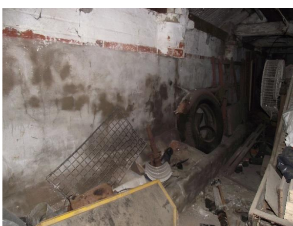
Evidence of the earlier roofline and roofing materials (left) and possible conversion into a milking shed with trough, rendered lower wall with fixings and drainage channel (right)
