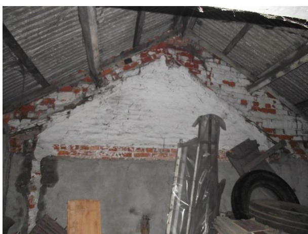
Evidence of the earlier roofline and roofing materials (left) and possible conversion into a milking shed with trough, rendered lower wall with fixings and drainage channel (right)
