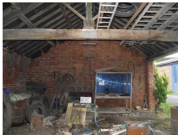
The entrance to the cartshed (left) and an internal view looking west showing the pitch-hole and king post roof (right)
