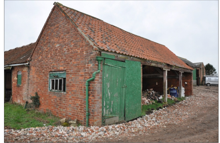
42. Northeast and southeast elevations of Building G, looking W
