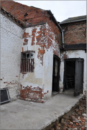
25. Southeast wall forming Building D, looking N
