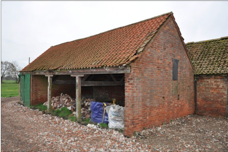
43. Northwest and northeast elevation of Building G, looking S
