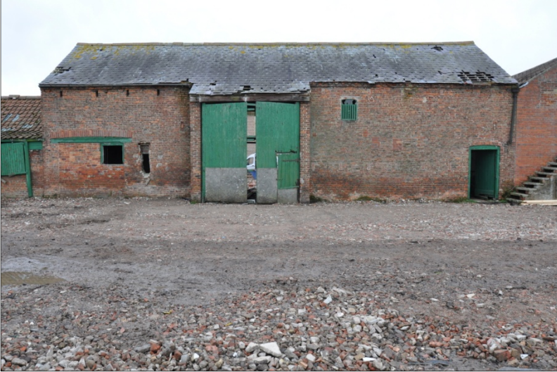
6. Northeast elevation of Building A, looking SW
