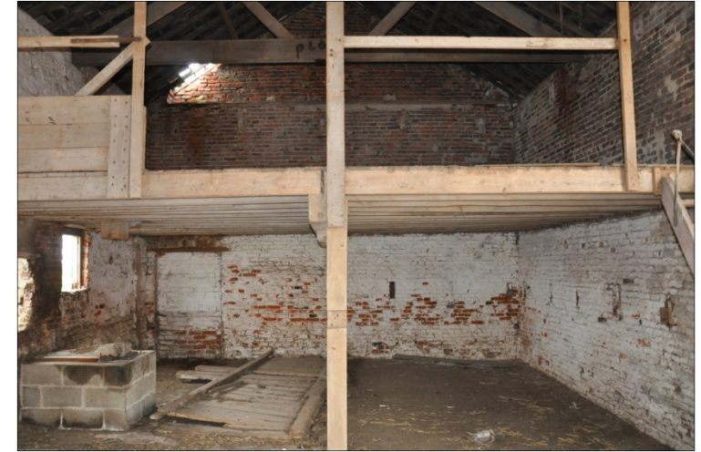
11. Upper floor in Building A, looking SE
