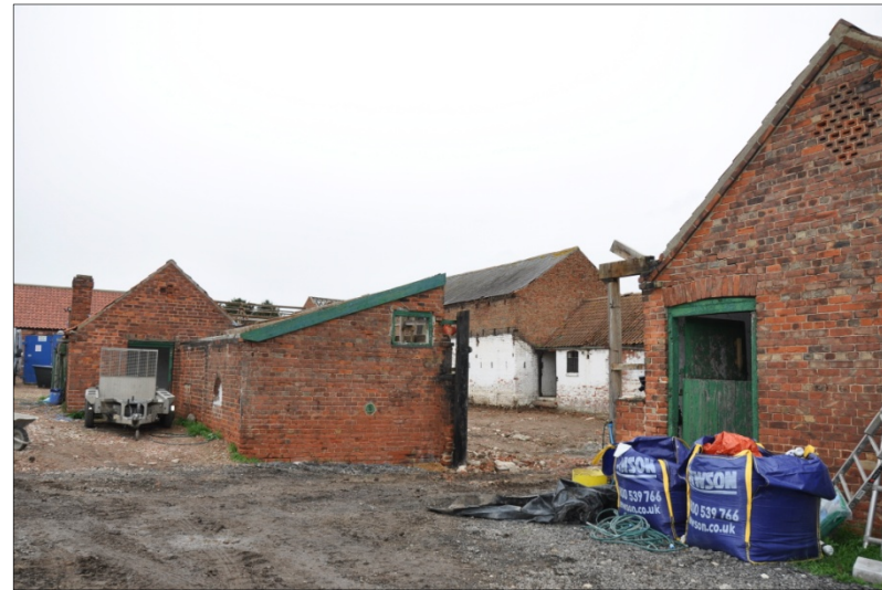
2. Farmstead looking N
