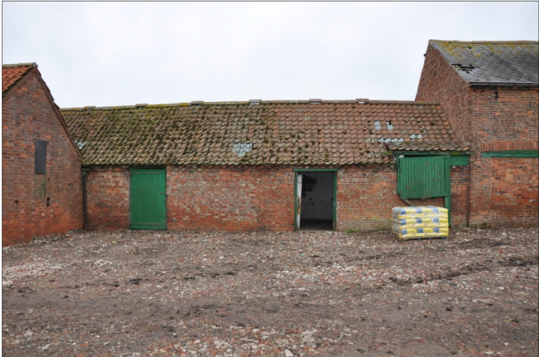
31. Northeast elevation of Building E (centre left) showing building break where it extends Building C (right centre), looking SW
