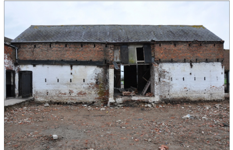
9. Southwest elevation of Building A, looking NE
