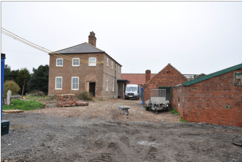
1. Farmhouse and farmstead looking NW
