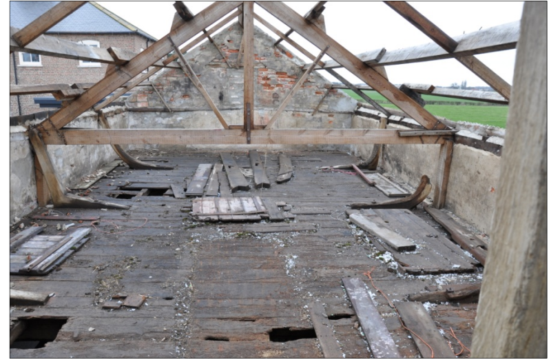
18. Granary above Building B showing unusual timbers, looking SW
