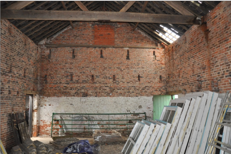
8. Building A, looking NW, showing the internal northwest elevation
