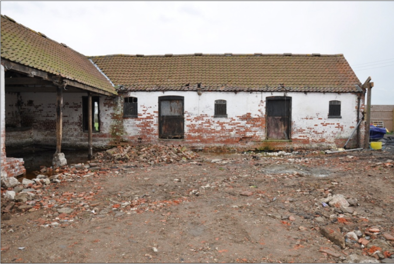
33. Northwest elevation of Building E, looking SE
