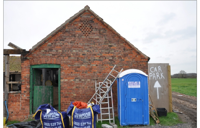
34. Southwest elevation of Building E, looking NE
