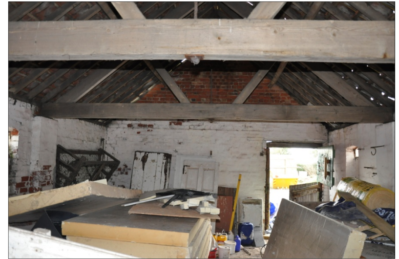
38. Interior of Building E, looking SW
