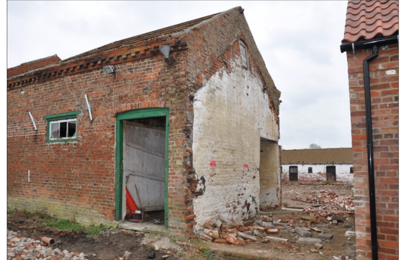
14. Southwest elevation of Building B, looking E
