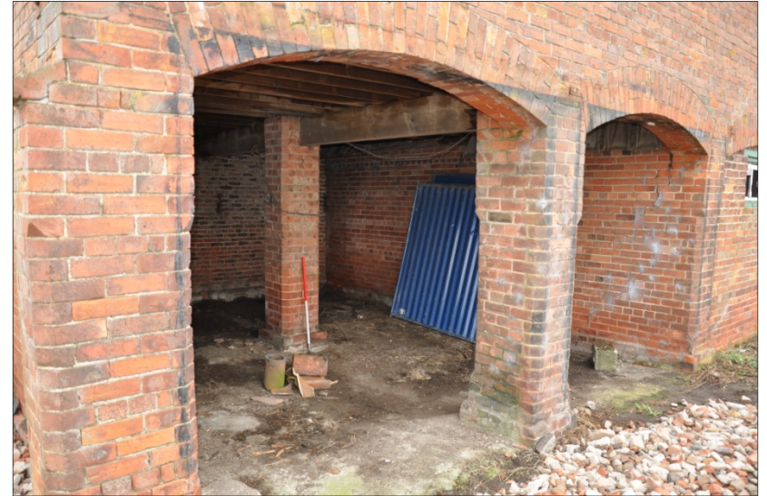
24. Interior of Building D showing original internal wall, looking S
