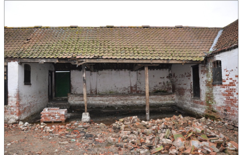
32. Covered stockyard of Building E, looking NE
