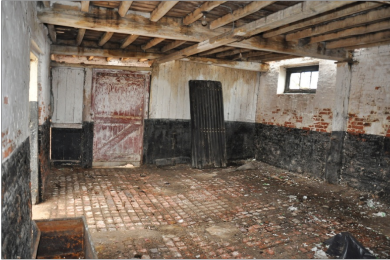
17. Building B interior, showing internal subdivision with timber panel, looking W
