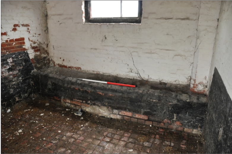
29. Built-in feeder in southwest bay of Building D (1m scale)
