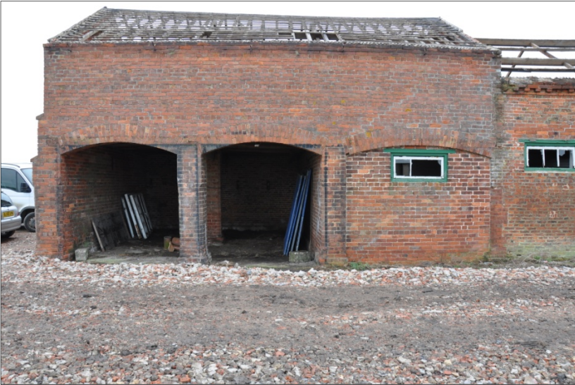
23. Northwest elevation of Building D, looking SE
