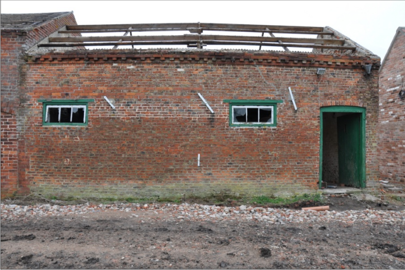
13. Northwest elevation of Building B, looking SE
