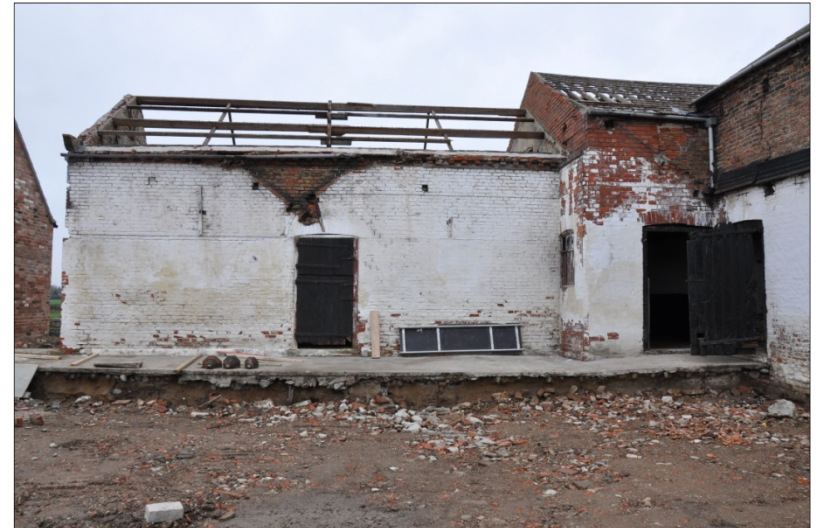
16. Southeast elevation of Building B, looking NW
