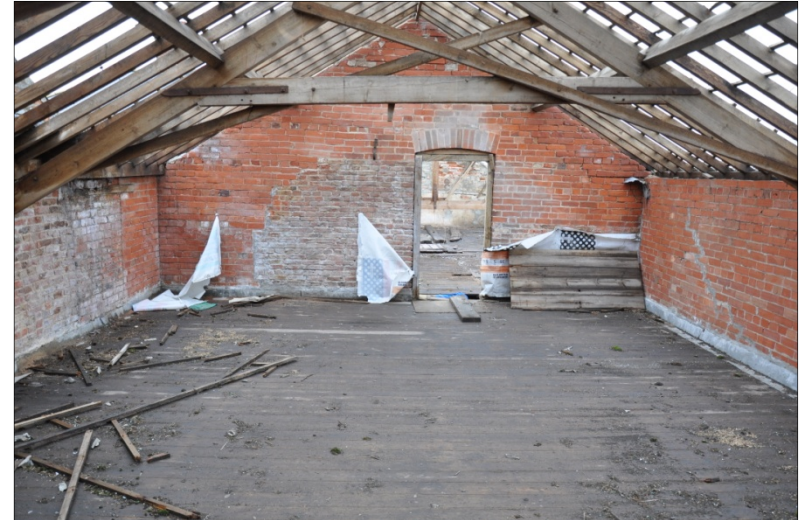
30. Granary floor of Building D, looking SW
