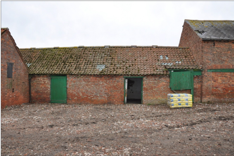
19. Northeast elevation of Building C (right centre) with break in fabric where it was later extended by Building E (left centre), looking SW
