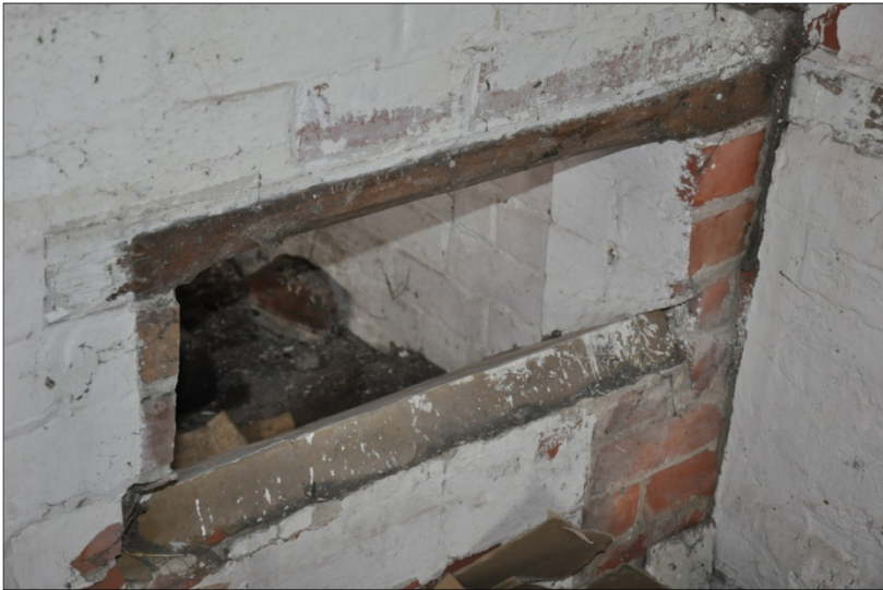
50. Detail of feeding chute from boiler house, looking N
