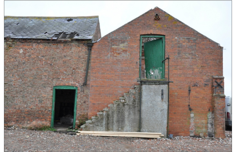
26. Northeast elevation of Building D, looking SW
