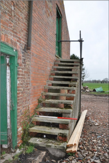
27. Sandstone stair to granary of Building D, looking W
