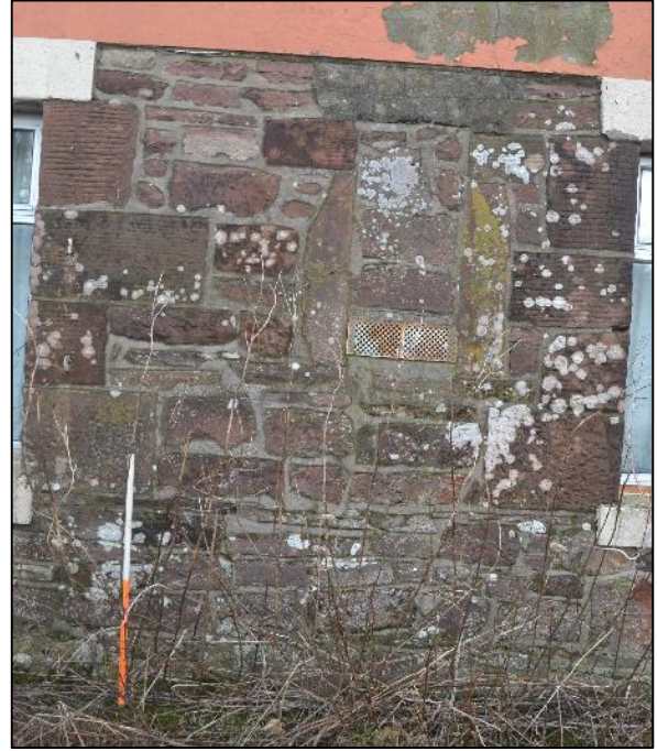
Plate 4: Blocked opening in the main farmhouse (SBR Photograph 039)
