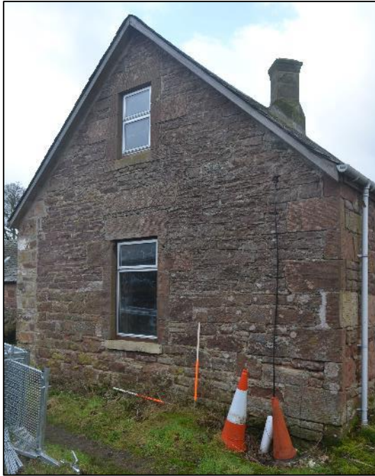
Plate 3: East facing gable of building showing change in masonry/construction breaks. Note the re-working of the N facing elevation (left) (SBR Photograph 005)
