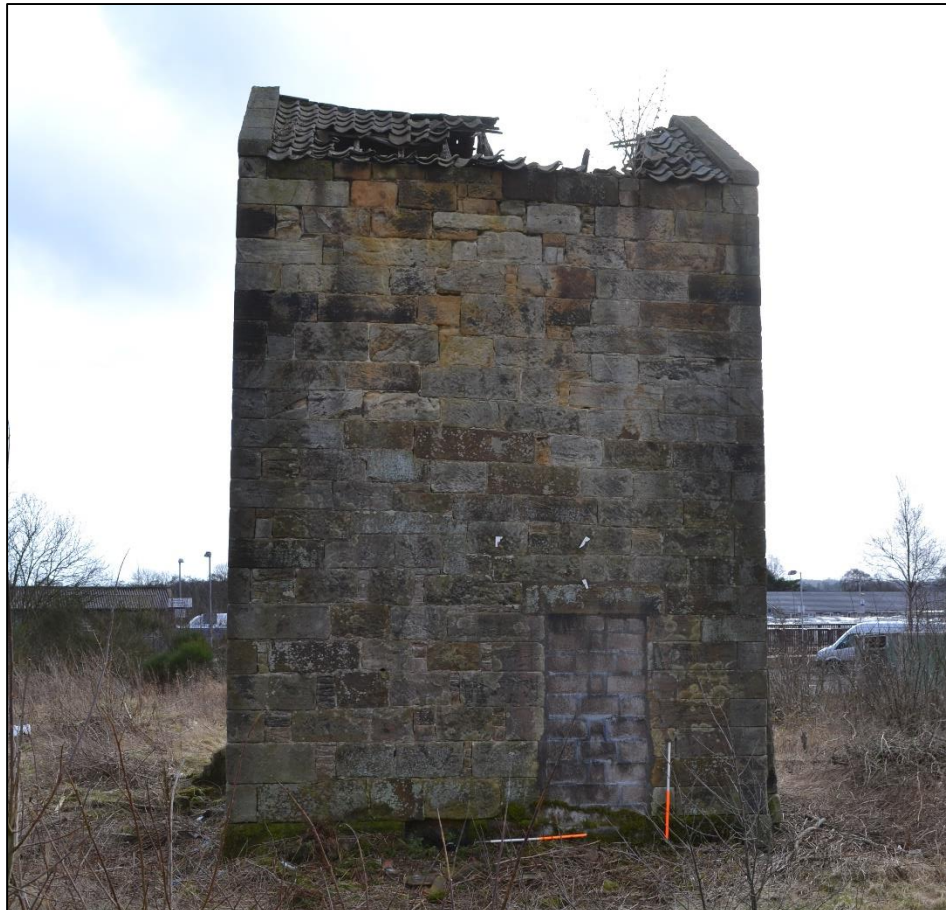
Plate 5: North elevation of the Beam Engine House (Photograph 012)
