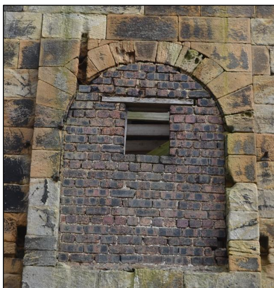
Plate 11: Detailed view of opening for the Beam in West Elevation (Photograph 037)
