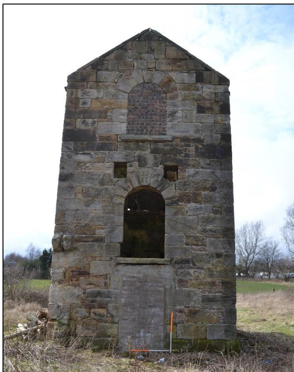
Plate 6: East Elevation of Thornton Beam Engine House (Photograph 016)
