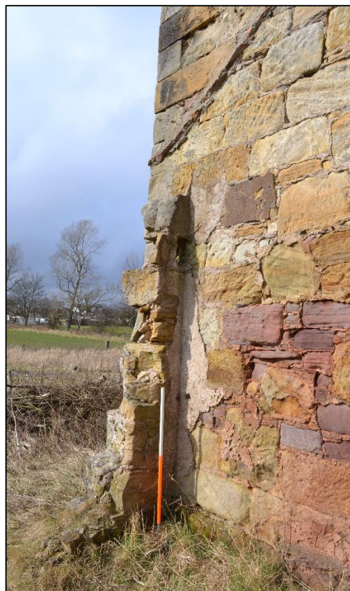
Plate 9: Detail of wall stub retaining plaster from the south east. Note the line of the raggle (top) and scorched stonework (right) (Photograph 034)
