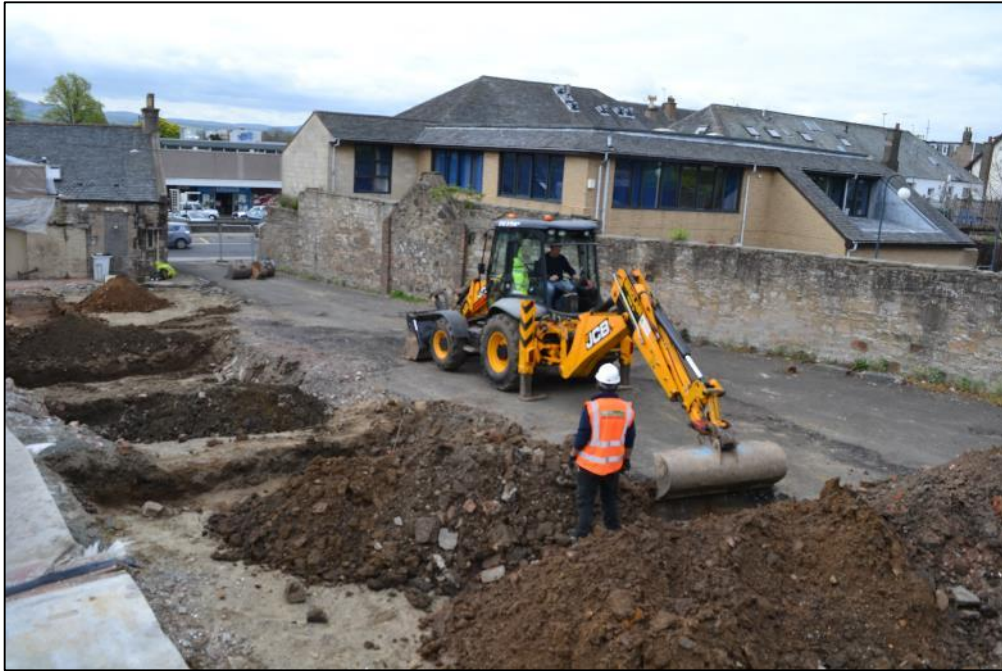
Plate 16 : Working shot showing trenches being opened across site (Photograph 074)
