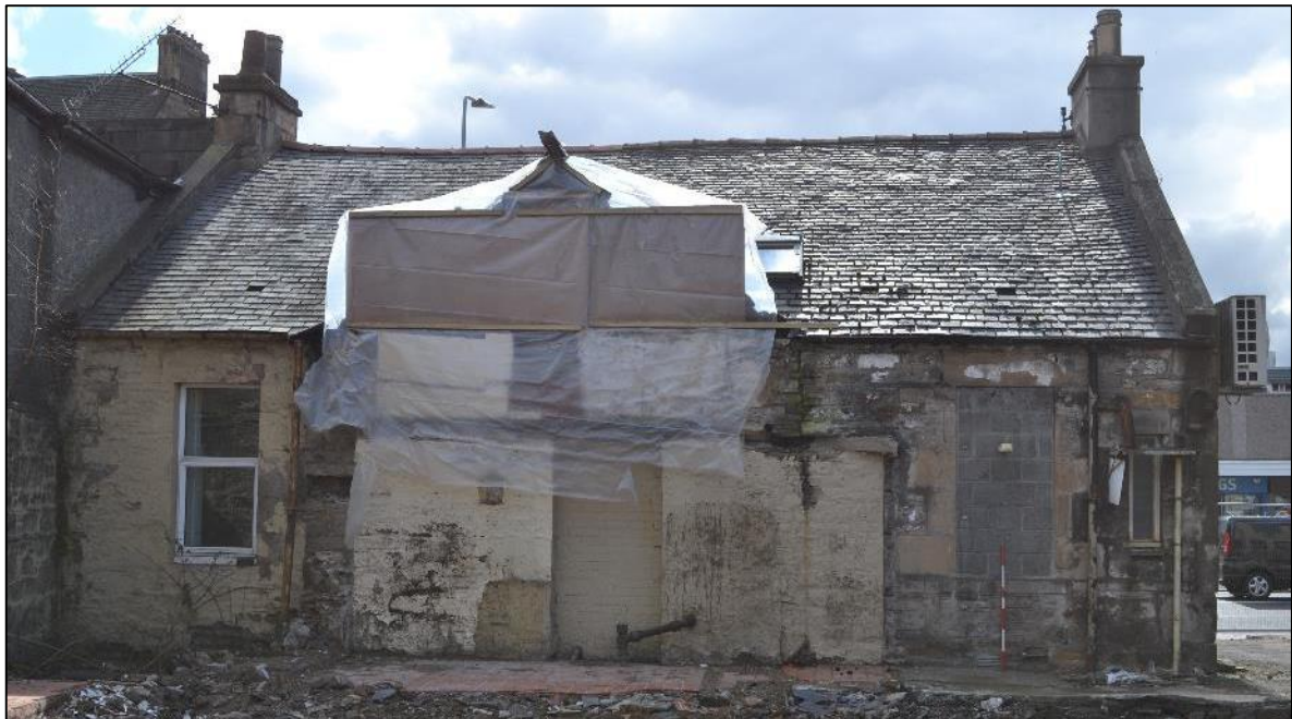
Plate 9: Rear (North facing) external elevation of the 'cottage' (Photograph 022)
