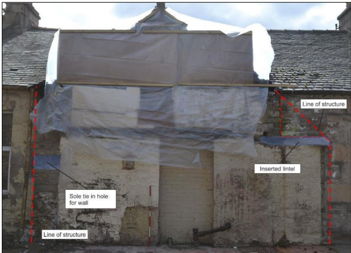
Plate 10: Middle of rear façade showing scars from secondary (now demolished) additions to the 'cottage' (Photograph 024)
