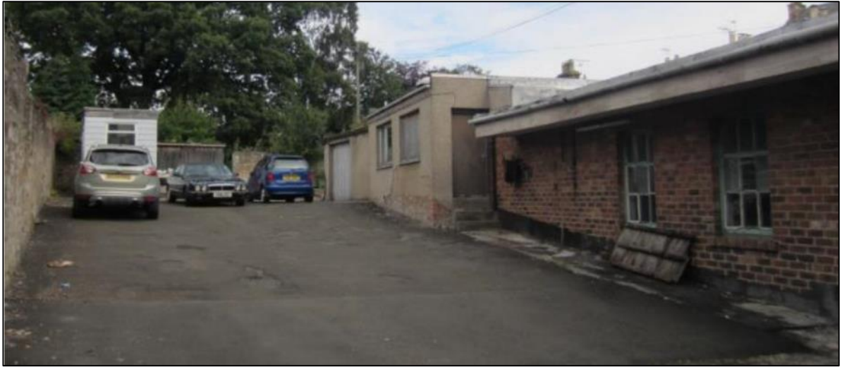
Plate 4: Looking north east across the demolished structures Image courtesy of Pink Architects
