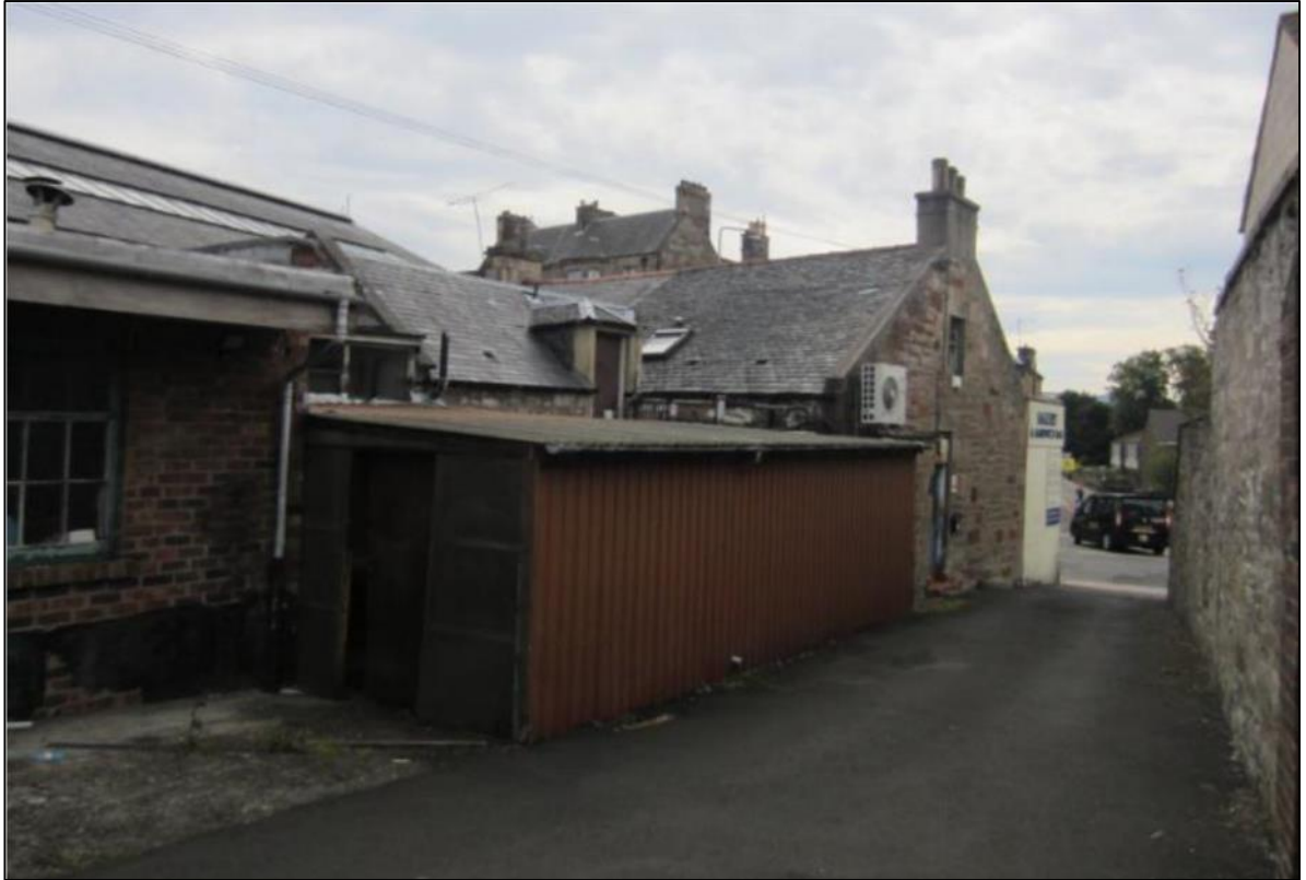
Plate 2: Looking south across the demolished structures Image courtesy of Pink Architects
