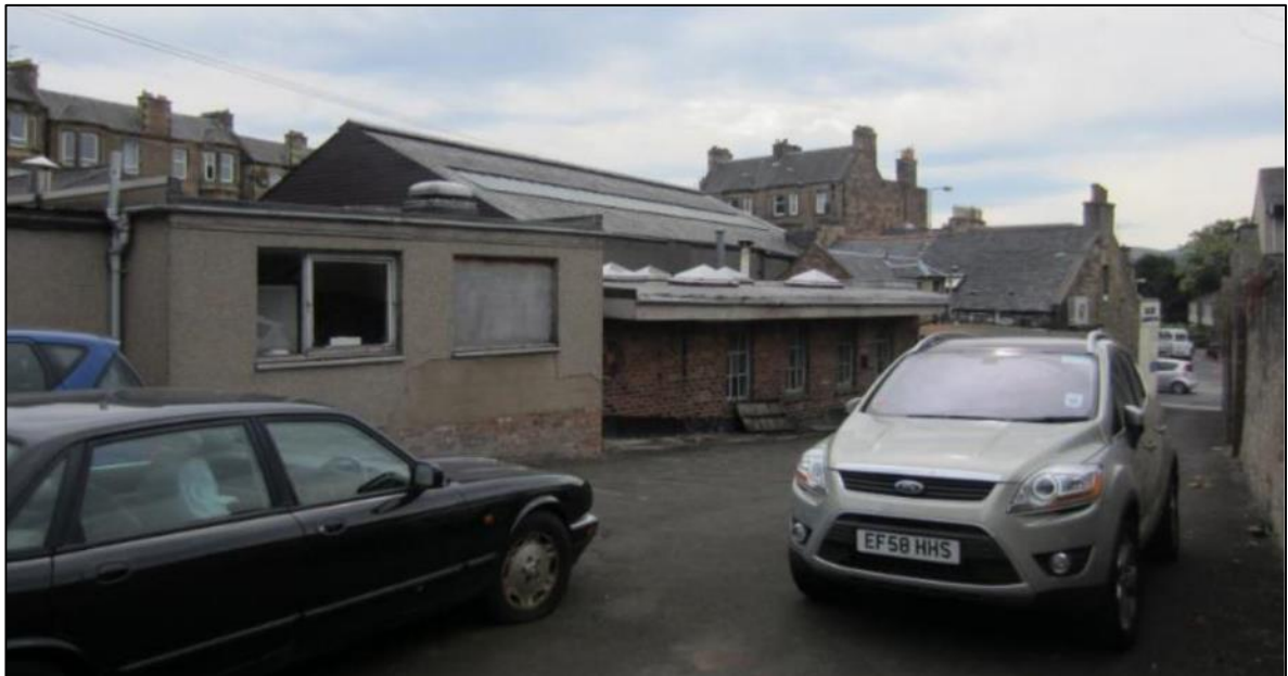
Plate 5: Looking south west across the demolished structures Image courtesy of Pink Architects
