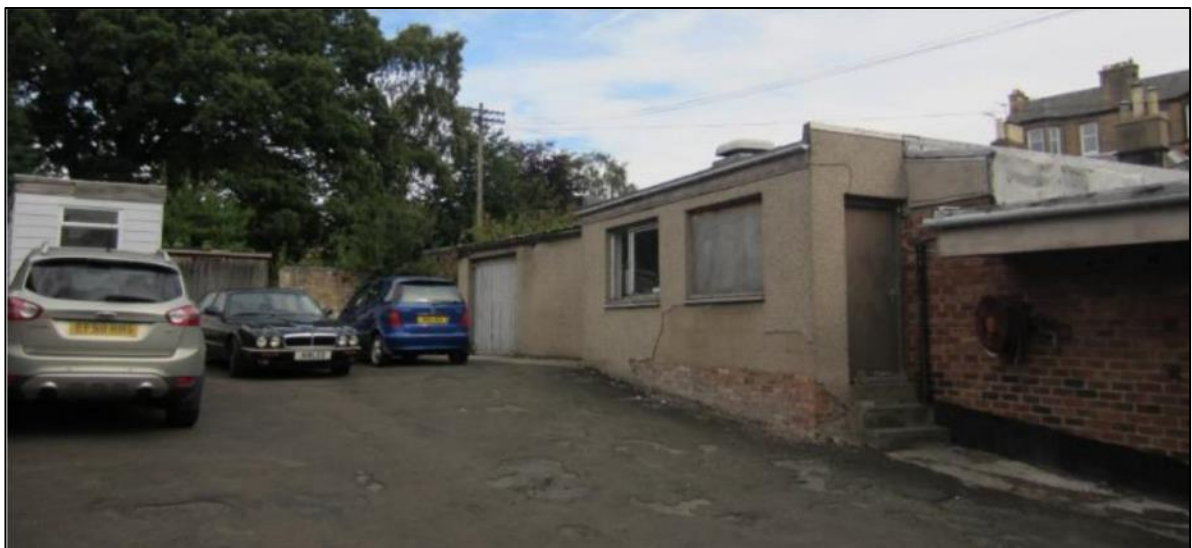
Plate 1: Looking north east across the demolished structures Image courtesy of Pink Architects
