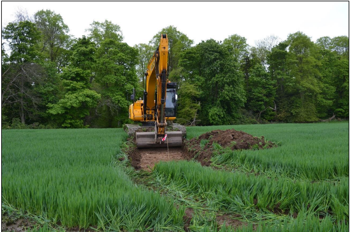
Plate 7: Working shot showing Trench 4 being opened
