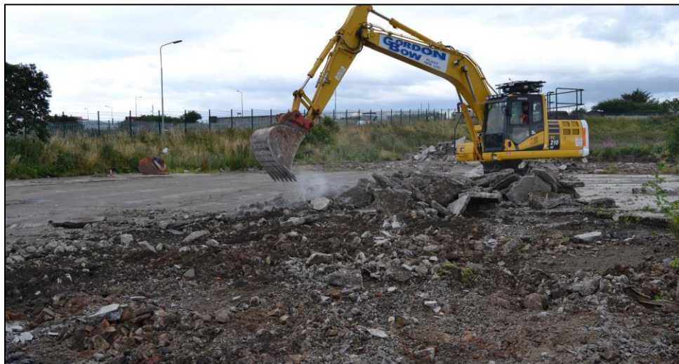
Plate 2: Removal of the concrete capping under watching brief conditions (Photograph 025)
