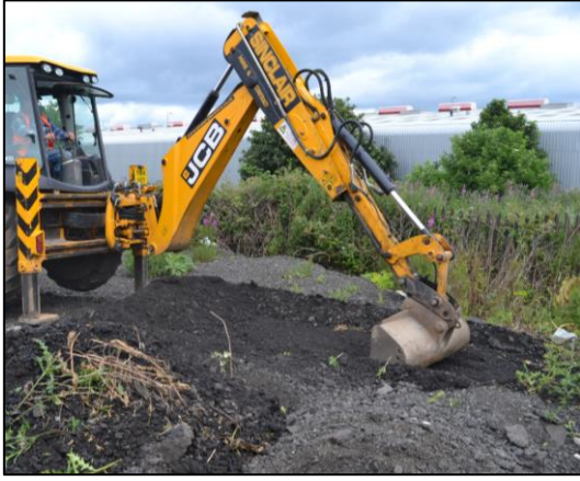
Plate 5: Working shot – opening Trench 1 (Photograph 003)
