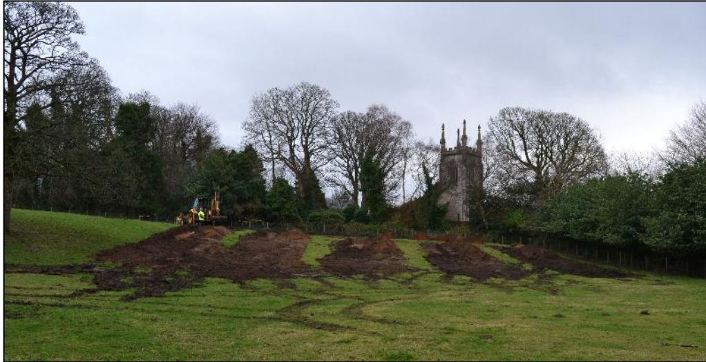
Plate 2: Working shot showing the locations of the trenches during backfilling (Photograph 039)
