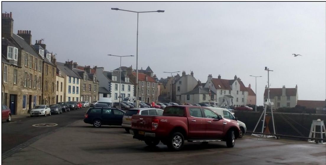
Plate 1: Looking east along East Shore, with the proposed development site at 14-15 East Shore visible as the three storey building on the left of the image (Photograph 007)
