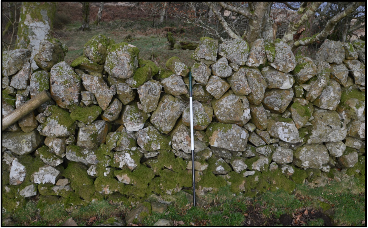
Plate 3: North-facing detail of drystone walling at Loskie East, main enclosure.
