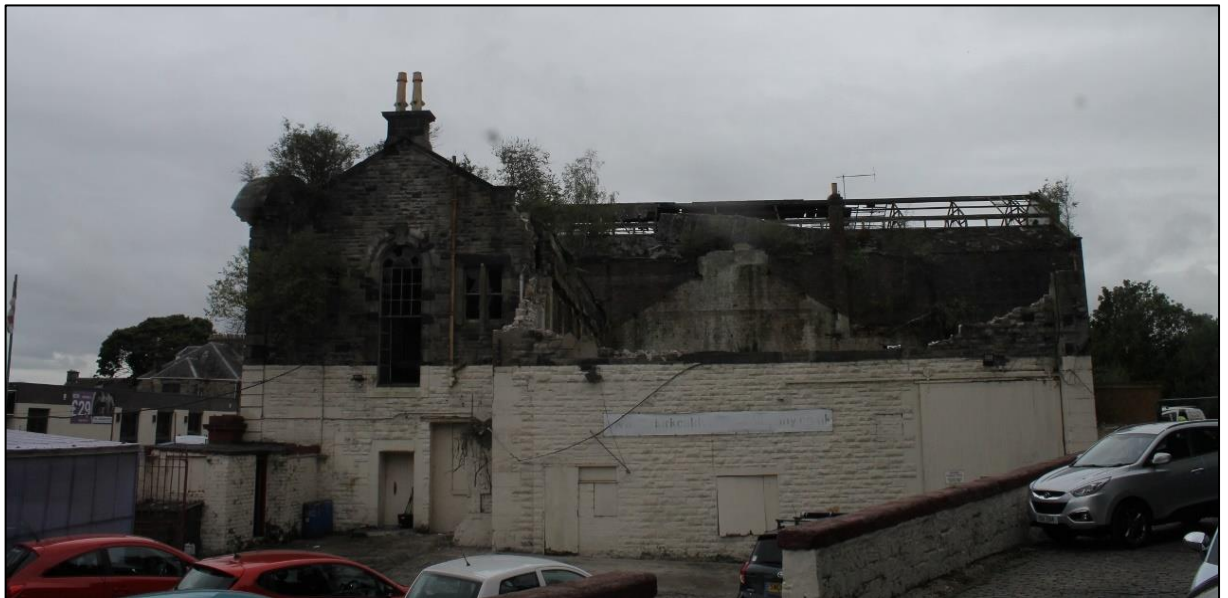
Plate 6: East elevation, after demolition (Photograph 005)
