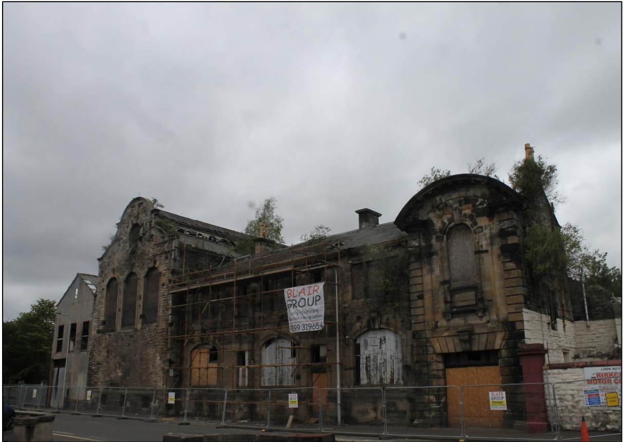
Plate 9: South Elevation from the east (Photograph 050)
