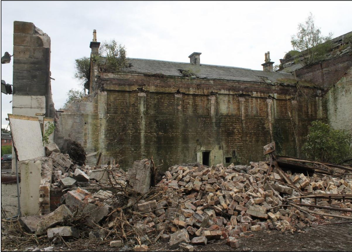
Plate 3: Demolished east side of the north elevation (Photograph 003)
