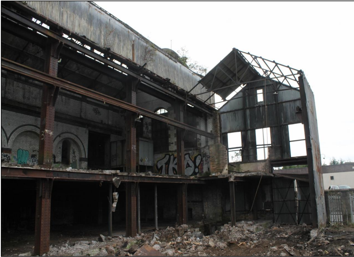
Plate 23: Interior; south and remains of the west elevation (Photograph 022)
