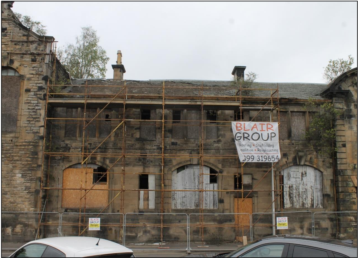
Plate 11: South elevation central bays (Photograph 011)
