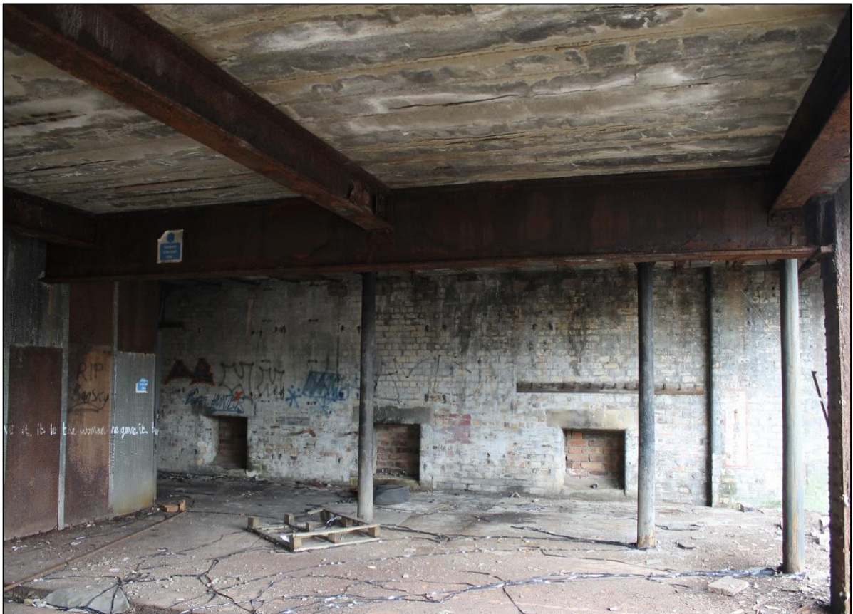
Plate 22: Interior; south elevation (Photograph 041)
