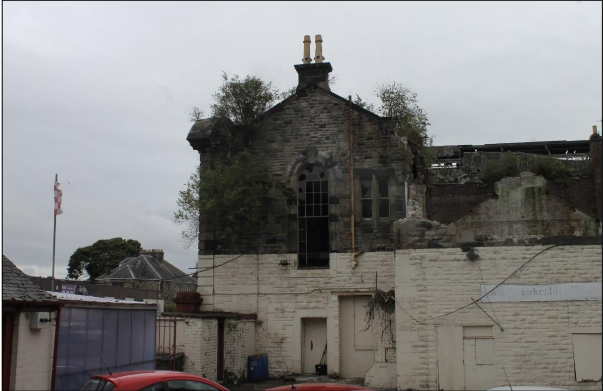
Plate 7: East elevation, south side/bay still standing (Photograph 006)
