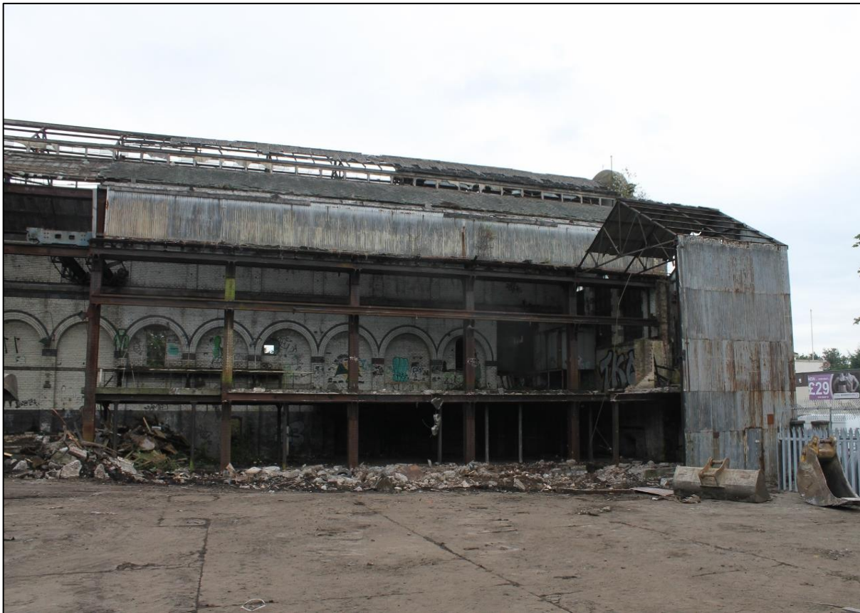
Plate 4: West elevation demolished prior to building recording (Photograph 014)
