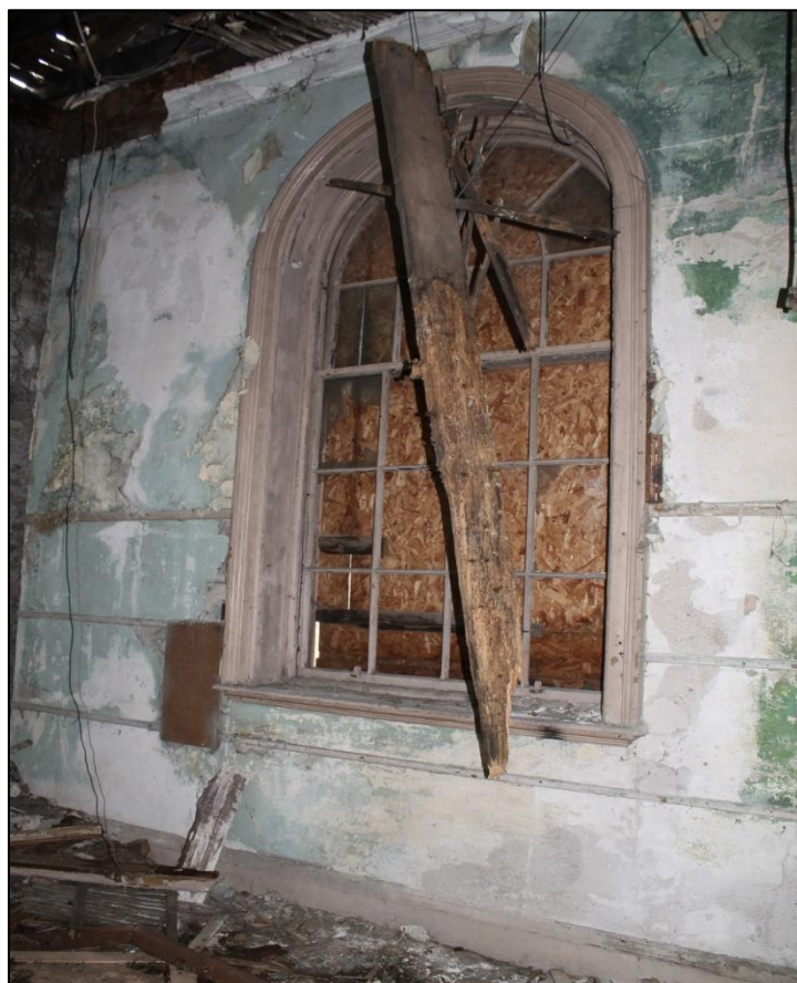
Plate 20: First floor; east room (Photograph 036)
