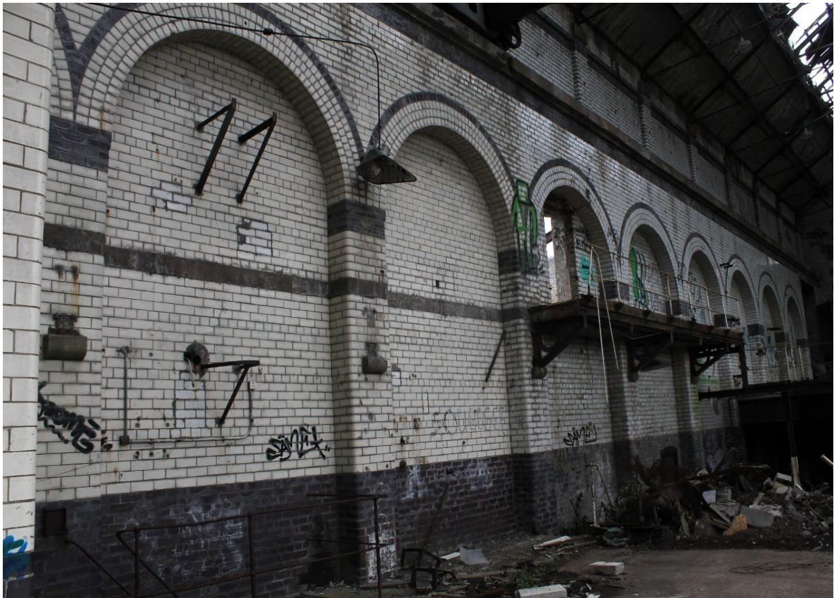
Plate 24: East elevation; showing the eight enamel glazed polychrome bricks arches (Photograph 020)
