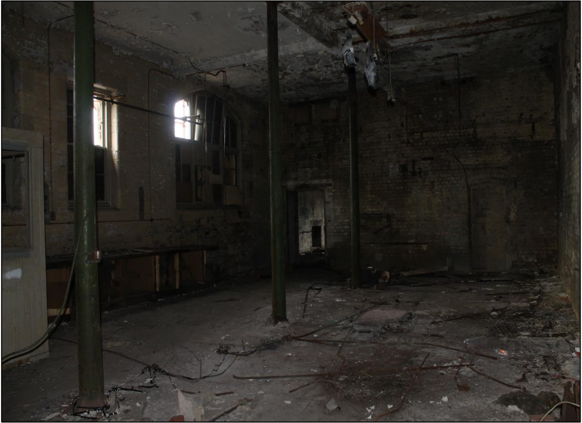
Plate 15: Room 1; west elevation (Photograph 027)
