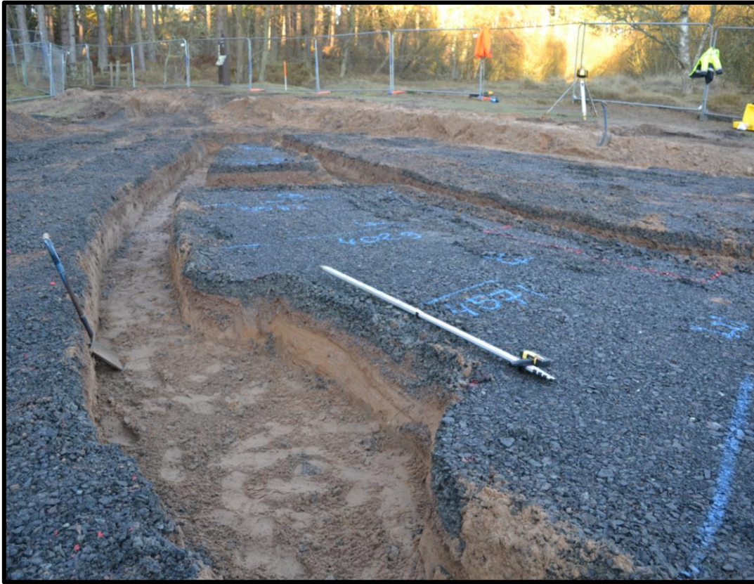
Plate 4: Excavation of foundation trenches
