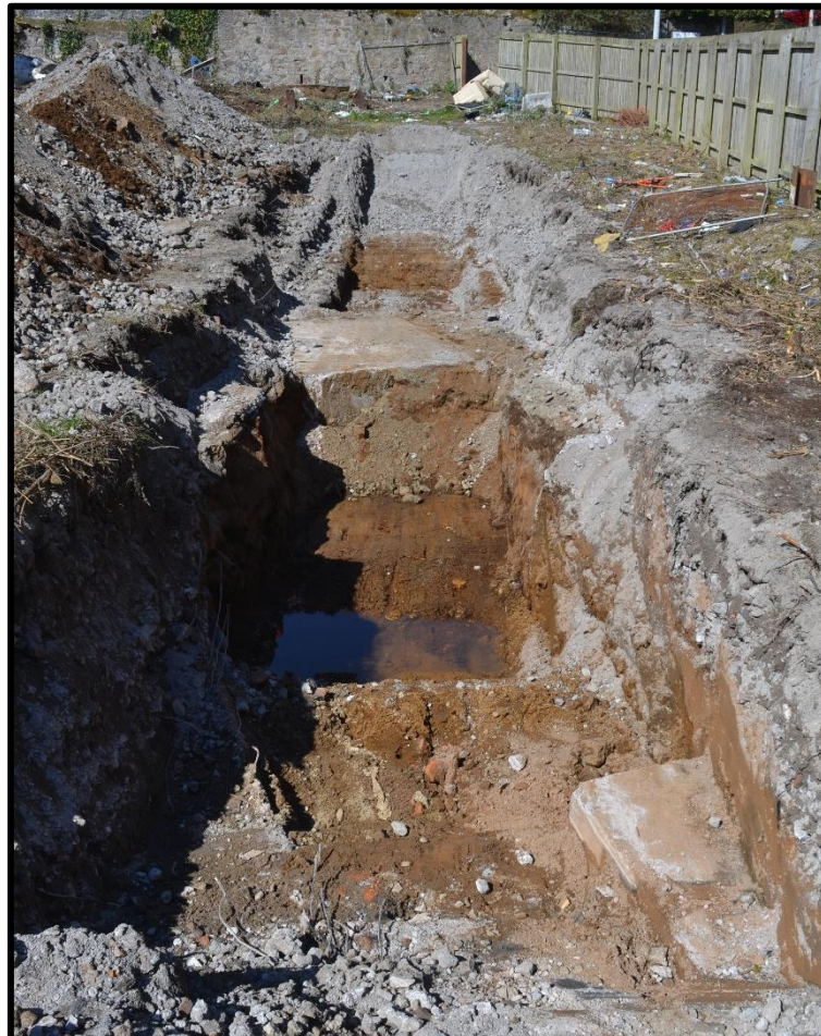
Plate 2: Trench 2 from south-east with the two concrete plinths visible
