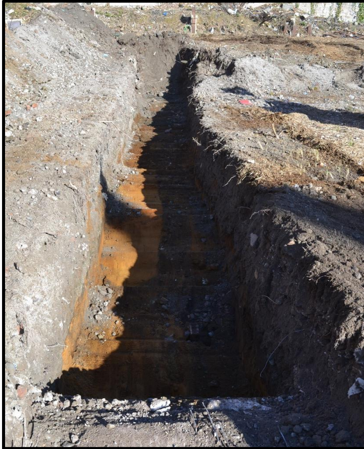
Plate 4: Trench 4 from south
