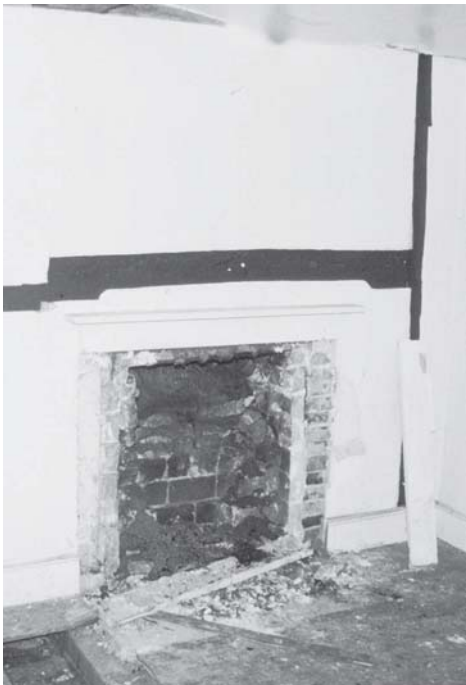
(c) Primary fireplace within Room FF08 before (left) and after (right) stripping
