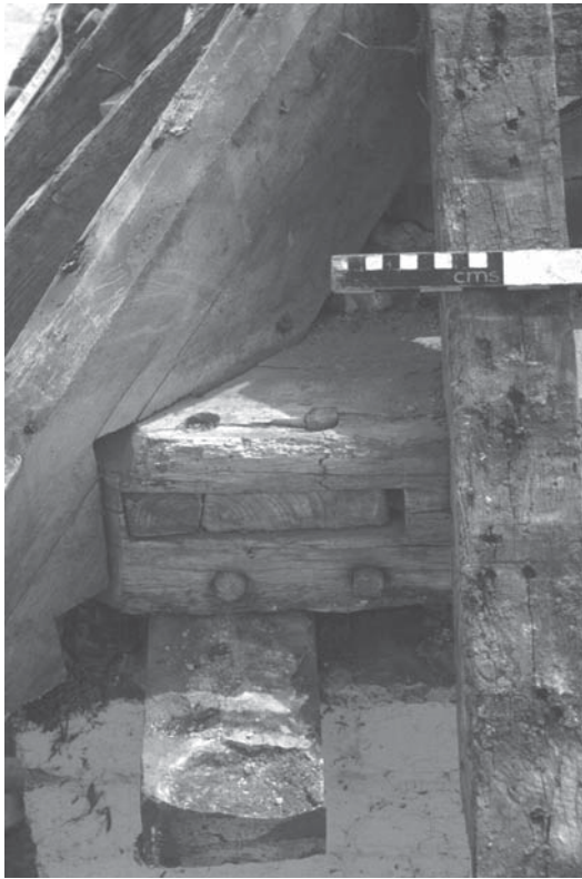
(a) sawn off tenon in outer face of north plate, east end
