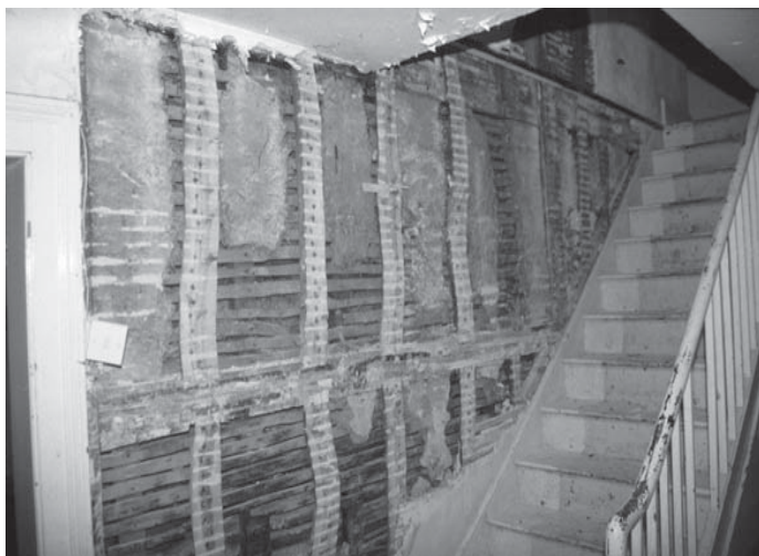
(a) Room GF03: north wall of stair
