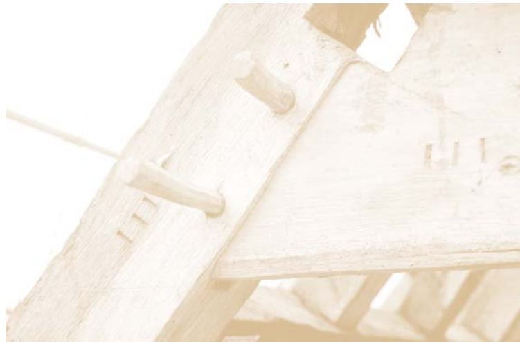
(c) Principal Rafter [ III ] (NB. chiselled marks)
