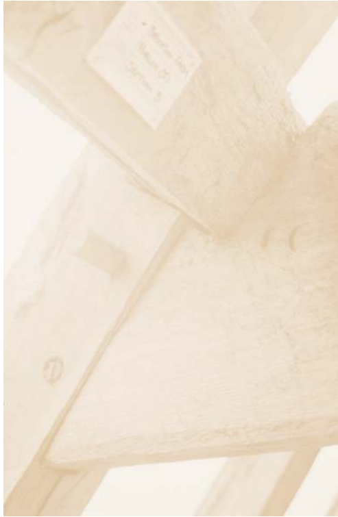
(a) Principal Rafter [ ( ) ] (NB. gauged marks)
