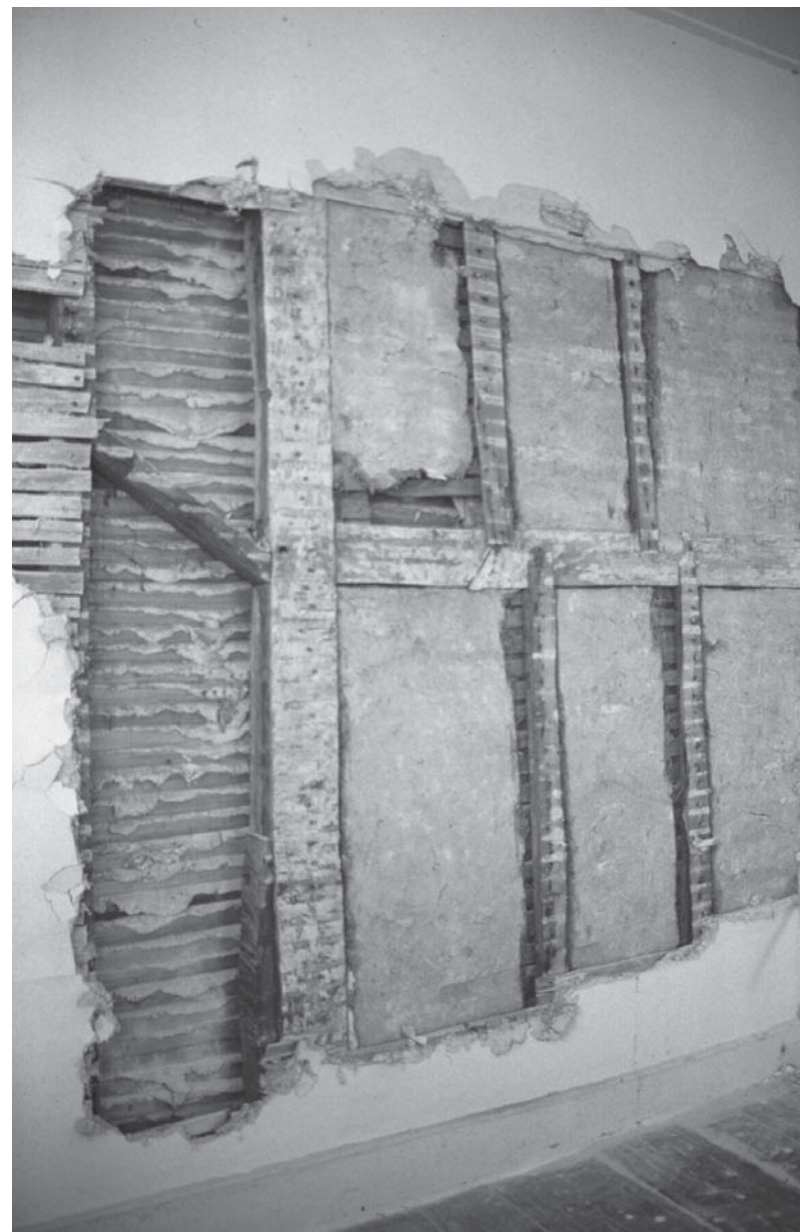
(c) Room FF01: south wall; note daub infill panels applied to laths
