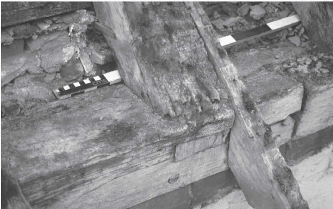
(c) sawn off tenon in outer face of north plate
