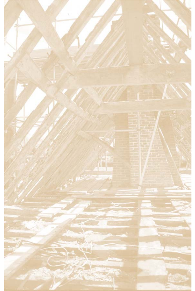
(d) General view along 17th-century roof towards contemporary brick stack
