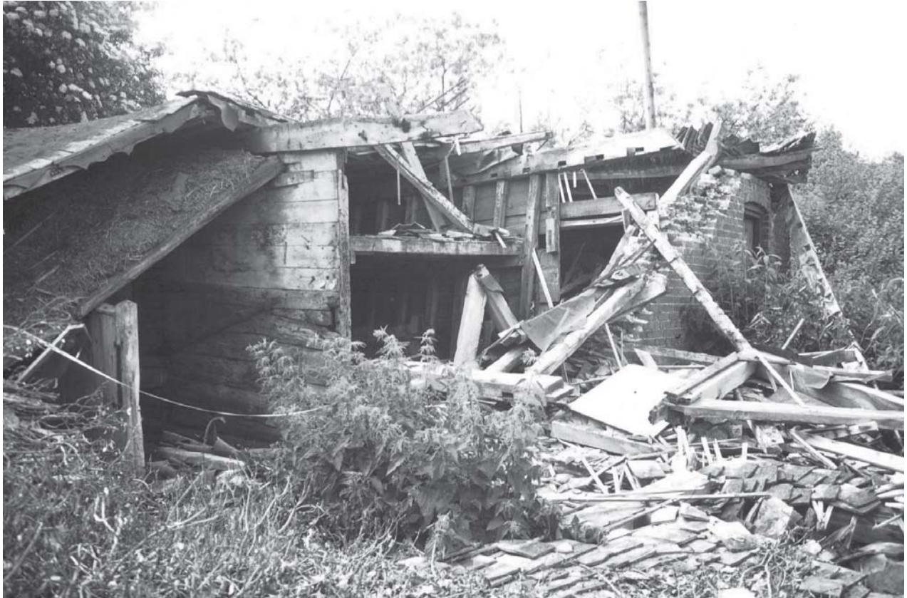
(a) general view from south-east
