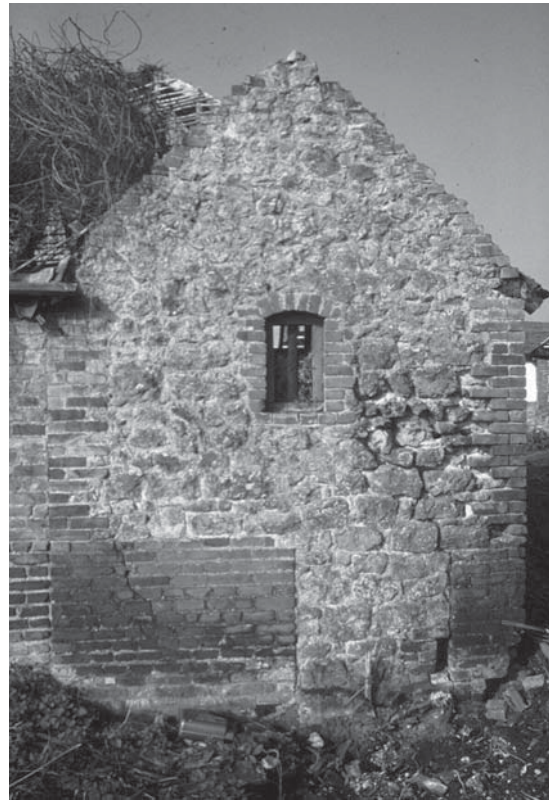
(c) east elevation; northern gable end
