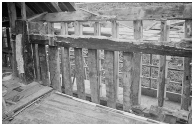
Plate 4: Bay 3(S); Phase I studwork with inserted studwork beyond (below bressummer) for support of tile hanging.
