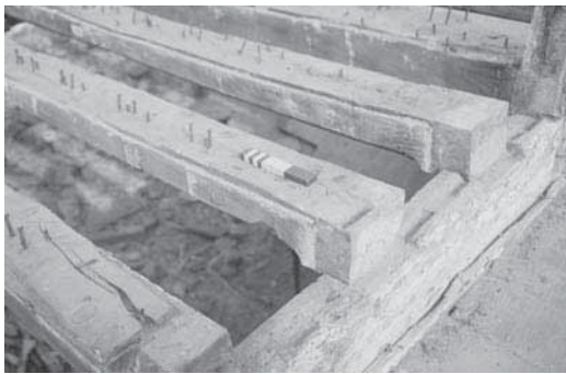
(b) At the high end of the hall, the common joists of the inserted floor are supported by packing pieces atop the pre-existing dias beam (left) or, in certain cases, are cut into the arch bracing of the end elevation (right).
