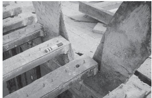
(b) At the high end of the hall, the common joists of the inserted floor are supported by packing pieces atop the pre-existing dias beam (left) or, in certain cases, are cut into the arch bracing of the end elevation (right).
