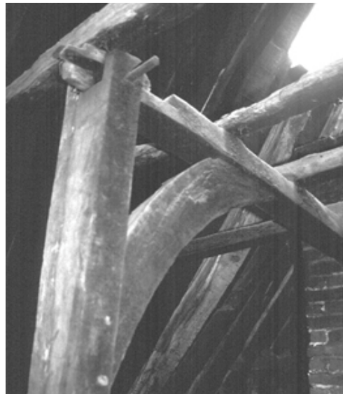
Plate 3: Surviving crown-post, arch brace and collar purlin at CF3.
