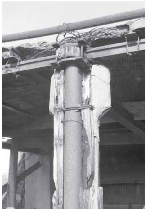
Plate 7: Detail of projecting roof support pillar
