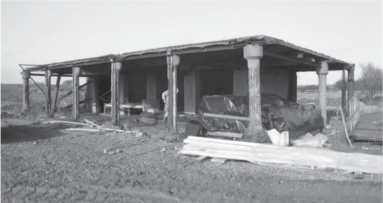
Plate 1: General view from the south-east
