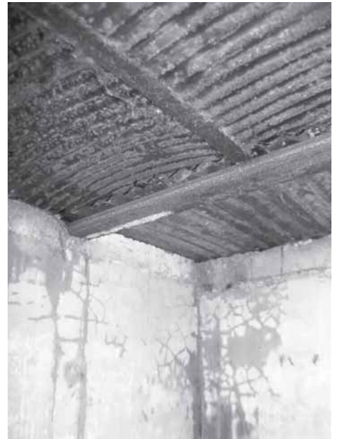
Plate 6: Detail of roof structure
