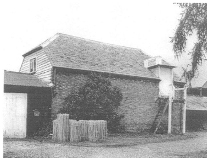
Plate 8: East elevation of granary
