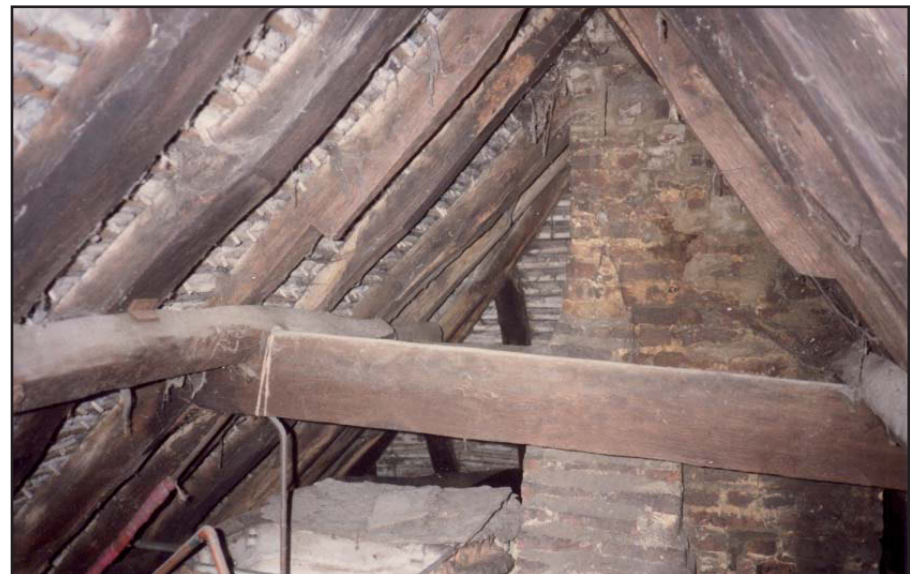
Plate 4: Roof truss and chimney
