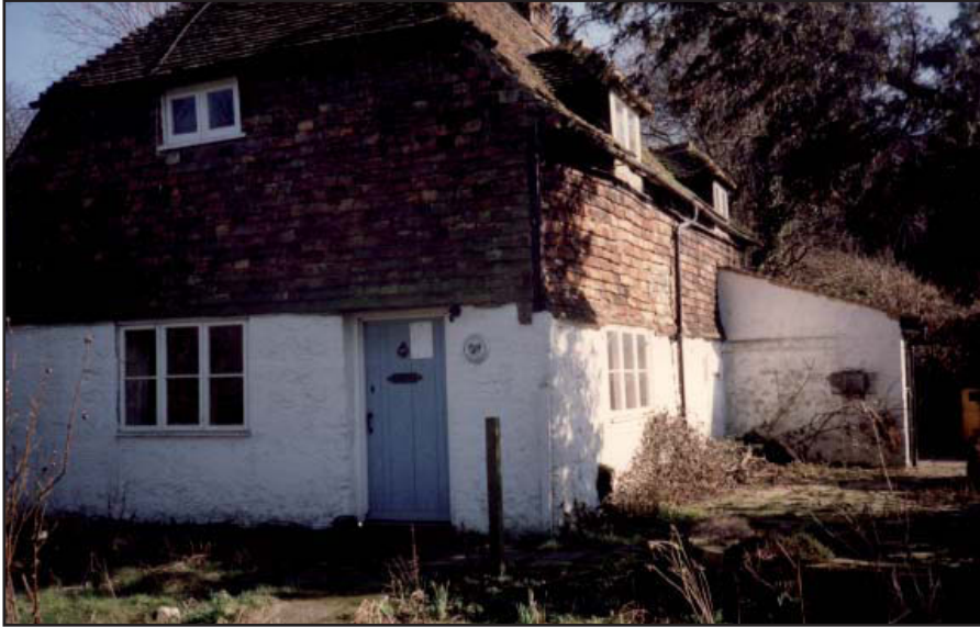
Plate 1: General view, west elevation
