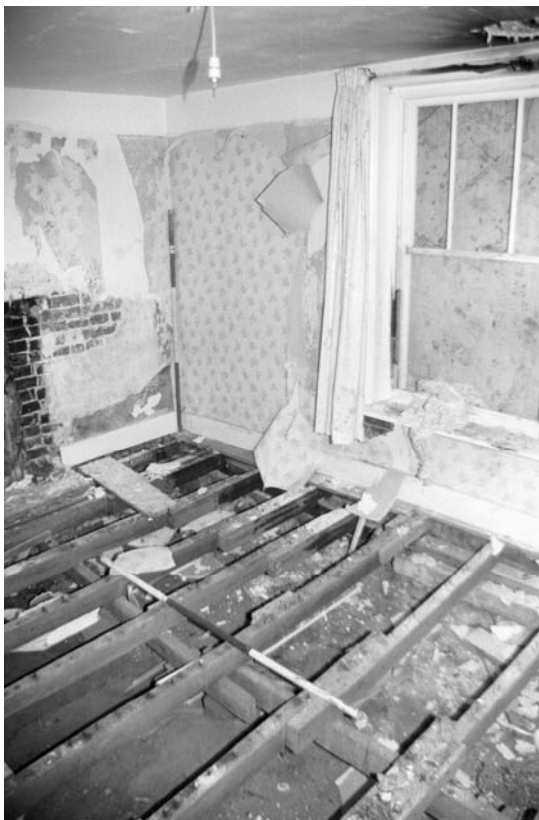
Figure 19: Room GF03 looking south-east
