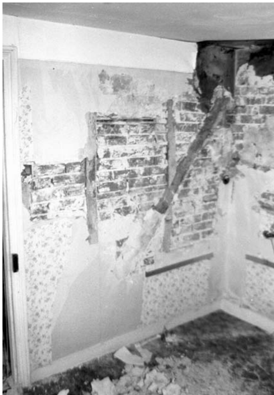
Figure 17: Room GF02 north wall (east)
