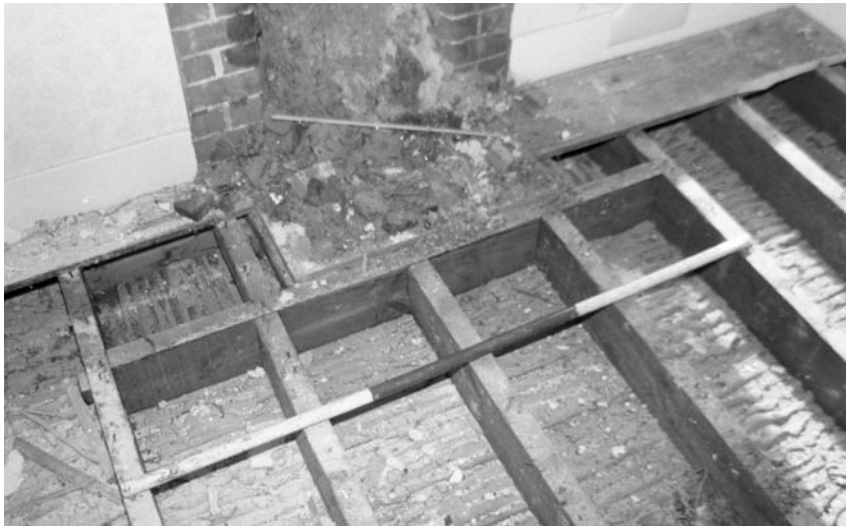
Figure 26: Room FF02, detail of first floor construction plus fireplace trimmer
