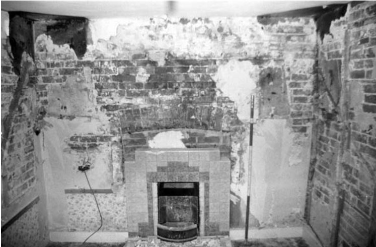
Figure 23: GF02, east wall, note area of rebuild to upper wall
