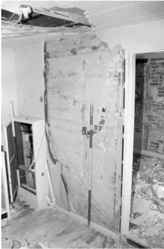
Figure 12: Room GF01, south wall
