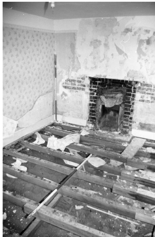
Figure 20: Room GF03 looking north-east
