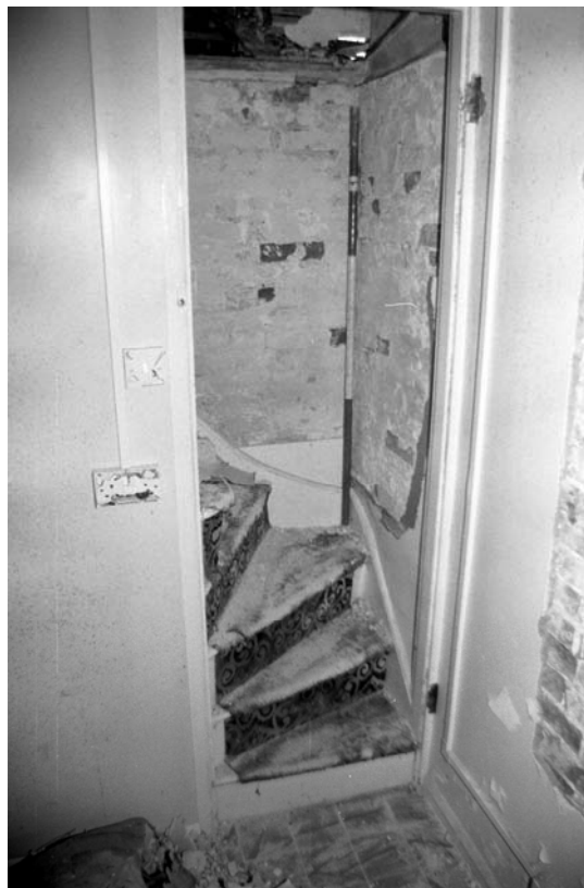
Figure 14: Room GF01(W), door to stairway GF06
