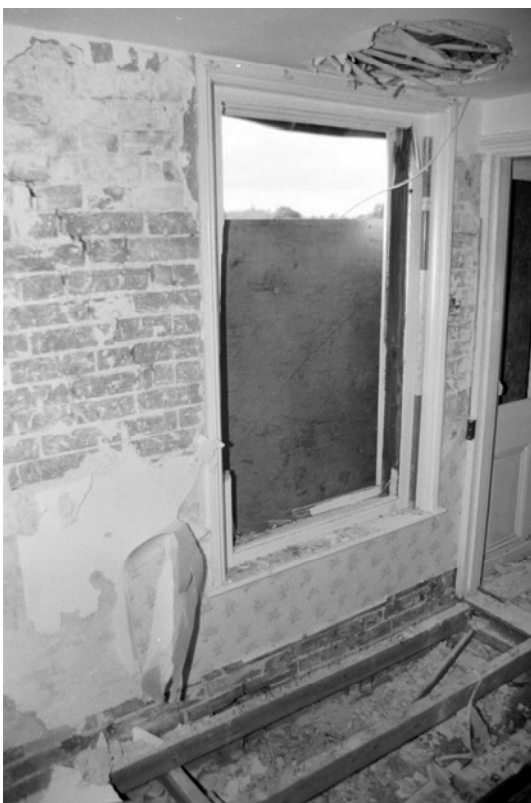
Figure 21: Room GF03 looking north-west
