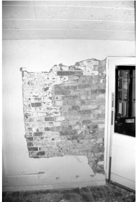
Figure 13: Room GF01, north wall: note area of rebuild to western jamb
