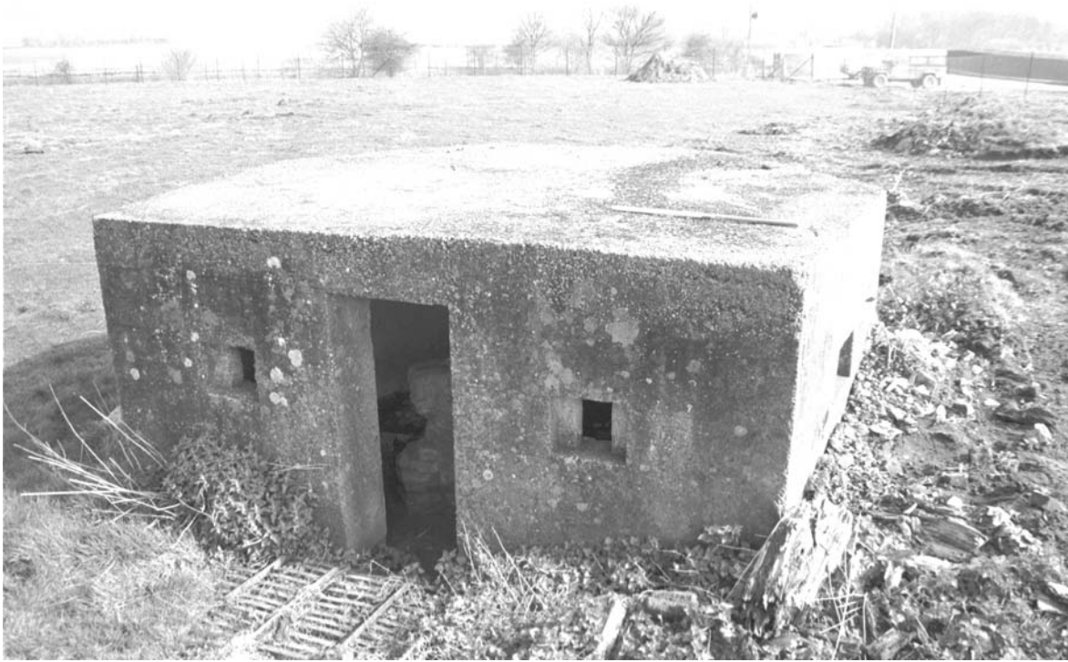
Plate 1: Pill Box A, south-west elevation
