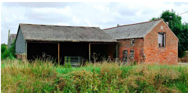
Outfarm with stacking yard and two cart shed extensions off a main brick threshing barn. (The Fens)
