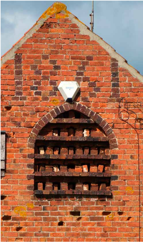
Left: 19th century 5 tiered pigeon loft in barn gable. (Humberhead Levels) © Jen Deadman)
