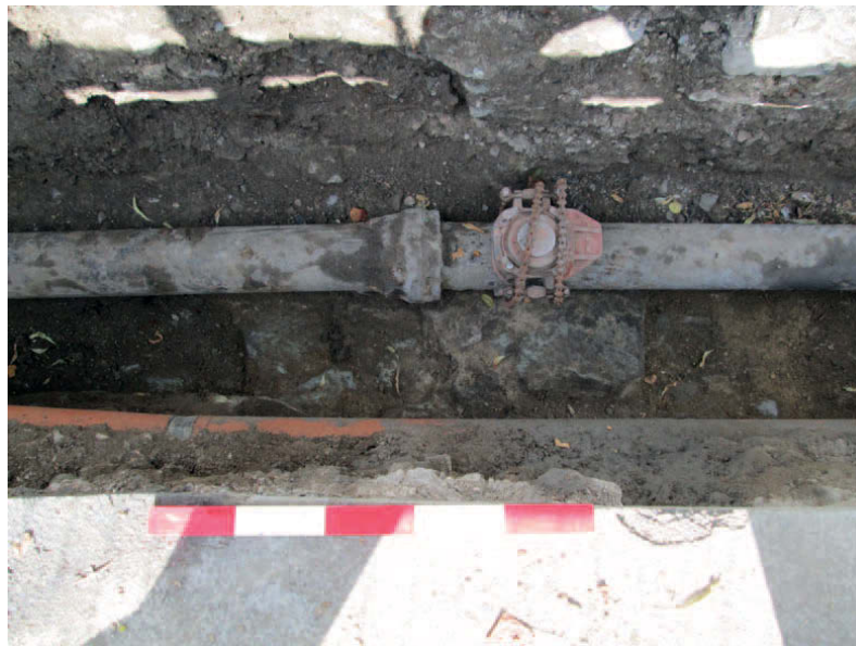
Trench 1; view of walls 1004 and 1005, looking north-west. (Scale 0.5m)
