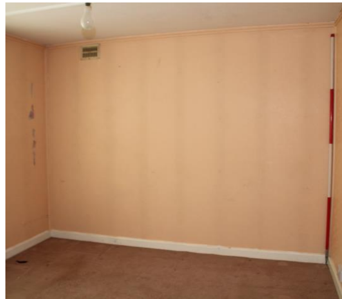
Photo 78: North elevation of the front bedroom of Number 36. Note vertical shading of the concrete panels through the wallpaper.
