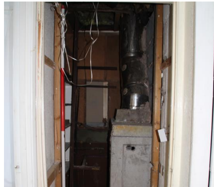
Photo 38: View of the 'boiler void' behind the north elevation of living room of 1 West Street. Evidence of original flue retained.
