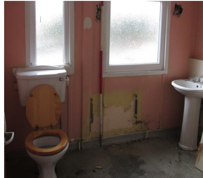
Photo 33: South elevation of the converted bathroom / W.C at 1 Pipeyard Lane. The former remnant of the former dividing wall right of the W.C.
