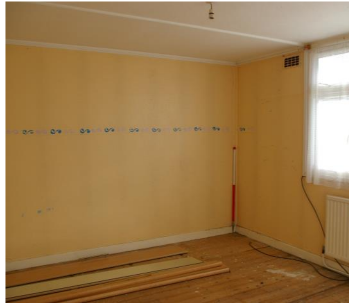
Photo 50: The south elevation of the back bedroom of 38 Pitt Street. Note the vertical lines of the concrete panels seen through the wallpaper.
