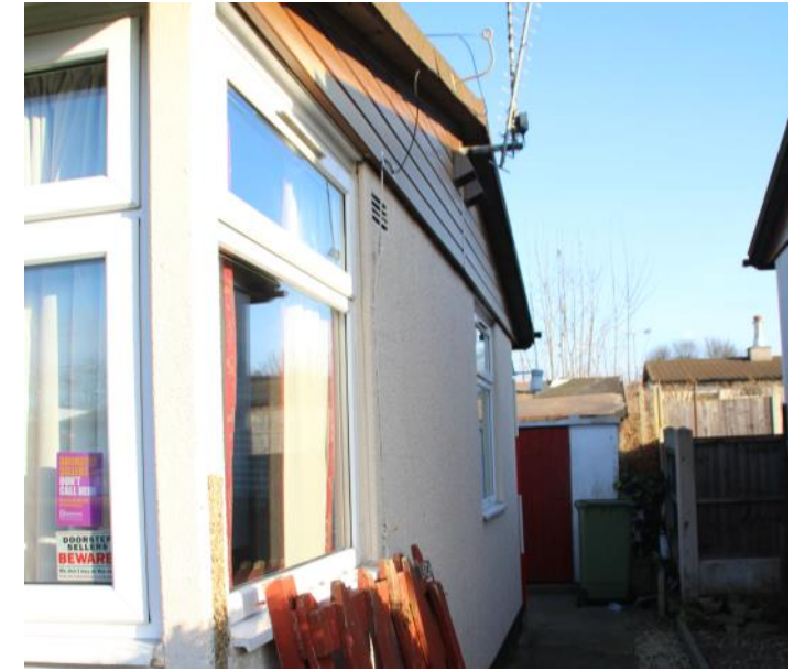
Photo 80: South exterior elevation of Number 36, demonstrating the corner window, typical of the Tarran Mark IV bungalow.
