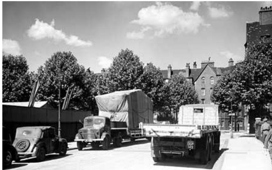
Photo 2: Sections of an AIROH Aluminum bungalow arriving at the Tate Gallery, London, 1945 (Stevenson, 2003)
