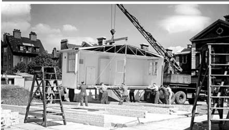
Photo 3: Sections of an AIROH Aluminum bungalow being craned into place for display at the Tate Gallery, London, 1945 (Stevenson, 2003)
