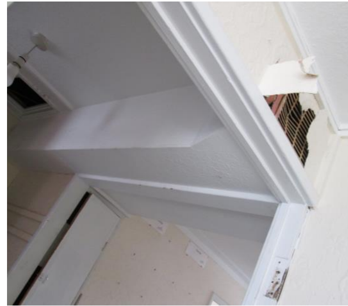
Photo 27: Block in former heating ventilation / flue between the back bedroom and hallway of 1 Pitt Street.
