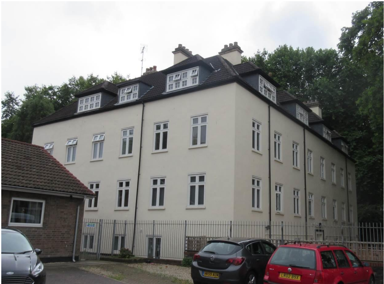
Figure 4: Former Quaker workhouse (listed Grade II), on site adjoining present meeting house
