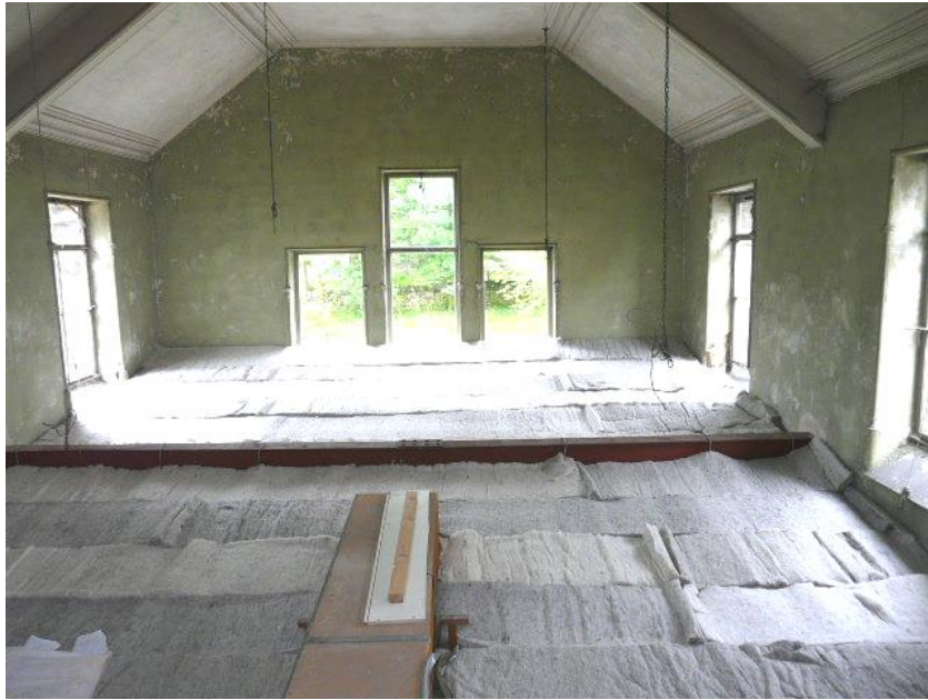
Figure 2: Upper level of the main meeting room (Brian Sawley, 2009)
