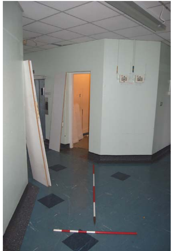
Plate 37: Widening of [1F02] to south.
