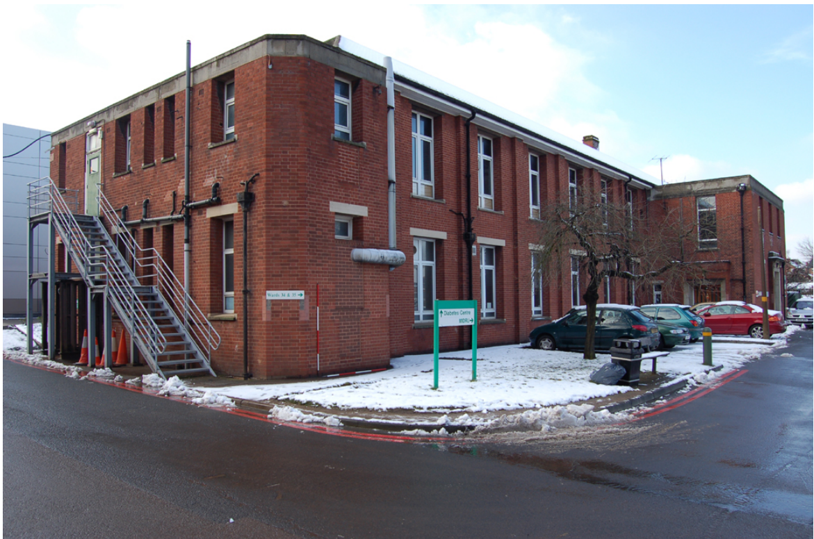
Plate 2: North elevation; oblique view looking south-west.
