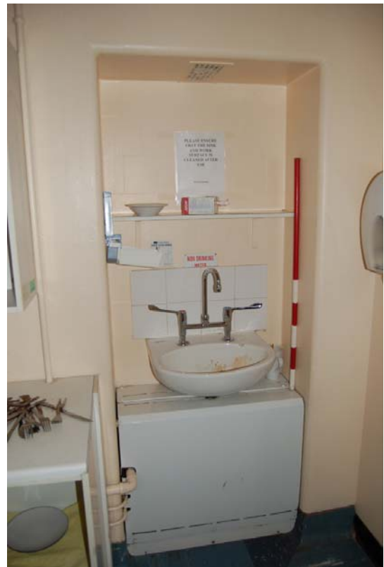
Plate 41: Recess within east wall of [1F40].
