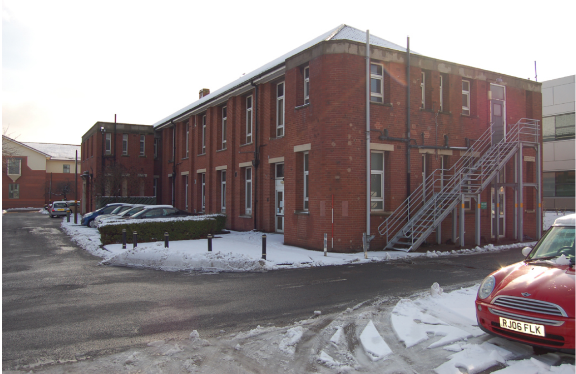
Plate 1: North elevation; oblique view looking south-east.
