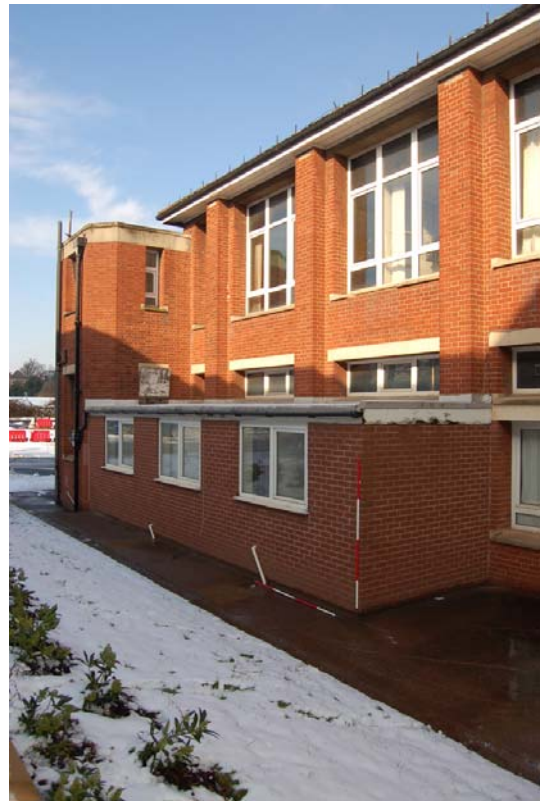
Plate 13: Secondary extension (west).
