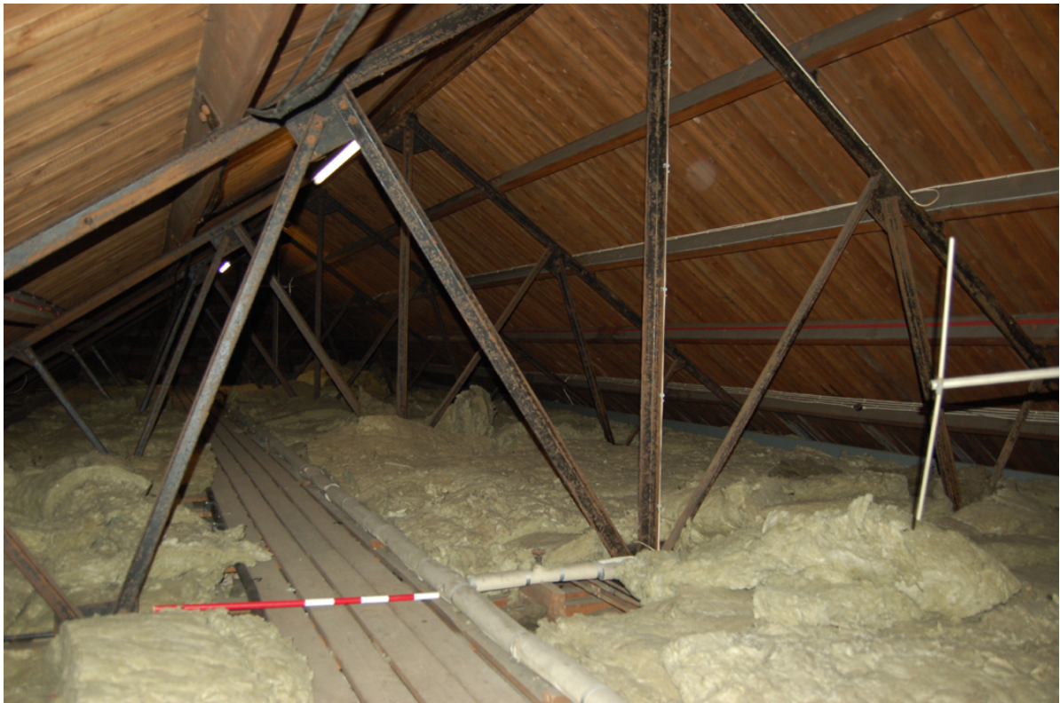
Plate 50: Roof structure over eastern section of ward block, looking east.
