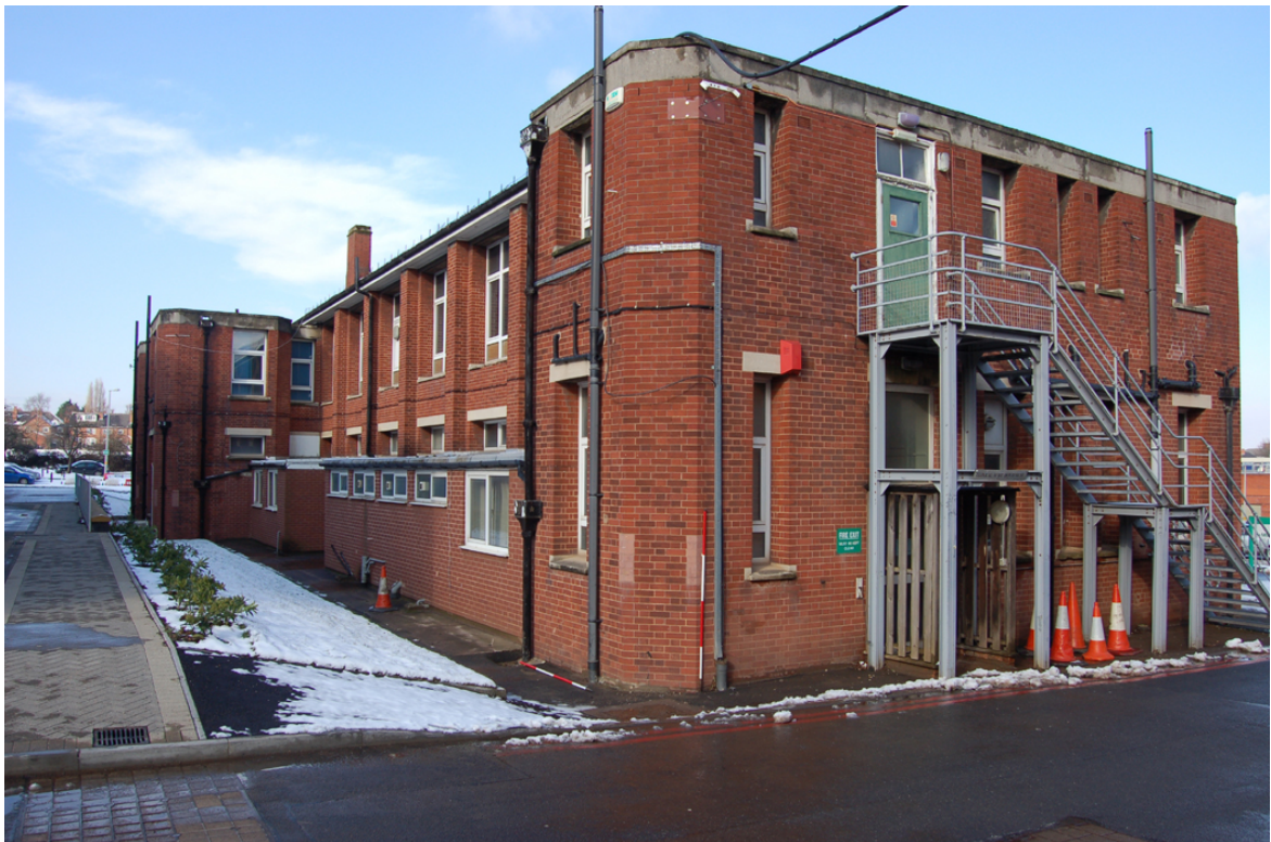
Plate 8: South elevation; oblique view looking north-west.
