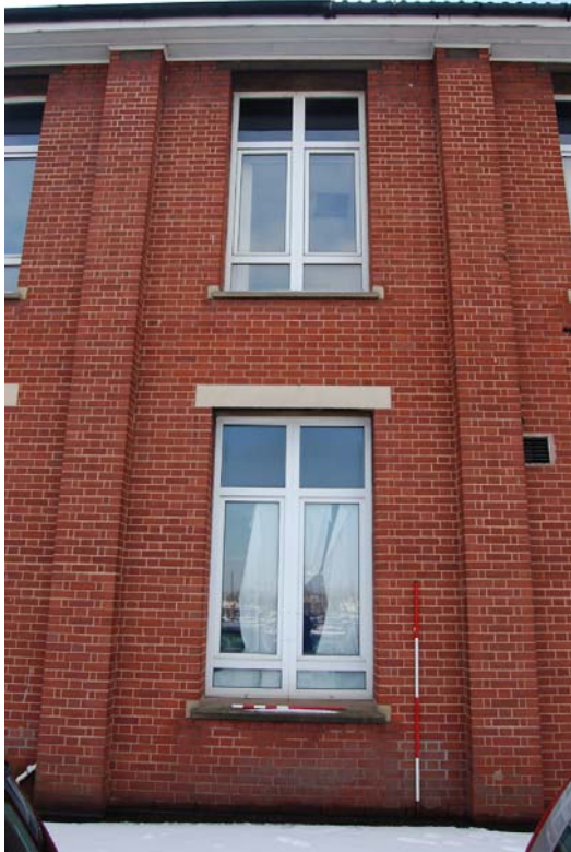
Plate 3: Sample window bay of north elev.
