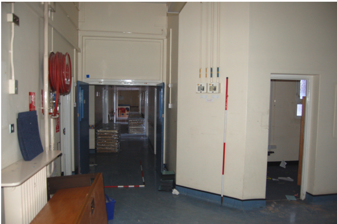
Plate 21: Widening of [GF26] to south, looking west towards corridor [GF15].
