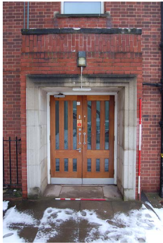
Plate 7: Doorway to 1F stair.
