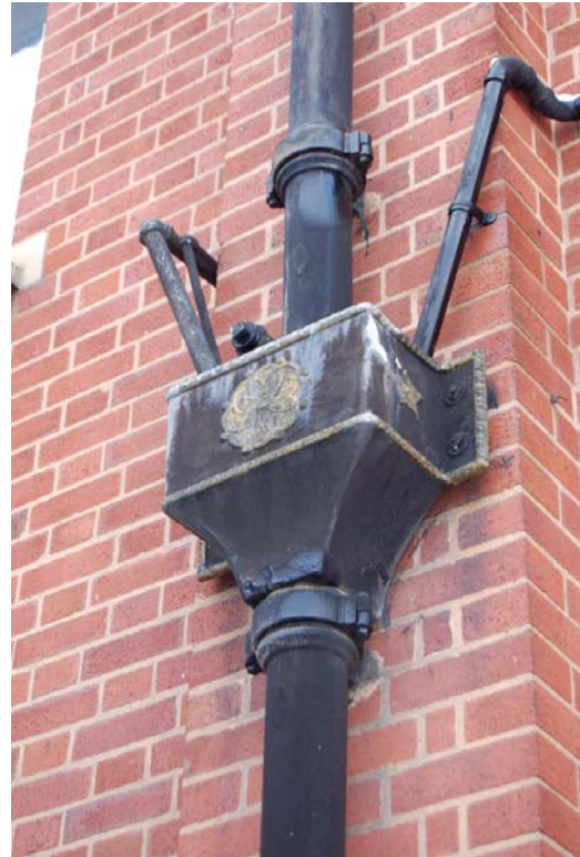
Plate 4: Rain-water hopper in north elev.
