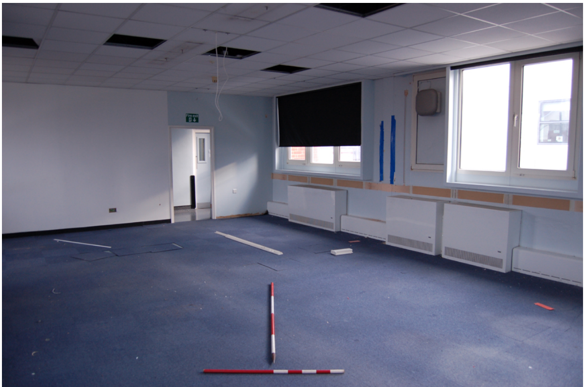
Plate 45: Room [1F13] looking south-east.
