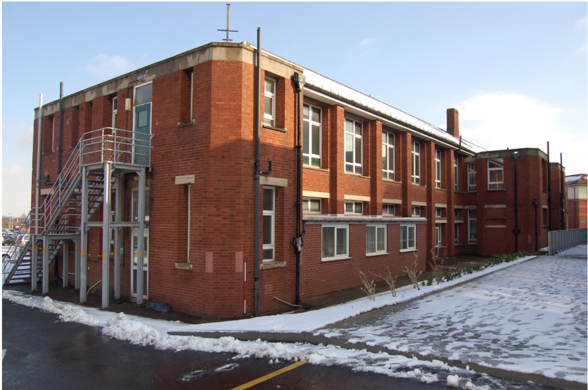
Plate 9: South elevation; oblique view looking north-east.
