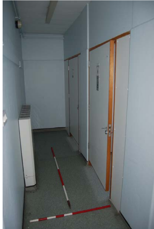
Plate 47: [1F16-18] looking north.
