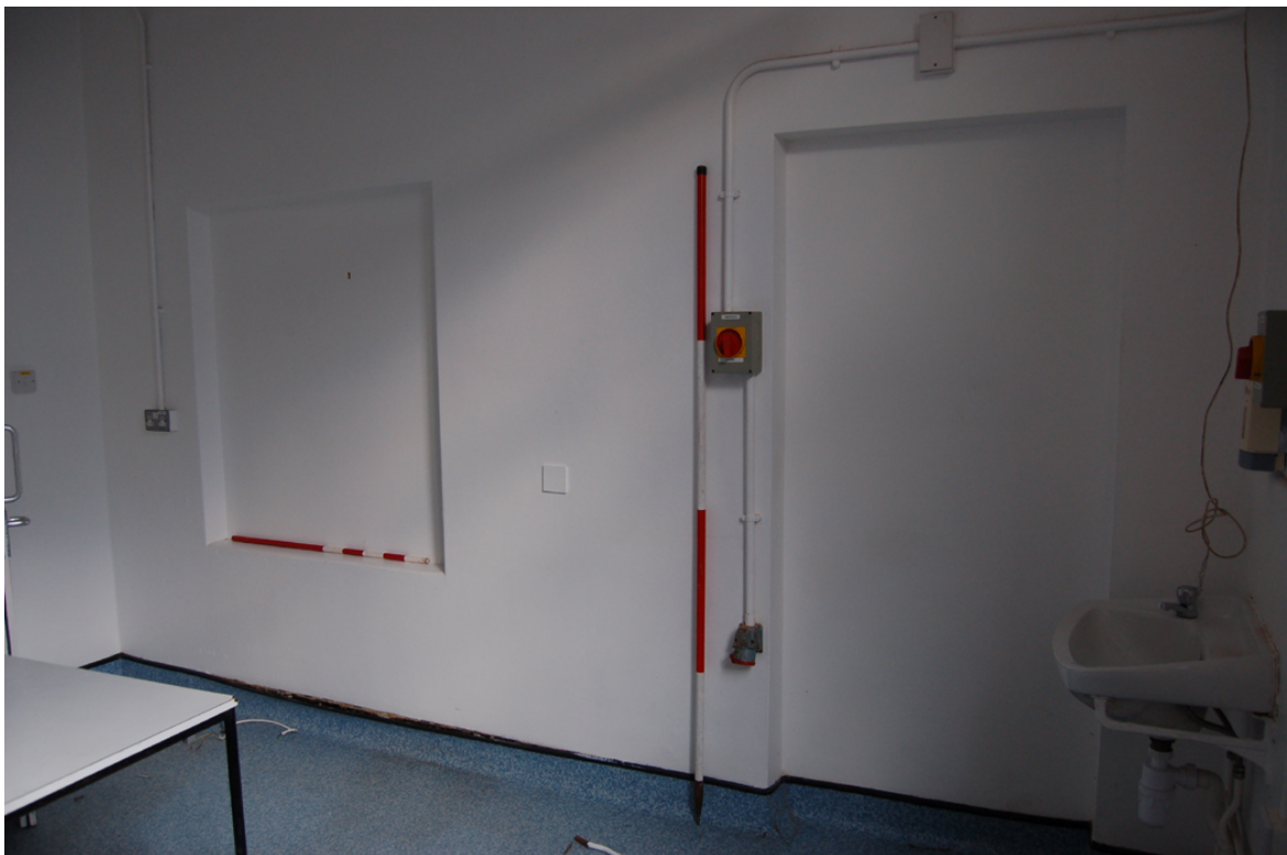
Plate 39: Corresponding blocked window and door openings within east wall of [1F05].
