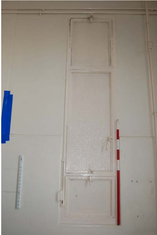
Plate 30: Surviving primary window, [GF07].
