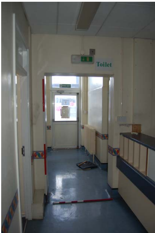
Plate 28: Doorway to [GF08].
