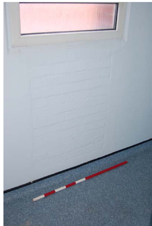
Plate 49: Blocking beneath window [1F15] (north wall).
