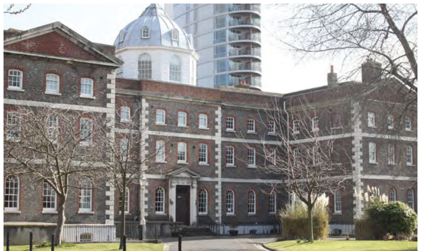
Fig. 25. Former Naval Academy at Portsmouth (1729–32, 1/14), east elevation. A. Coats 2014. Reproduced with the permission of the MoD.
