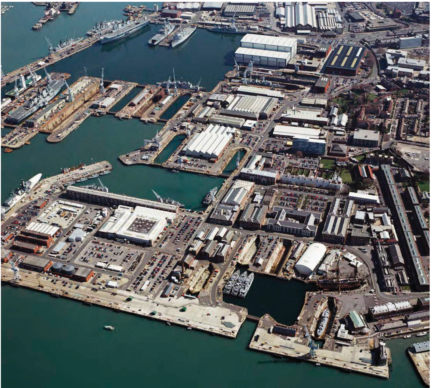
Fig. 43. 23834/01 SU 6200/31. Aerial photograph of Portsmouth's straightened Western Jetties and North Corner from the west, showing Dock No. 6 cut off from the harbour, as is Monitor HMS M33 in Dock No. 1, with HMS Victory in Dock No 2 and Mary Rose in Dock No. 3 (11 Apr 2005). ©Historic England.
