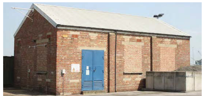
Fig. 33. Portsmouth D East Substation, built as Motor Generator House No. 18 and extended in 1950 (1939, 2/205), enhanced by a painted flagpole. A. Coats, 2013. Reproduced with the permission of the MoD.
