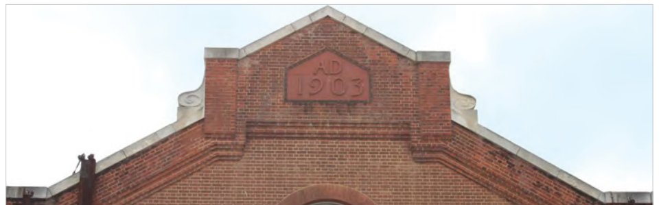
Above: Fig. 49. Date plaque 1903 on Portsmouth Factory (1903, 3/82) north elevation. Note the scrolled abutments which also support Rodney's pediment (1847–48, NE/14), the Gymnasium roof gable (1893–1900), the gable on the north elevation of Barham (1899, NE/82) and Rochefort Dockyard Ropery (1666–69). A. Coats 2013. Reproduced with the permission of the MoD.
