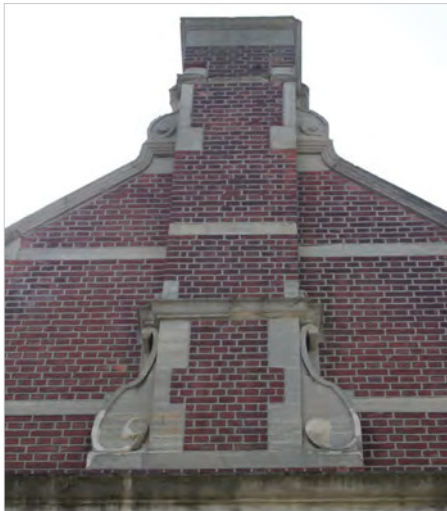
Fig. 46. Stone pediment on the east elevation of Rodney at Portsmouth (1847–48, NE/14, now Leviathan), the Warrant Officers' Mess in the former army Anglesey Barracks, incorporated in 1899 into the Naval Barracks (later HMS Nelson Barracks). It features the scrolled abutments seen at Rochefort Dockyard Ropery (1666–69), on the Gymnasium south elevation roof gable (1899), the gable on the north elevation of Barham (1899, NE/82) and the date plaque (1903) on the north elevation of the Factory (1903, 3/82). The southern section was bombed during the Second World War. A. Coats 2013. Reproduced with the permission of the MoD.
