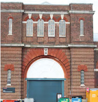
Above: Fig. 38. Concrete architrave, north elevation, Portsmouth Storehouse No. 5 (1951, 1/34). A. Coats 2013. Reproduced with the permission of the MoD.
