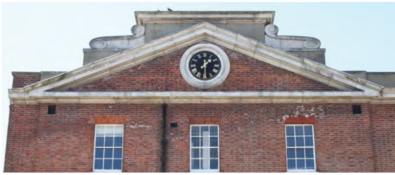
Fig. 46. Stone pediment on the east elevation of Rodney at Portsmouth (1847–48, NE/14, now Leviathan), the Warrant Officers' Mess in the former army Anglesey Barracks, incorporated in 1899 into the Naval Barracks (later HMS Nelson Barracks). It features the scrolled abutments seen at Rochefort Dockyard Ropery (1666–69), on the Gymnasium south elevation roof gable (1899), the gable on the north elevation of Barham (1899, NE/82) and the date plaque (1903) on the north elevation of the Factory (1903, 3/82). The southern section was bombed during the Second World War. A. Coats 2013. Reproduced with the permission of the MoD.
