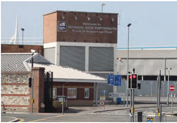
Fig. 28. Welcome message borne on the electricity substation (c.1950, 3/156) at Portsmouth Trafalgar Gate (2011). A. Coats 2013. Reproduced with the permission of the MoD.
