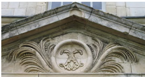
Fig. 24. Louis XIV's personal 'L' emblem at Rochefort Dockyard Ropery (1666–69). A. Coats 2008.
