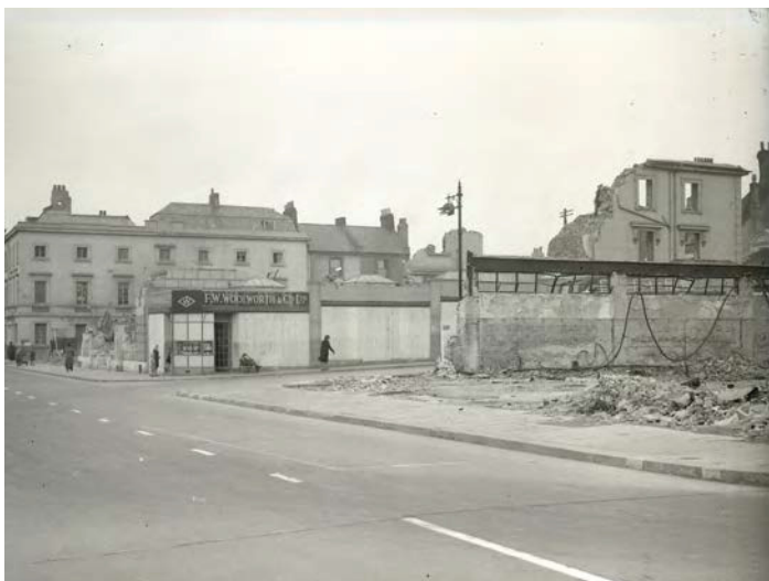
Fig. 10. Photograph Devonport, Fore Street, air raid damage, c. October 1941. PWDRO, 1418/1360. © Plymouth City Council (Arts and Heritage) / courtesy of Western Morning News Ltd.
