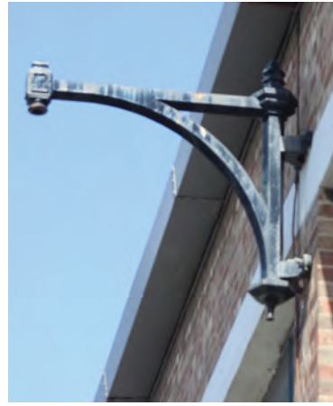
Fig. 62. Cast iron light bracket, similar to those on Portsmouth North Pumping Station (1913, 2/239) and the Gunnery Mounting Store (1896, 2/165), attached anachronistically and non-functionally to the Weapon Electrical Workshop (1936, 2/152). A. Coats, 2015. Reproduced with the permission of the MoD.
