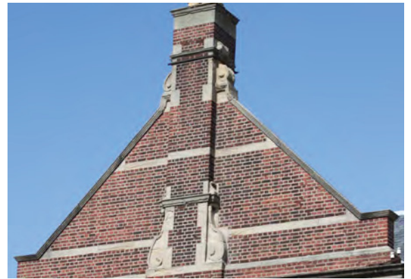
Fig. 47. Portsmouth HMS Nelson Barracks, Gymnasium (1893–1900, NE/81) south elevation roof gable. Note the scrolled abutments similar to those at Rochefort Dockyard Ropery (1666–69), which also support Rodney's pediment (1847–48, NE/14), the gable on the north elevation of nearby Barham (1899, NE/82) and the date plaque (1903) on the north elevation of the Factory (1903, 3/82). A. Coats 2013. Reproduced with the permission of the MoD.
