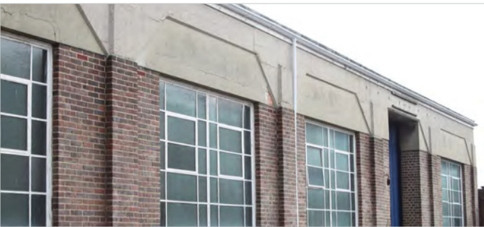
Above: Fig. 38. Concrete architrave, north elevation, Portsmouth Storehouse No. 5 (1951, 1/34). A. Coats 2013. Reproduced with the permission of the MoD.
