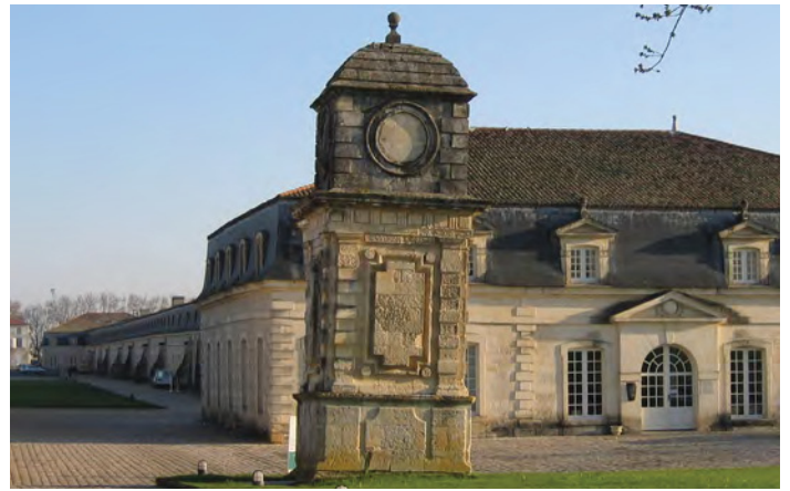
Fig. 23. Large decorative scrolled abutments at Rochefort Dockyard Ropery (1666–69). A. Coats 2008. They are also used on Rodney (1847, NE/14), the Gymnasium south elevation roof gable (1899), the gable on the north elevation of nearby Barham (1899, NE/82) in HMS Nelson Barracks, and the date plaque (1903) on the north elevation of the Factory (1903, 3/82).
