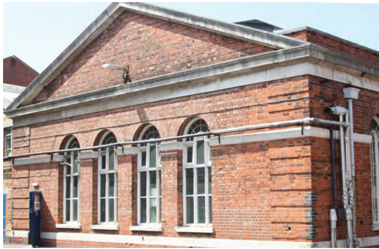
Fig. 53. Tall windows on the east elevation of Portsmouth Painters' Shop (1896, 2/191), to maximise natural light. A. Coats 2013. Reproduced with the permission of the MoD.
