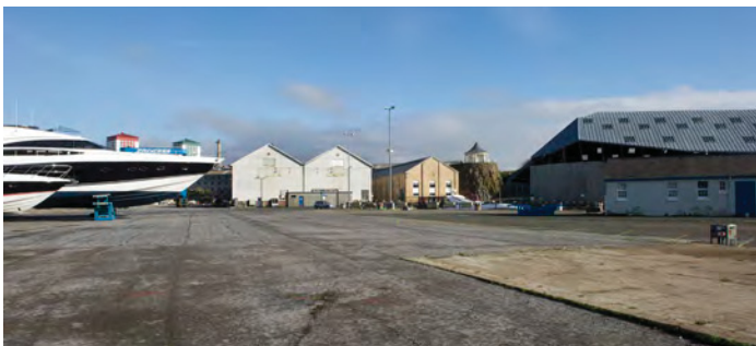
Fig. 181. DP130113. Devonport South Yard: photograph of Building S173 recorded before demolition. General view looking northeast across the dockyard towards S172 and S173 (8 Feb 2011). King's Hill Gazebo (1822, S186) and the newly roofed Covered Slip No. 1 are on the right. S173 was constructed as a Plumbers' Shop as part of the project dating from 1900 to supply the building of Dreadnoughts on nearby Slip No. 3 (English Heritage, Aug 2010, Listing Advice Report Building S173). Princess Yachts vessels are seen on the left. ©Historic England.
