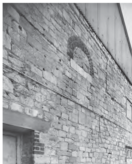
Left: Fig. 68. BB96/03859. Devonport South Yard South Smithery (S126) photograph detail of evidence of the line shaft on the north side of central building (29 Feb 1996). ©Crown copyright.HE.
