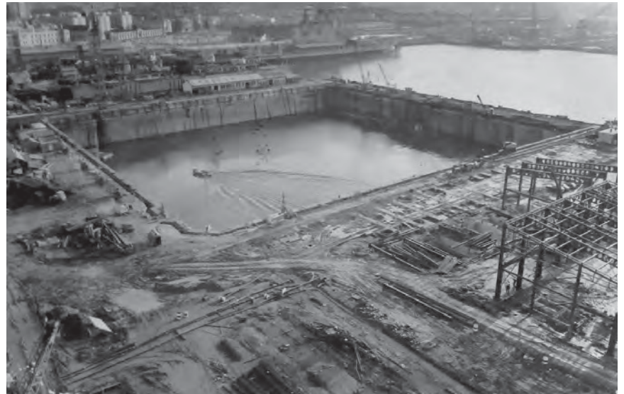
Fig. 150. Cofferdam completed. TNA, CM 20/61 (1973–74). PSA: Devonport: Works Projects. Photograph albums. Nuclear Submarine Refit Complex book no. 1. Submarine Refit Complex December 1974. Reproduced with the permission of The National Archives.
