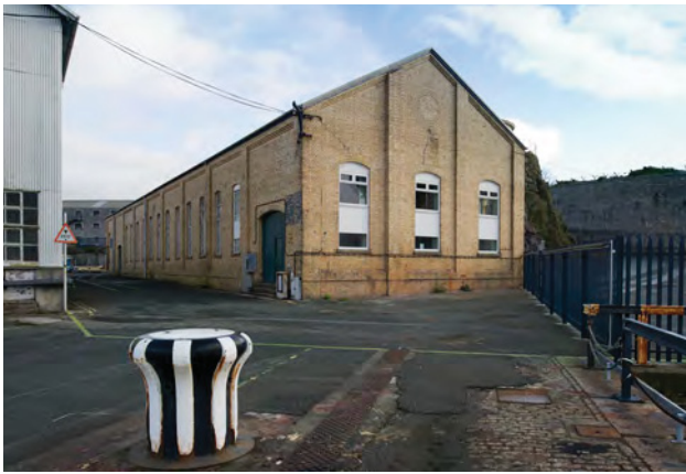
Fig. 182. DP130116. Devonport South Yard: photograph of Building S173 recorded before demolition. View of S173 looking towards the west end doorway on the west elevation (8 Feb 2011). King's Hill Gazebo (1822, S186) can just be seen behind it to the right, with new fencing to secure Princess Yachts' land. Shallow Dock is in the bottom right hand corner. ©Historic England.
