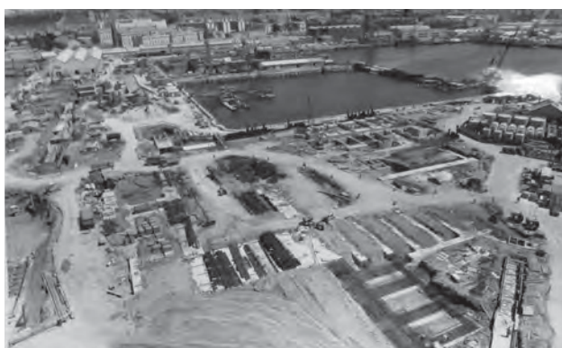
Fig. 115. Photograph albums. Fleet Maintenance Base Devonport: Foundations book no. 1 (1974). TNA, CM 20/77 (1973–74). PSA: Devonport: Works Projects. Reproduced with the permission of The National Archives.
