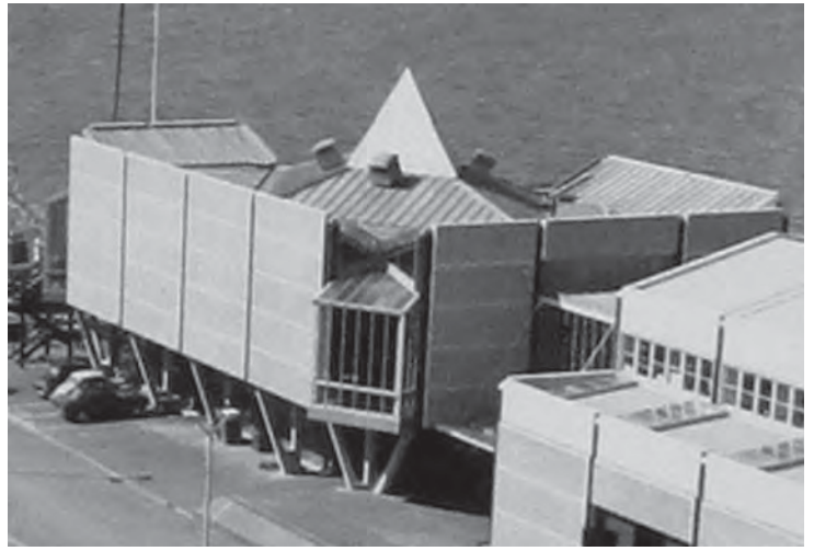
Fig. 130. NAAFI building, September 1979. Detail from Fig. 125. TNA, CM 20/80 (1976). PSA: Devonport: Works Projects. Photograph albums. Fleet Maintenance Base Devonport: book no. 4. Reproduced with the permission of The National Archives.
