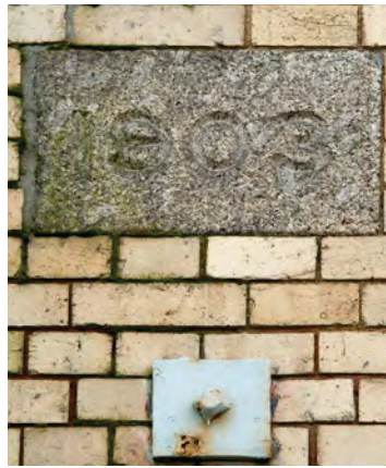
Fig. 183. DP13021. Devonport South Yard: photograph (8 Feb 2011) of Building S173 recorded before demolition. Stone dated 1903 on the west elevation. ©Historic England.
