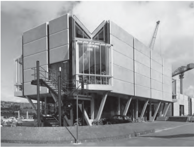
Fig. 129. NAAFI building (September 1979). TNA, CM 20/80 (1976). PSA: Devonport: Works Projects. Photograph albums. Fleet Maintenance Base Devonport: book no. 4. Reproduced with the permission of The National Archives.
