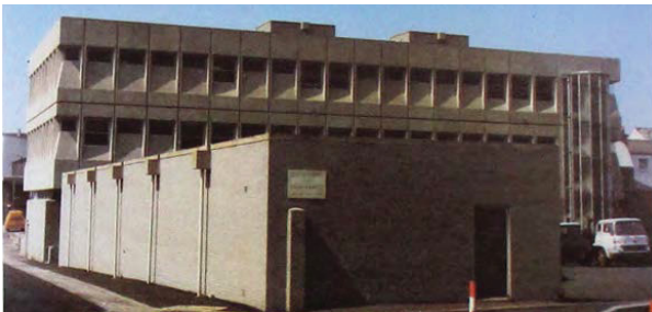
Fig. 142. External Planning Guide by Joint PSA and MOD Planning Team: a study of spaces around and between buildings. TNA, CM 20/55 (1976). PSA: Devonport: Publication and Research Studies. Reproduced with the permission of The National Archives.
