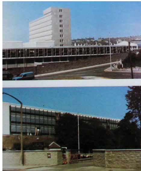
Fig. 141. External Planning Guide by Joint PSA and MoD Planning Team: a study of spaces around and between buildings. TNA, CM 20/55 (1976). PSA: Devonport: Publication and Research Studies. Reproduced with the permission of The National Archives.
