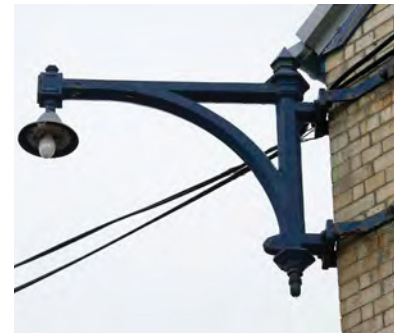
Fig. 184. DP13023. Devonport South Yard: photograph of Building S173 recorded before demolition. Cast iron lamp bracket on the southwest corner of S173 (8 Feb 2011). ©Historic England.
