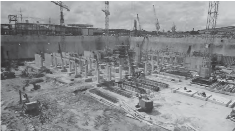
Fig. 151. Submarine Refit Complex (May 1975). TNA, CM 20/62 (1975). PSA: Devonport: Works Projects. Photograph albums. Nuclear Submarine Refit Complex book no. 2. Reproduced with the permission of The National Archives.
