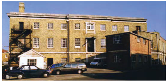
Fig. 265. Portsmouth Boathouse No. 6. Photograph of the south elevation. PNBPT Record Photograph no. E02 (June 1998). Reproduced with the kind permission of Portsmouth Naval Base Property Trust.
