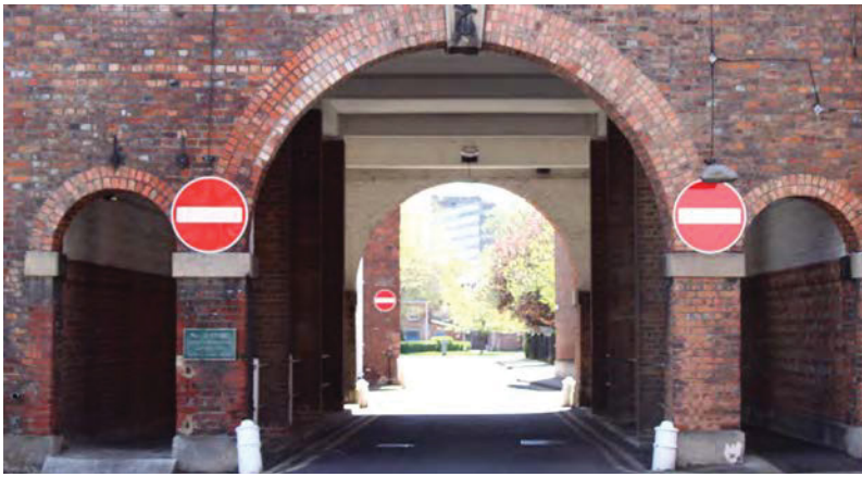
Fig. 319. Arches cut through the former Portsmouth Great Ropehouse (1771, 1/65), north elevation, when it ceased making rope in 1868. A. Coats 2013. Reproduced with the permission of the MoD.
