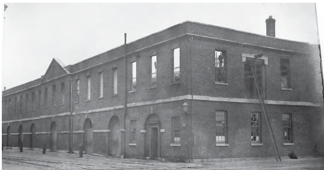
Fig. 357. Storehouse No. 33 before reconstruction after fire 23.3.1908, photograph no. 99. TNA, ADM 195/79 (1857–1915). 100 photographs depicting: construction works at Portsmouth Dockyard. Reproduced with the permission of The National Archives.
