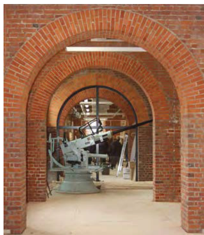
Above: Fig. 312. Ground floor of Portsmouth Storehouse No. 10 (1776, 1/59) looking south along the eastern bay, showing renewed brickwork and timber pillars and beams during its refurbishment for the twentieth century Babcock Galleries (2014) A. Coats 2013. Reproduced by kind permission of the Trustees of the National Museum of the Royal Navy.
