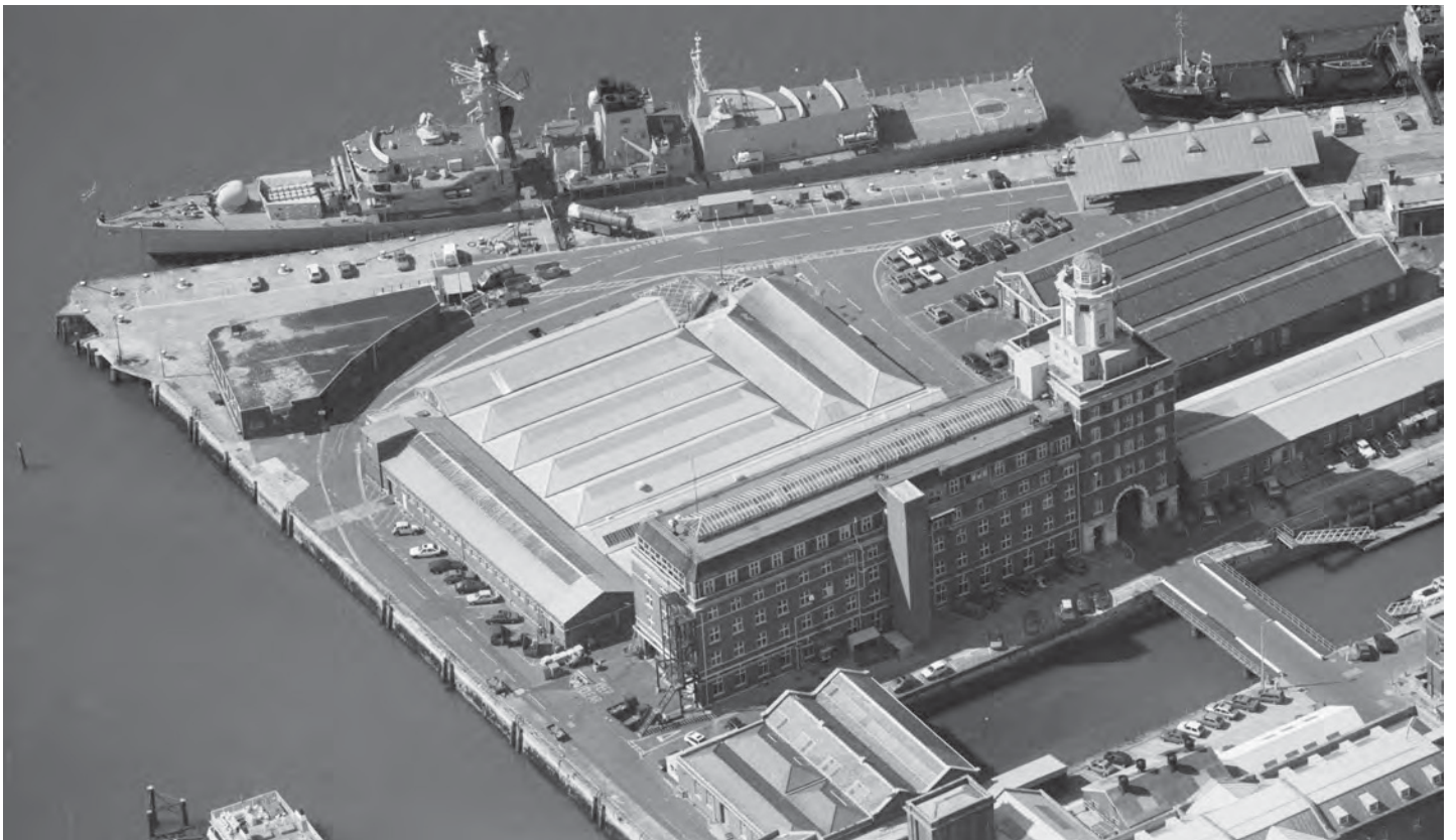
Fig. 290. 15800/33 SU 6200/17. Aerial photograph of the Semaphore Tower and Rigging House from the east. (9 Sept 1997). ©Crown copyright.HE.
