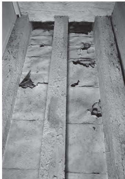
Fig. 310. J360/06/72. Photograph of Storehouse Nos 9, 10, 11: Mr Hartley's fire plates on first floor joists and floorboards (c.1971). ©Crown copyright.HE.
