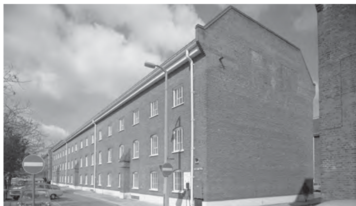
Fig. 318. J188/03/71. Photograph of Storehouse Nos 15, 16 and 17 (28 Apr 1971) from the east, showing 'GR 1771' inserted in darker bricks on the east elevation of Storehouse No. 16. ©Crown copyright.HE.
