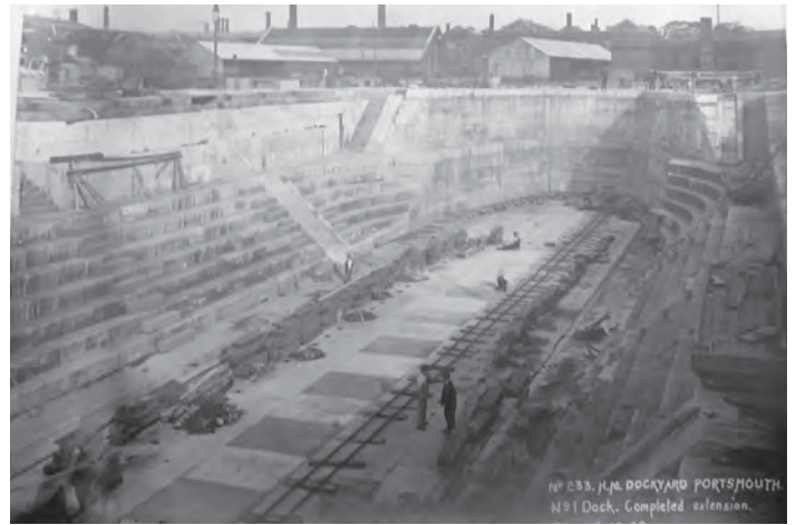
Fig. 335. Dock No. 1 (6.1.1909). Photograph of completed extension, looking northeast. TNA, ADM 195/79 (1857–1915). 100 photographs depicting construction works at Portsmouth Dockyard. Reproduced with the permission of The National Archives.
