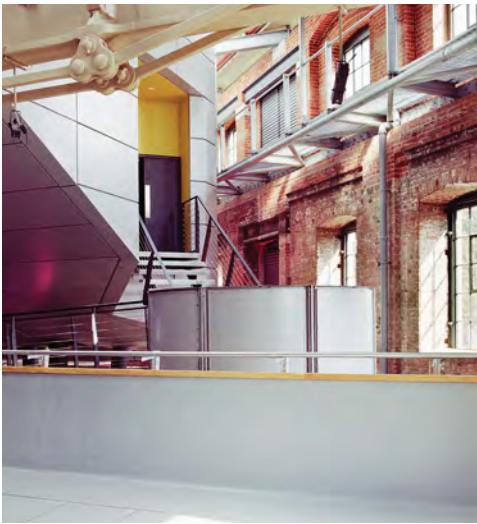
Fig. 275. AA026355. Photograph of the eastern interior of Portsmouth Boathouse No. 6 showing the cinema structure inserted within the area damaged by a bomb in the Second World War (2001). ©Historic England.
