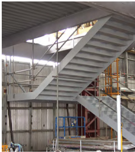
Fig. 242. Interior of the corrugated steel wall forming the south elevation of Portsmouth Boathouse No. 4 (1940, 1/6), showing the newly constructed stairway and mezzanine floor. A. Coats 2015. Reproduced with the kind permission of Portsmouth Naval Base Property Trust.
