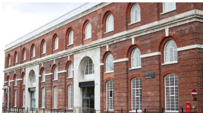
Fig. 356. West elevation of the refurbished Portsmouth Iron and Brass Foundry (1854, 1/140), now BAES HQ. A. Coats 2012. Reproduced with the permission of the MoD.
