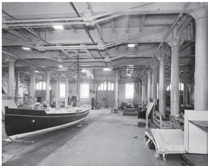
Fig. 261. BB012875. Photograph of the ground floor interior of Portsmouth Boathouse No. 6 from the northeast, before refurbishment in 2001 (11 Jun 1991). ©Crown copyright.HE.
