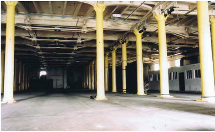
Fig. 264. Portsmouth Boathouse No. 6. Photograph of the ground floor, looking east showing the cast iron pillars and trusses. PNBPT Record Photograph no. G41 (June 1998). Reproduced with the kind permission of Portsmouth Naval Base Property Trust.
