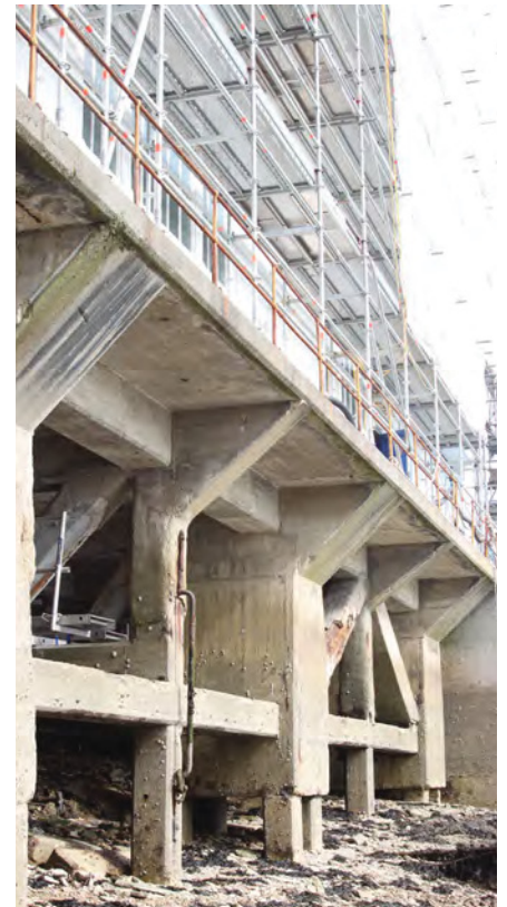
Fig. 232. West elevation of the undercroft of Portsmouth Boathouse No. 4 (1940, 1/6) at low tide, showing its beams and trusses. A. Coats 2015. Reproduced with the kind permission of Portsmouth Naval Base Property Trust.
