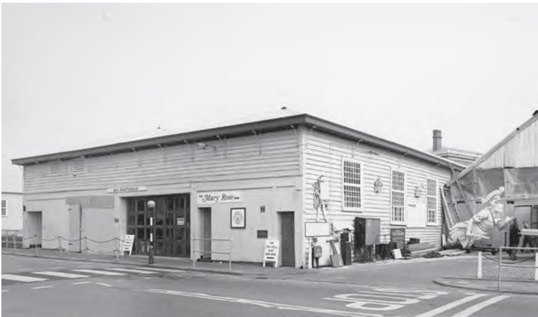
Fig. 276. PK318/11 FL00982.02.001. Photograph of the conversion of Boathouse No. 5 (1/28) and the Sail Loft (1/27) into the Mary Rose Museum (8 Mar 1984). ©Crown copyright.HE.
