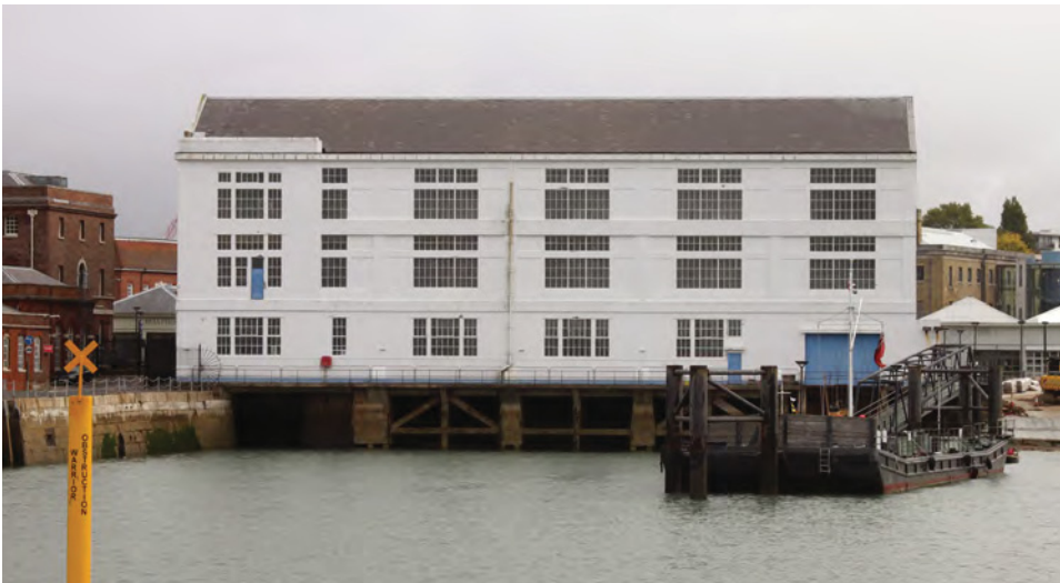
Fig. 230. West (harbour) elevation of Portsmouth Boathouse No. 4 (1940, 1/6). A. Coats 2015. Reproduced with the kind permission of Portsmouth Naval Base Property Trust.
