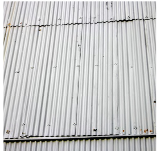
Fig. 243. Exterior of the corrugated steel wall forming the south elevation of Portsmouth Boathouse No. 4 (1940, 1/6). A. Coats 2015. Reproduced with the kind permission of Portsmouth Naval Base Property Trust.
