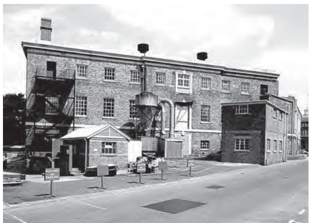
Fig. 259. Pre-1985 photograph of Boathouse No. 6. Courtesy of Portsmouth Royal Dockyard Historical Trust.
