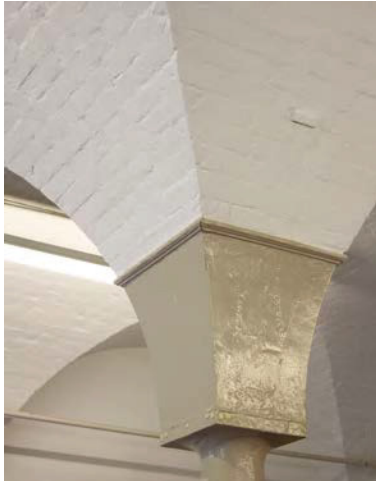
Fig. 255. Interior of Portsmouth Pay Office (1808, 1/11), showing the cast iron bases to the vaulted brick ceiling columns. A. Coats 2012. Reproduced with the kind permission of Portsmouth Naval Base Property Trust.
