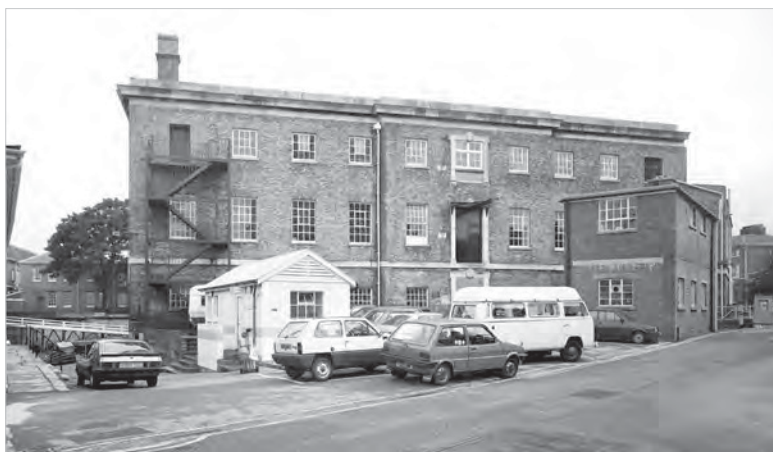
Fig. 260. BB012872. Photograph of Portsmouth Boathouse No. 6 from the southwest before refurbishment in 2001 (11 Jun 1991). ©Crown copyright.HE.
