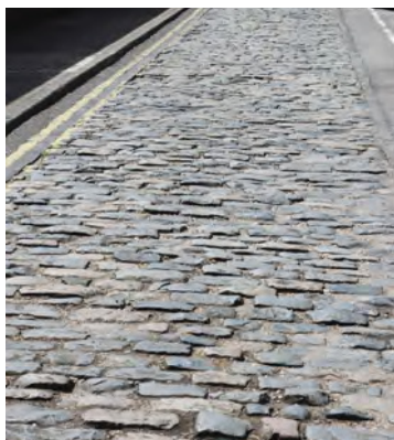
Fig. 330. In Portsmouth Admiral's Walk, a seven foot wide section of setts running along the north side of 1/81 (c.1850–90). A. Coats 2013. Reproduced with the permission of the MoD.
