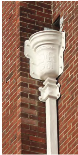
Fig. 328. Rainwater hopper dated 1961, west elevation of Portsmouth Fleet Headquarters, Jago Road (1961, 1/80). A. Coats 2014. Reproduced with the permission of the MoD.
