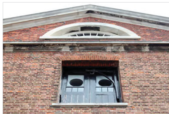
Fig. 316. A refurbished rear pediment of Portsmouth Storehouse No. 10 (1776, 1/59), showing the access doors to the upper floor and cast iron bracket (2014). A. Coats 2014. Reproduced by kind permission of the Trustees of the National Museum of the Royal Navy.
