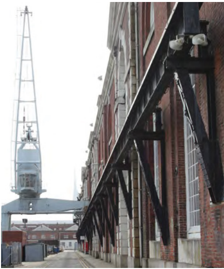
Fig. 376. Portsmouth Steam Factory (1847, 1/208), east elevation, showing the 10 ton gantry crane. A. Coats 2013. Reproduced with the permission of the MoD.
