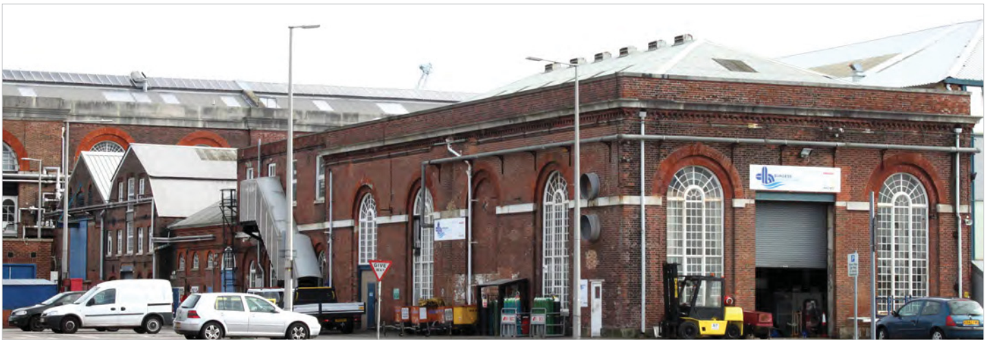
Fig. 379. Former 80hp Portsmouth Engine House (1849, 1/209) from the northeast, with the Steam Factory in the background. A. Coats 2014. Reproduced with the permission of the MoD.
