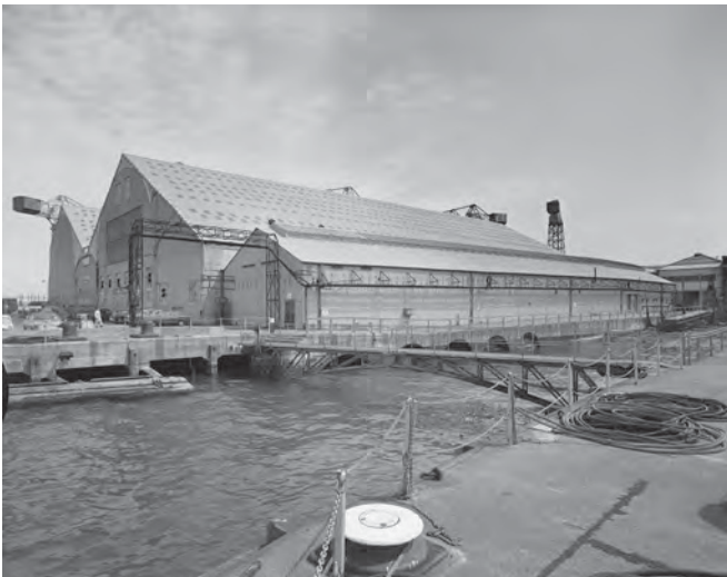
Fig. 368. J297/06. Photograph of Ship Shop Nos 3-4, south of Slip No. 5, before their demolition in 1980 (23 June 1971). ©Crown copyright.HE.
