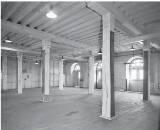
Fig. 309. J186/06/71. Photograph of Storehouse No. 9, 10 or 11 (28 Apr 1971). ©Crown copyright.HE. It is hoped that the particular storehouse can be identified.
