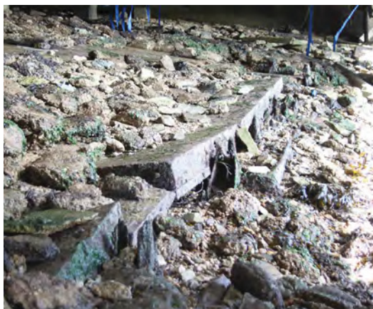
Fig. 235. Lowest level of the eighteenth century Portland Stone slipway stones, held in place by a line of wooden posts, visible beneath a layer of solidified bags of concrete, below Portsmouth Boathouse No. 4 (1940, 1/6). A. Coats 2015. Reproduced with the kind permission of Portsmouth Naval Base Property Trust.
