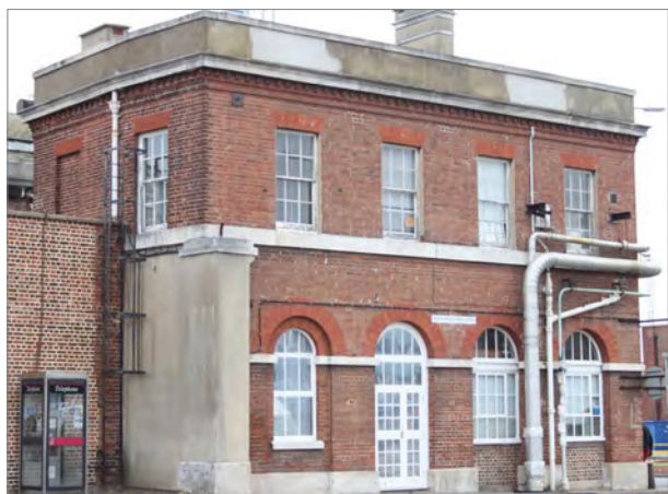
Fig. 352. Former Portsmouth Chief Inspector's Office (1857, 1/138) at the western side of the first Marlborough Gate, adjoining the original Dockyard Wall (1711). A. Coats 2013. Reproduced with the permission of the MoD.
