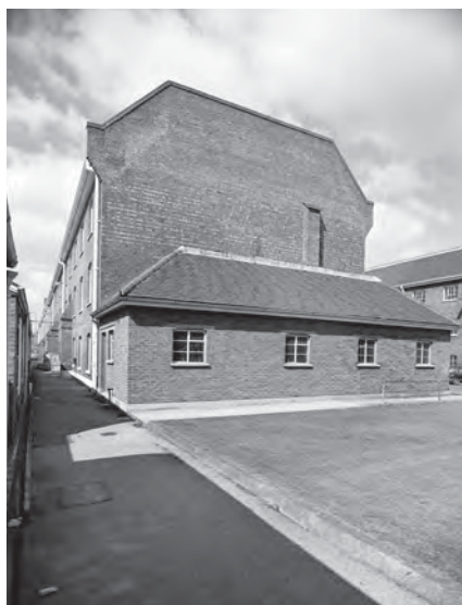
Fig. 317. J188/01/71. Photograph of Storehouse Nos 15, 16 and 17 (28 Apr 1971) from the west, showing the former site of Storehouse No. 14 or West Sea Store (1771), which suffered a direct hit on 24 August 1940. ©Crown copyright.HE.
