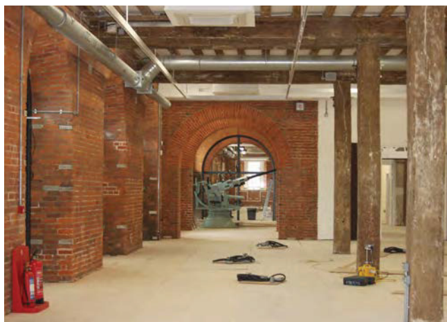
Above: Fig. 312. Ground floor of Portsmouth Storehouse No. 10 (1776, 1/59) looking south along the eastern bay, showing renewed brickwork and timber pillars and beams during its refurbishment for the twentieth century Babcock Galleries (2014) A. Coats 2013. Reproduced by kind permission of the Trustees of the National Museum of the Royal Navy.
