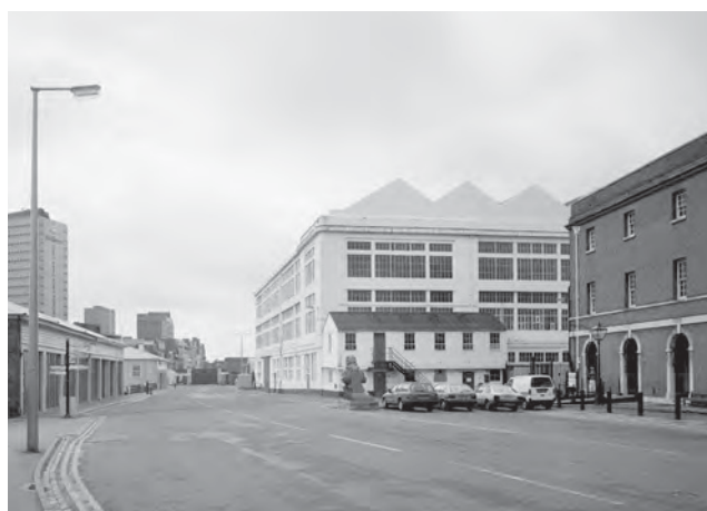
Fig. 250. BB97/012856. Photograph of the northwest corner of Portsmouth Boathouse No. 4 with Boathouse No. 4 Annex on the north side (28 Jul 1997). ©Crown copyright.HE.
