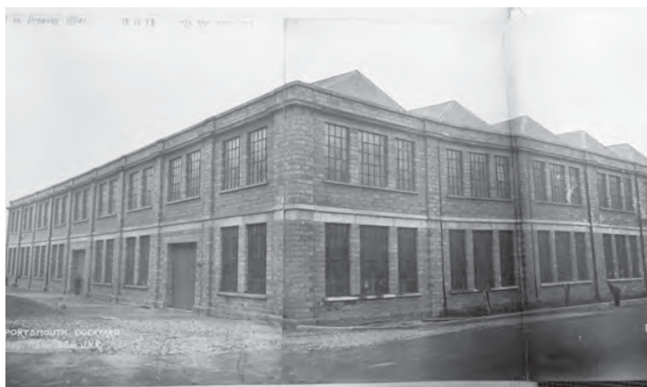
Fig. 340. Portsmouth Joiners Shop 3.2.1911. TNA, ADM 195/79 (1857–1915). 100 photographs depicting: construction works at Portsmouth Dockyard. Reproduced with the permission of The National Archives.
