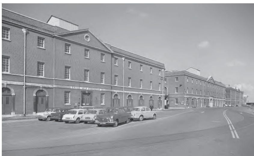
Fig. 302. J186/01/71. Photograph of the west elevations of Storehouse Nos 9, 10 and 11 (28 Apr 1971). ©Crown copyright.HE.
