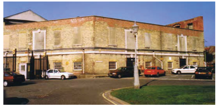
Right: Fig. 266. Portsmouth Boathouse No. 6. Photograph of the east end, south and east elevations, showing the missing roof after the air raid. PNBPT Record Photograph no. E07 (June 1998). Reproduced with the kind permission of Portsmouth Naval Base Property Trust.
