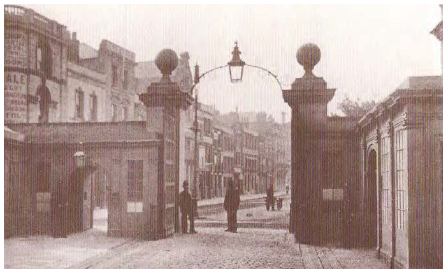
Fig. 204. Photograph of the north elevation of the Main (now Victory) Gate in 1895, showing its original width. Courtesy of Portsmouth Royal Dockyard Historical Trust.
