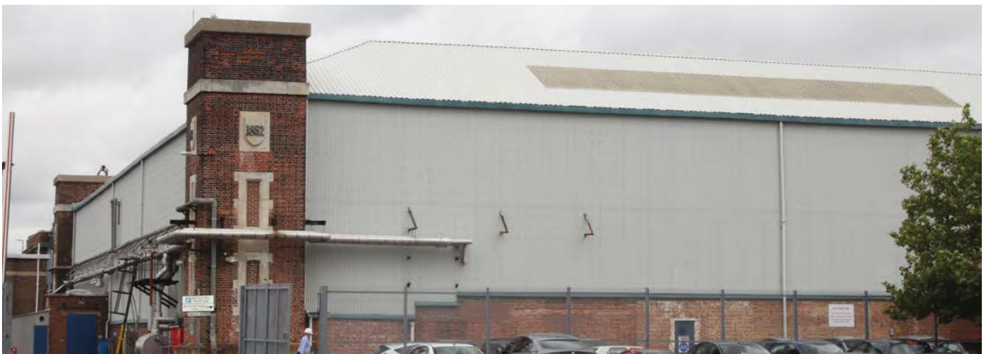
Fig. 380. Former Portsmouth Smithery (1852, 1/209), south and west elevations, showing the original western chimney bases dated 1852. A. Coats 2014. Reproduced with the permission of the MoD.
