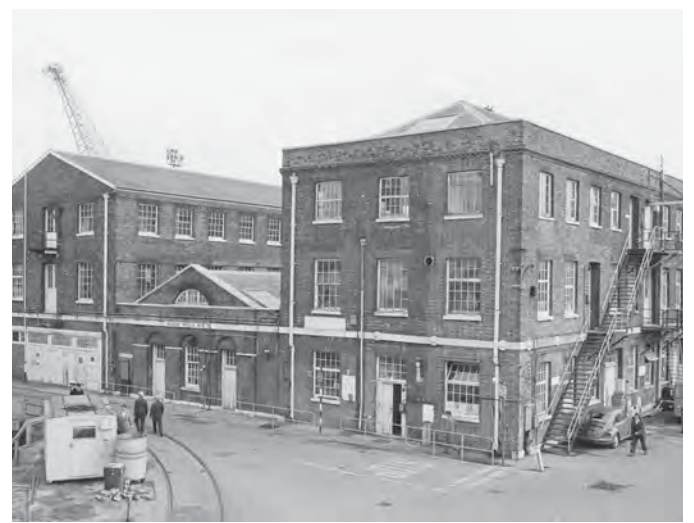
Fig. 371. PK318/07 FL00982.02.002. Photograph of the Block Mills from the southwest with the head of Dock No. 6 on the left (n.d. c.1970s). ©Crown copyright.HE.
