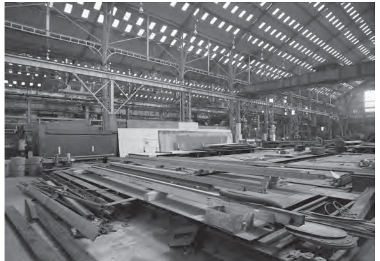
Fig. 369. J297/11. Photograph of the interior of Ship Shop Nos 3-4 before their demolition in 1980 (23 June 1971). ©Crown copyright.HE.
