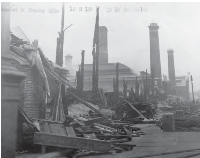
Fig. 360. Damage to Portsmouth No. 1 Slip Jetty looking east, 1.2.1915, with the Smithery and the Steam Factory in the background. TNA, ADM 195/79 (1857–1915). 100 photographs depicting: construction works at Portsmouth Dockyard. Reproduced with the permission of The National Archives.
