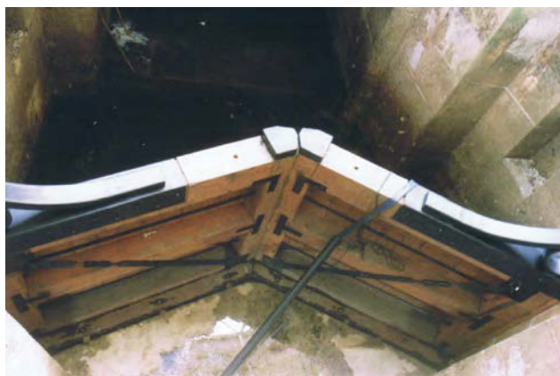
Fig. 246. Photograph of Portsmouth Boathouse No. 4 tunnel: west opening, view south, ready for pintles (PNBPT, 22.9.1999 no. 38). Reproduced with the kind permission of Portsmouth Naval Base Property Trust.
