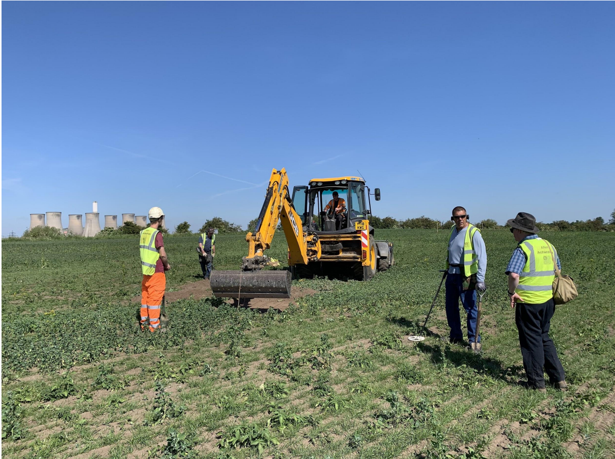
Commencing removal of topsoil, with metal detector survey
