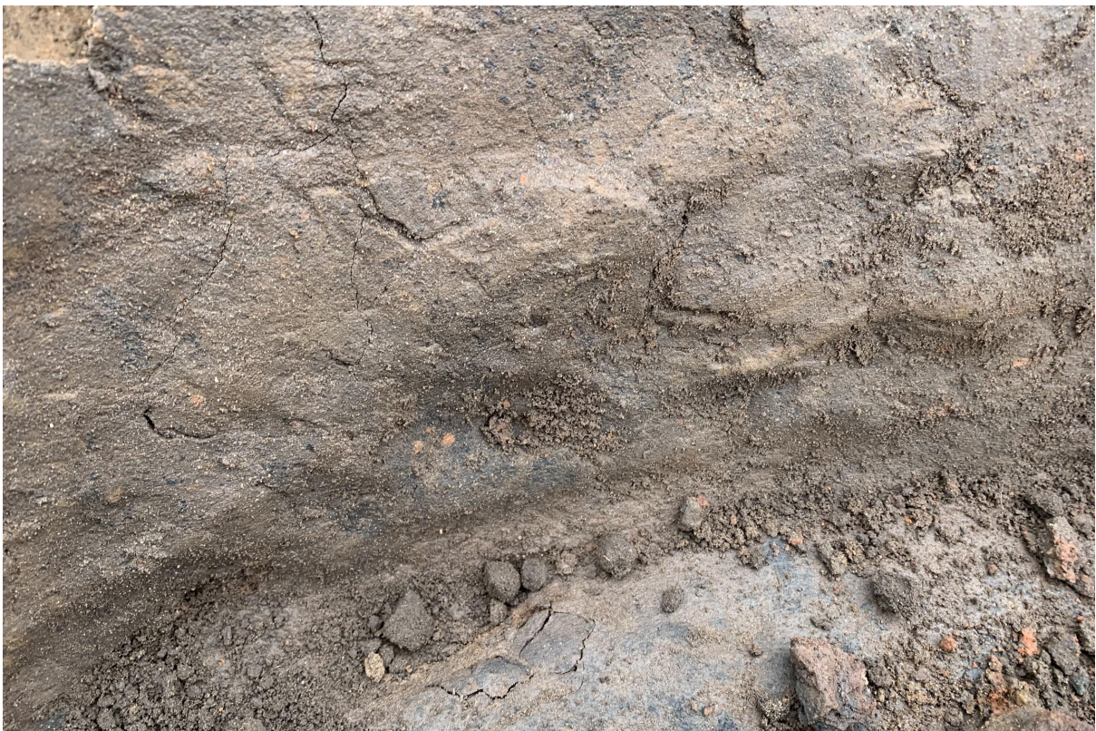
Kiln wall showing that it was built from hand-pressed slabs of clay
