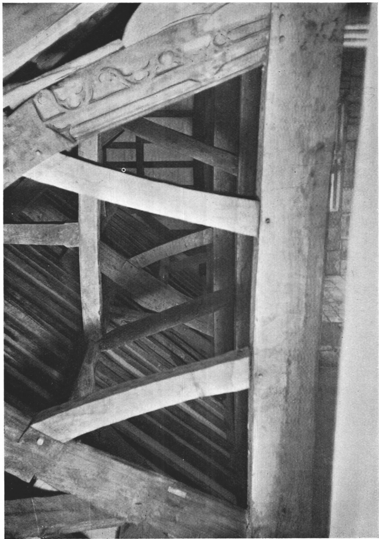
Bridge Chapel: Interior showing roof-timbers after restoration.
