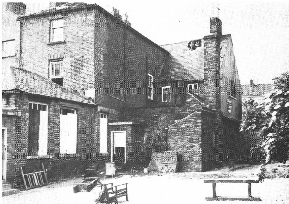
1 (b) The Peacock Inn from the south: 19th century wing, outbuildings and rear of Bay 2.
