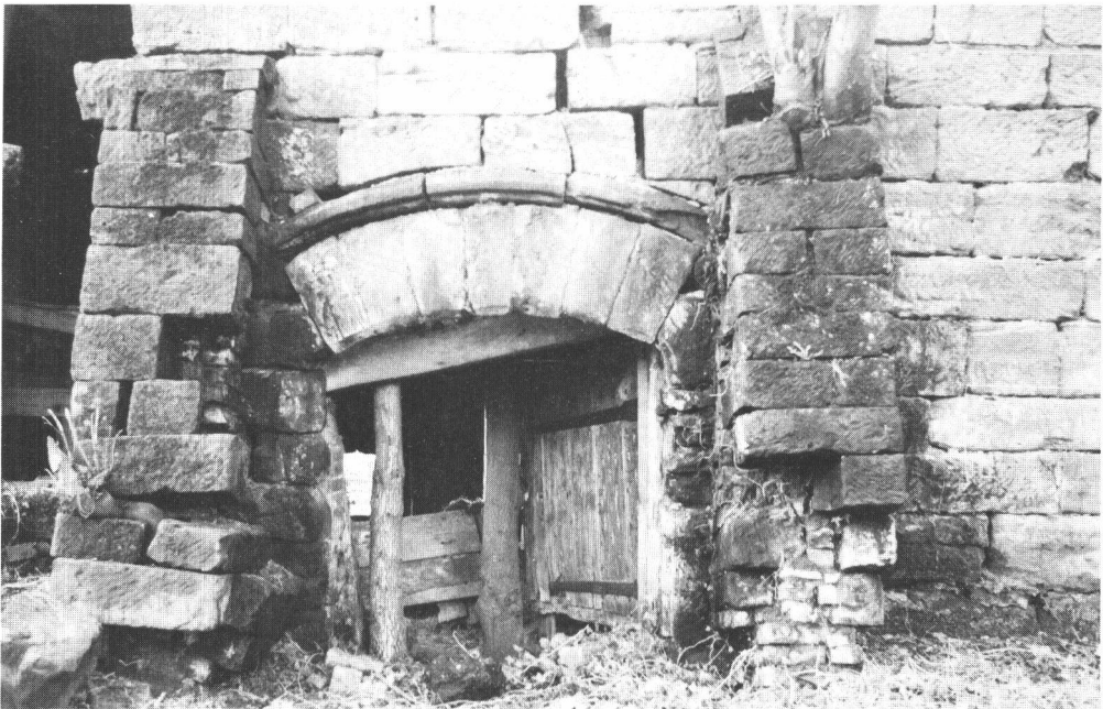
Plate 5 Norbury Mill: east door.
