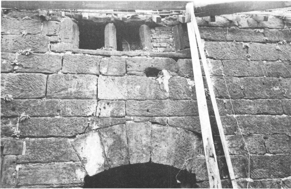
Plate 4 Norbury Mill: west elevation — detail. (Note the head of the west door and the common rafters trenched into the head of the wall and the first floor window.)
