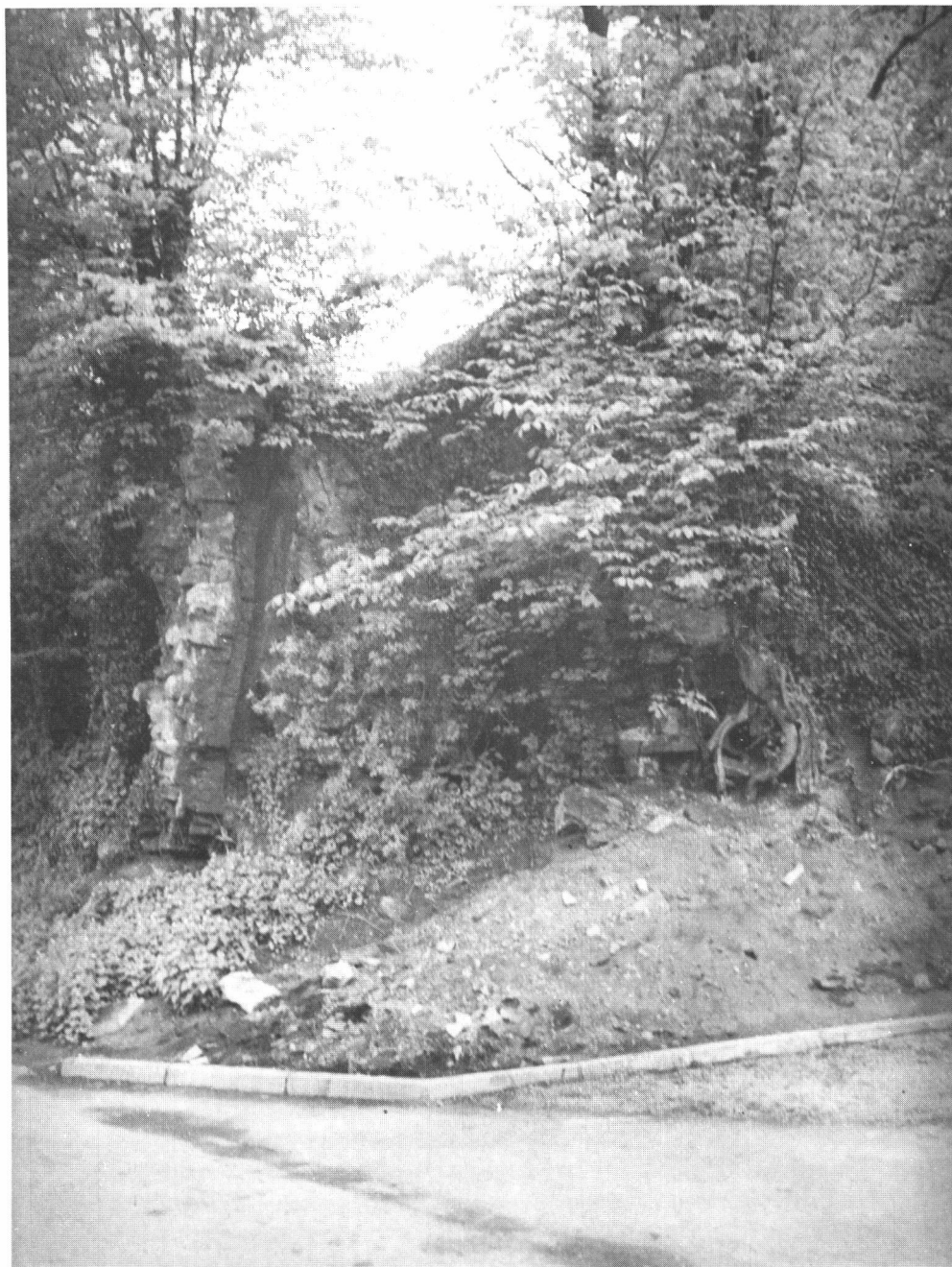
Plate 1 The remains of the blast furnace at Alderwasley, probably photographed about 1962. The view is from the NE and shows the lining of the shaft and the uncoursed rubble core of the shaft, built against the natural bank which runs down the western side of the works at Alderwasley. ( Courtesy Derby Industrial Museum; from the collection of the late Frank Nixon )
