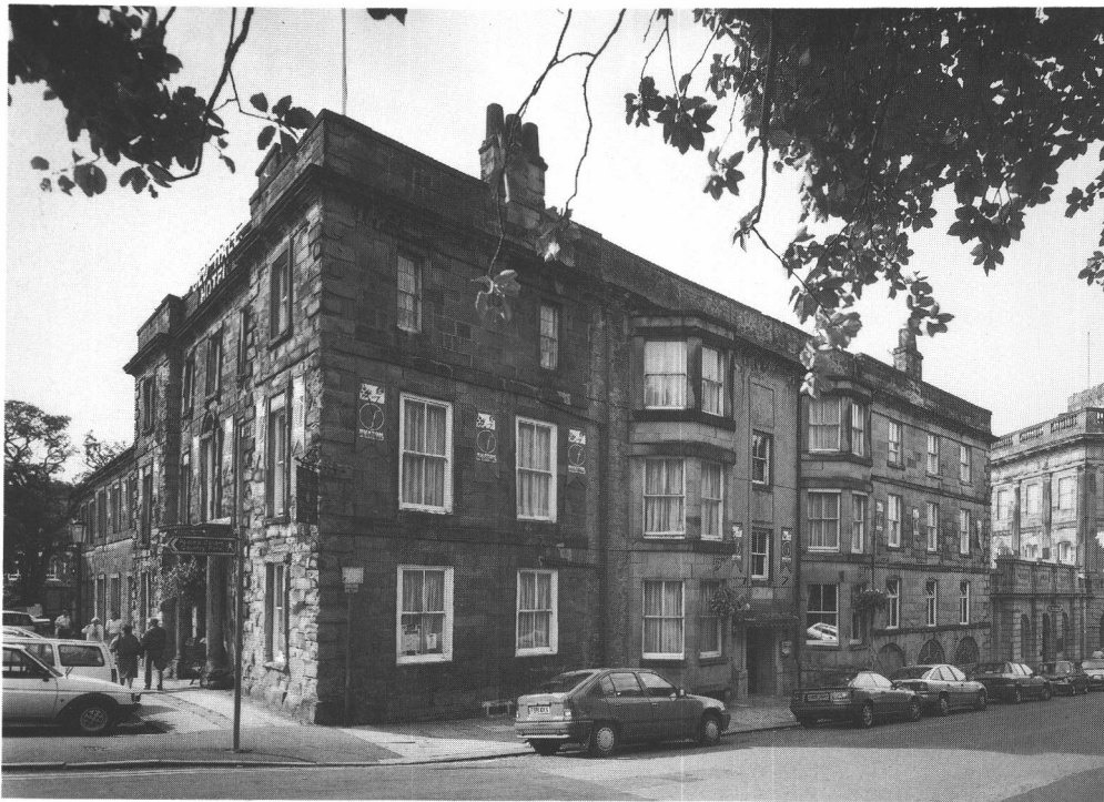
Plate 6 The south-east angle of the Hall, showing the earlier eighteenth century two bay addition to the front with the New Hall (now with canted bay windows) behind. Adjoining the New Hall to the north is a three bay extension built at the end of the eighteenth century over the former hot baths.
