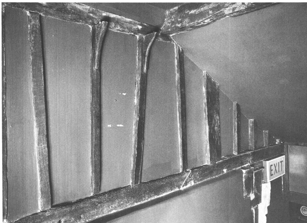
Plate 8 Surviving timber-framed partition adjacent to the staircase on the ground floor
