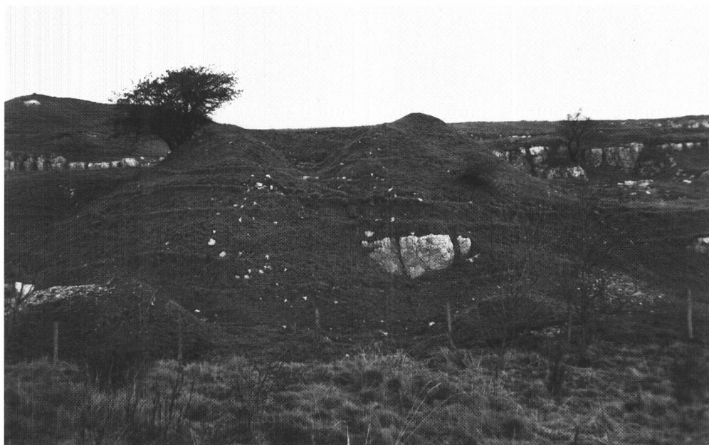
Plate 2 Large (running) 'pudding pie' kiln on Grin Hill. The kiln is approx 30ft high and the grirstone lining can just be seen. Marked 'D' on Fig 2 it probably dates from c1807-37. (Author's Collection)
