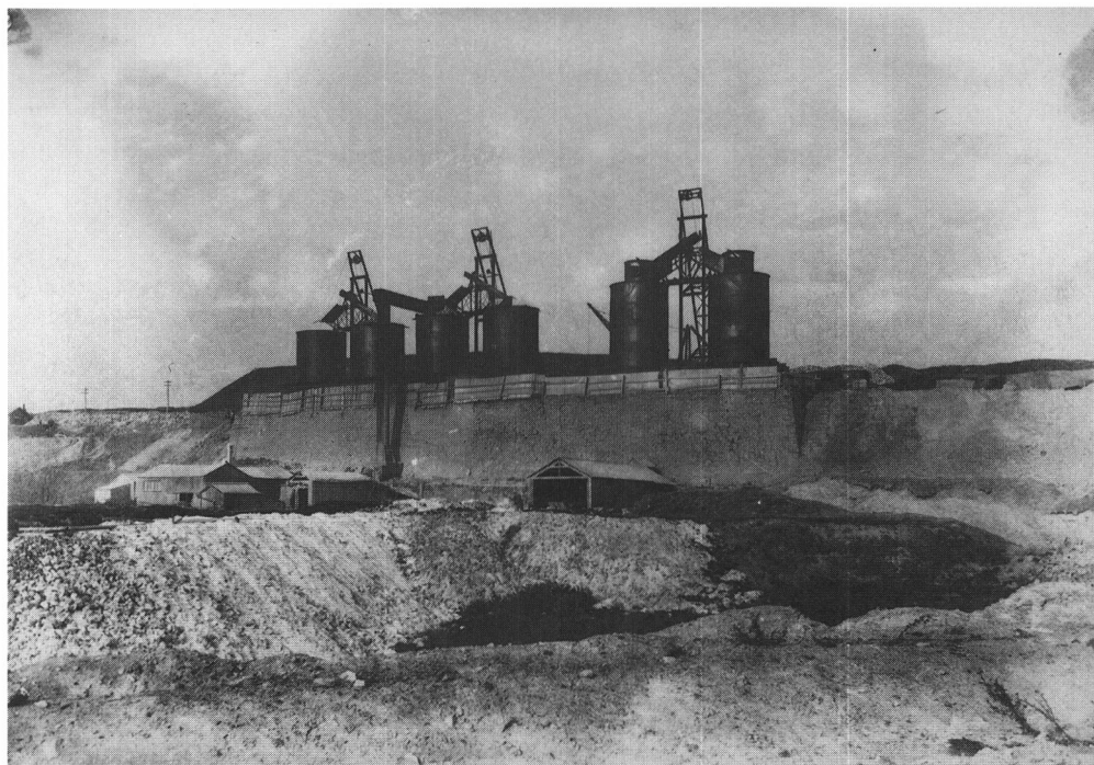
Plate 3 Masonry kilns at Grin, built 1858-66 (marked 'H' on Fig 2). The steel 'cans' were added at an unknown date, but possibly 1905. (Author's Collection)
