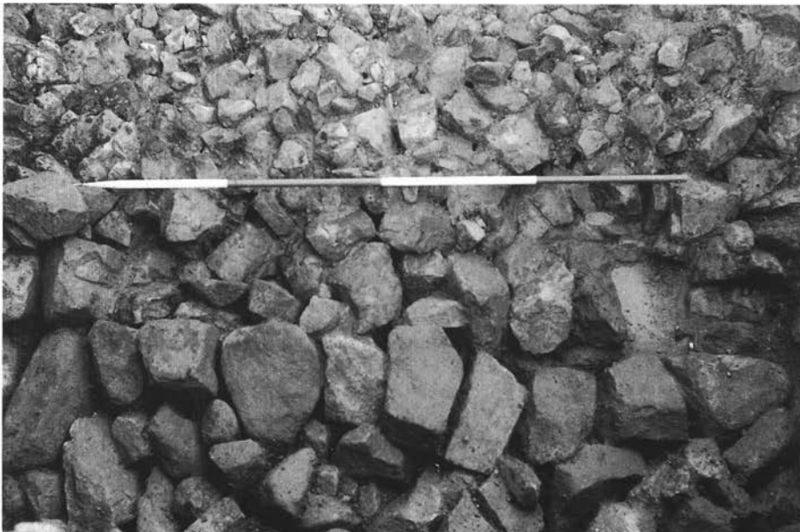
Plate 5: Detail of surviving wall footing in section C-D, showing gang-junction in construction on corner.
