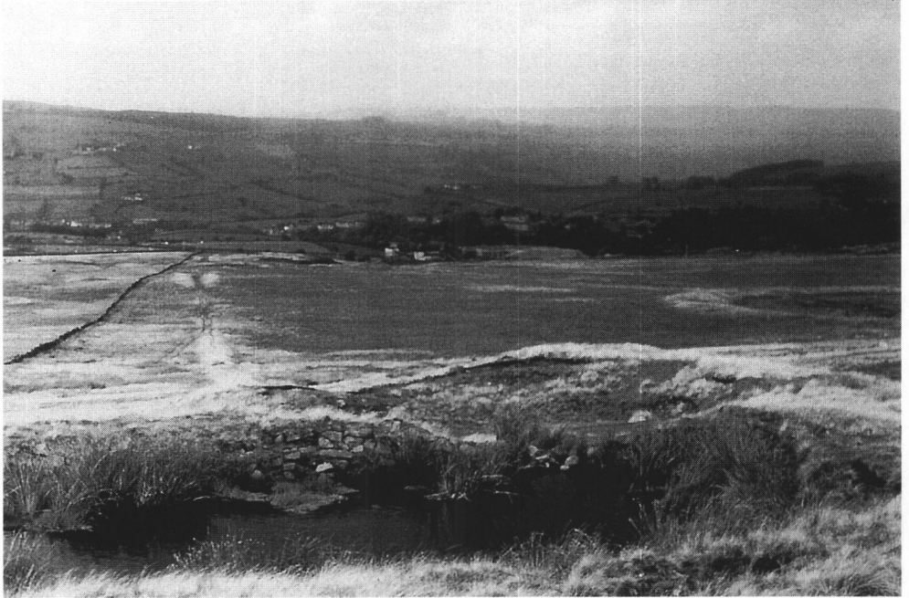
Plate 5: Reservoir (for steam engine) and beyond it the shaft for Burnt Edge Colliery on Ollersett Moor. Note the line of a tramroad leading down the slope. On the right, the circular depression is the filled-in reservoir built on the site of a spring for the Ollersett Waterworks in 1831. (SK 033852).
