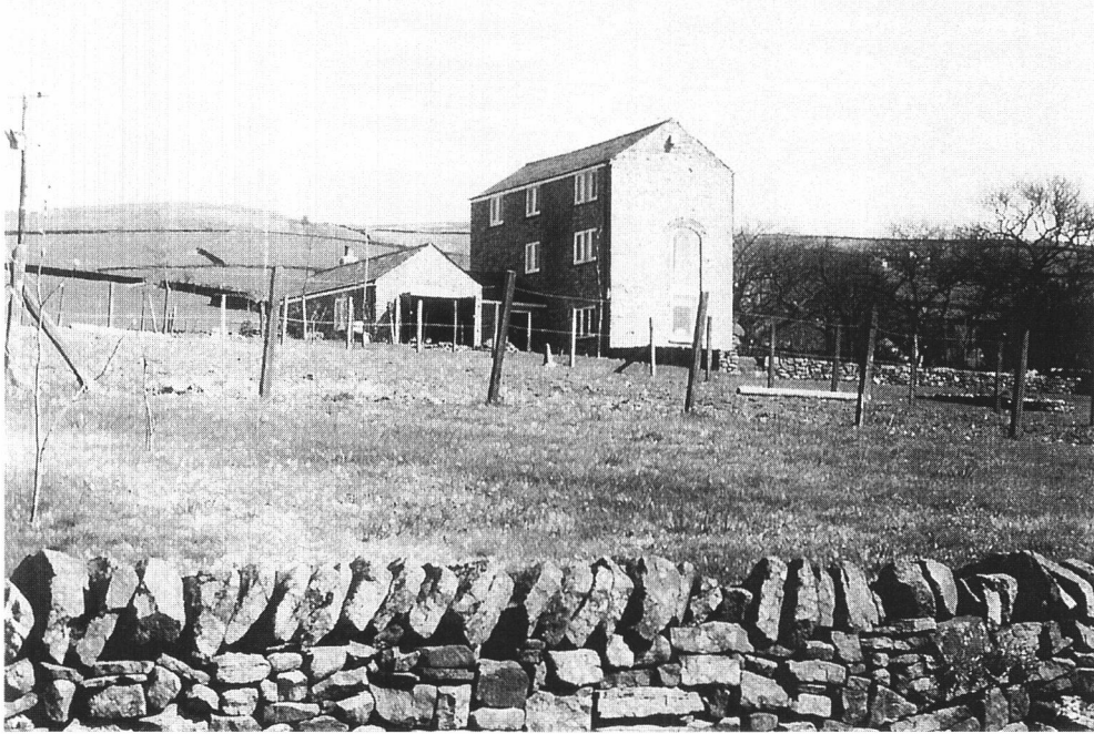
Plate 4: Converted engine house on Dolly Lane. Dolly was the name of the pit. (SK 022831).
