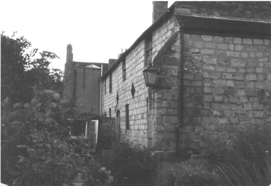
Plate 6: Rear of 7-9 Abbey Lane after renovation, 1983 (J. Steer).
