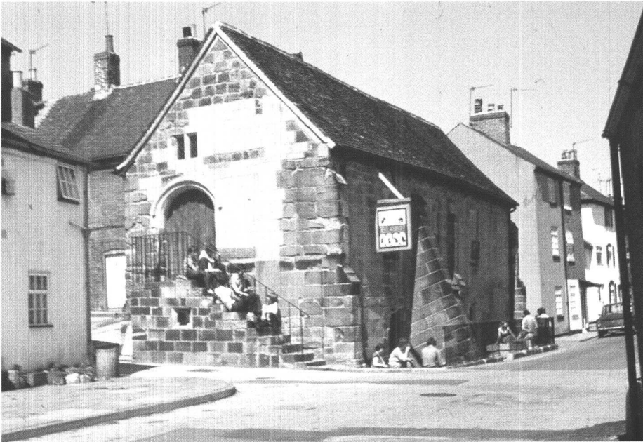
Plate 20: Abbey pub after restoration, 1979 (R. Dallas). Much of the south wall was removed during the renovation works. The hoodmould has been replaced and appears to have a deeper curve than that shown in 1869.
