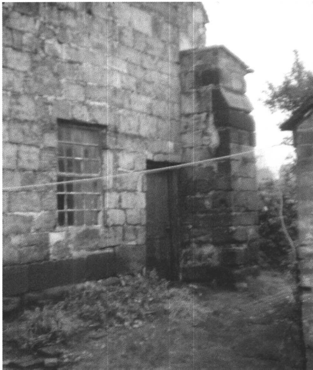
Plate 8: Buttress at rear of 9 Abbey Lane, before renovation, 1971 (R. Dallas).
