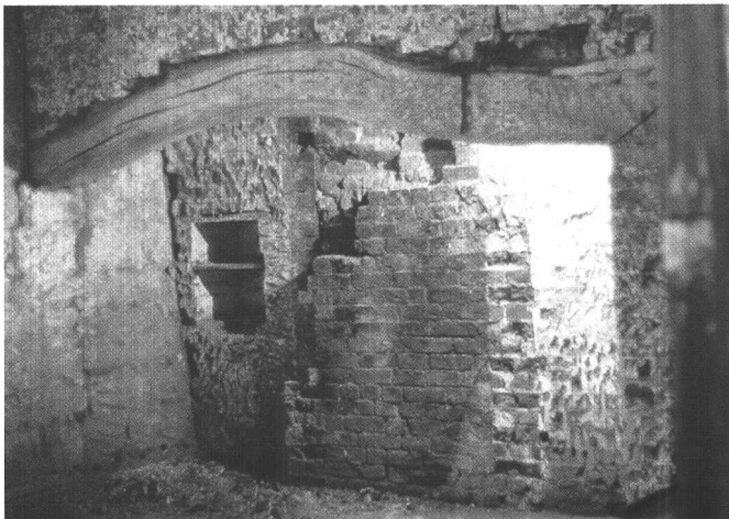
Plate 13: Dining room ceiling during renovation, 1971–72 (R. Dallas).
