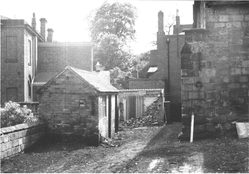
Plate 9: North wall of 9 Abbey Lane and workshop, during renovation, 1971 (R. Dallas). Note plinth forming base of the buttress.
