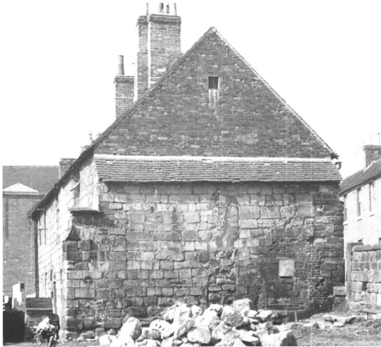
Plate 11: 9 Abbey Lane. north wall before renovation, 1971–72 (R. Dallas). Note the bricked up doorway and outline of the cutback ends of 3 former walls (2 outer, 1 internal). The cut down buttress supporting this wall which adjoins no 9 still has its small tiled cover.
