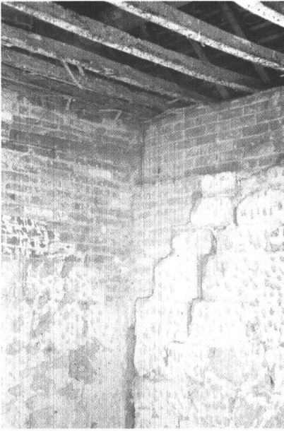
Plate 12: 9 Abbey Lane First floor during renovation. Internal and west walls. Note different sizes of bricks indicating two building phases, 1971–72 (R. Dallas).
