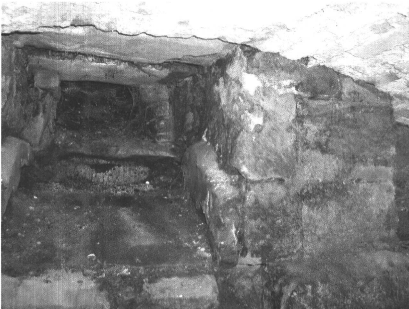
Plate 15: 7a Abbey Lane (Darley Abbey Stores). Ground Floor, north room, west wall with coal shute, 2007 (P. J. Steer).
