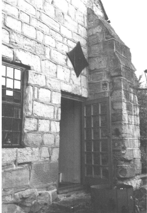
Plate 9: North wall of 9 Abbey Lane and workshop, during renovation, 1971 (R. Dallas). Note plinth forming base of the buttress.
