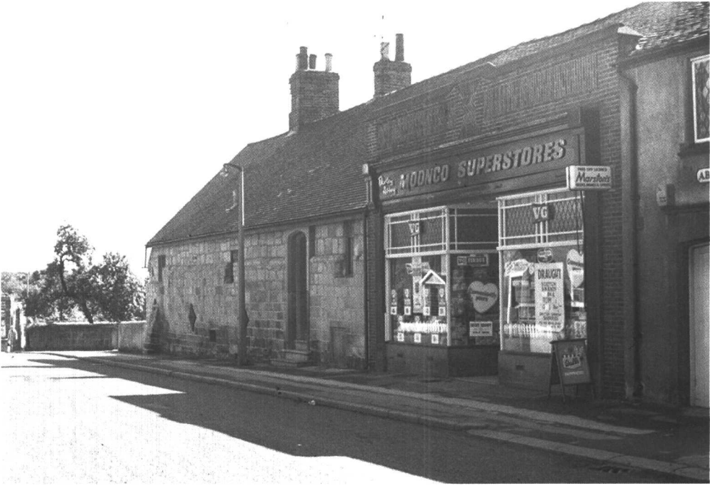
Plate 2: 7a (Moonco), 7 and 9 Abbey Lane after renovation of exterior of nos 7 and 9, 1972 (R. Dallas). Note the 19th-century entrance to no 7 which leads into the first floor and the grille to its right. The west wall shows the cladding wall and the raised line of the original wall.
