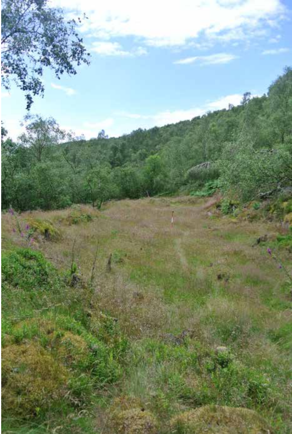
Plate 5: Site 2 silted dam (looking east).
