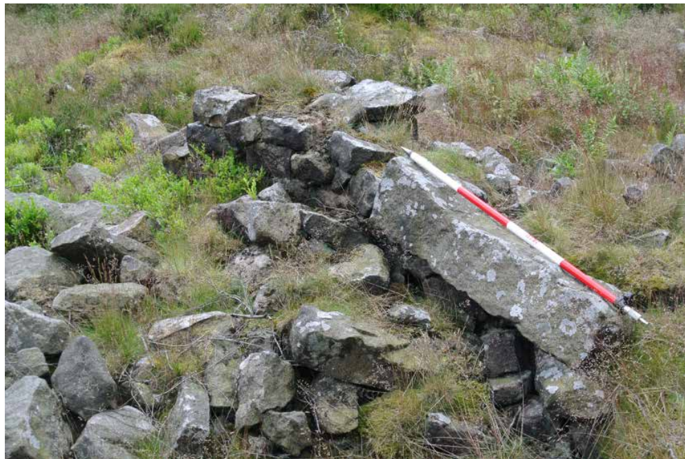
Plate 10: Lintel partly in situ .
