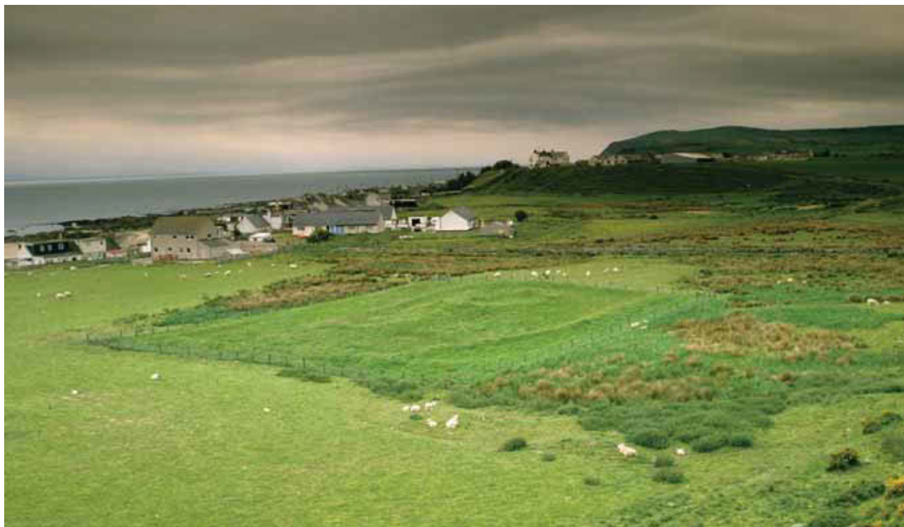
Illustration 1.4 View of the chapel site from the north-east
