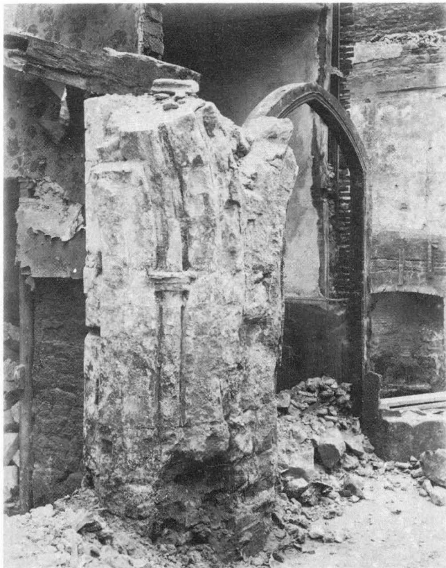
Plate XLIII. Two adjacent doorways possibly on the street frontage; as suggested by the position of the fireplace.
