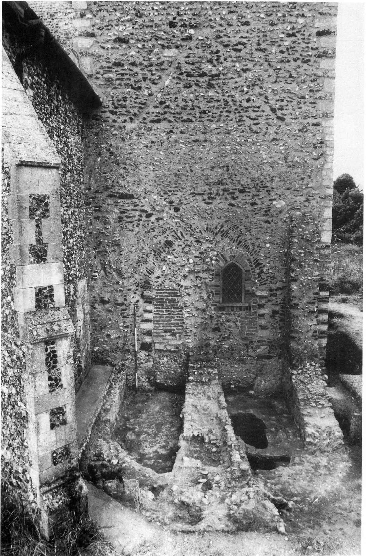
Plate XVII Guestwick: the excavation of the chancel and lower part of tower east face. Ref.CLP 20
