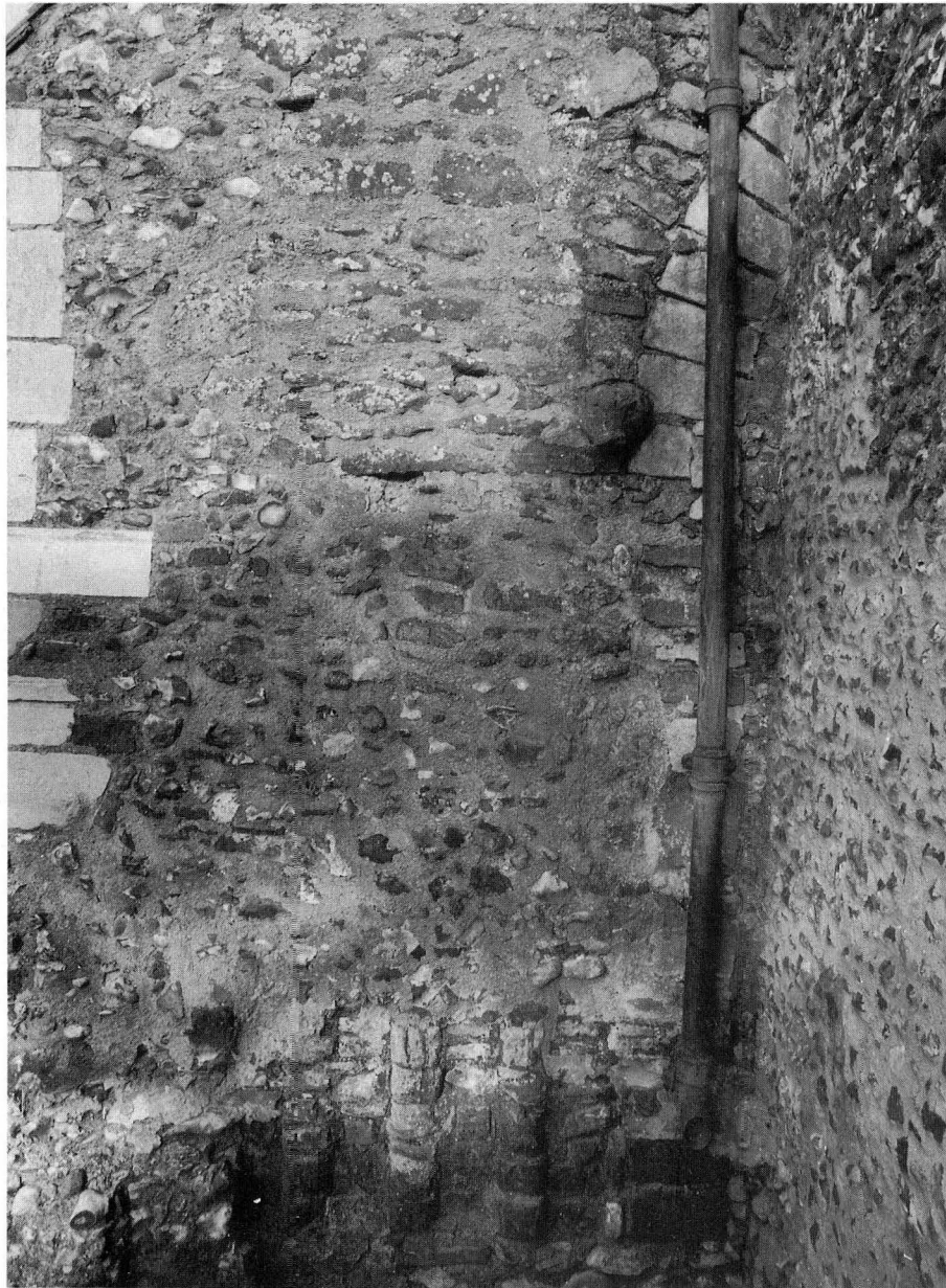
Plate XX. Guestwick: the lower part of the tower west face showing voussoirs of nave arch and recessed half-round mouldings. Ref.CLN 27
