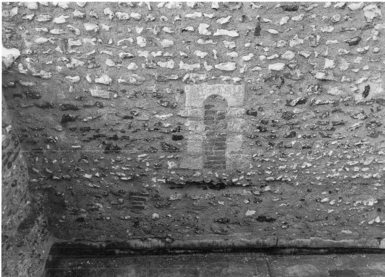
Plate XXII Guestwick: south face of tower showing blocked window above horizontal recess. Ref.CLN 10
